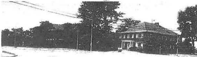
The buildings are now connected to the Ford Club with additional offices. *
