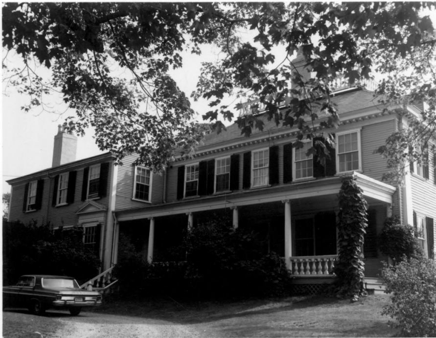
Vassall-Craigie-Longfellow House, 1759 West (side) elevation; rear service wing at left, and part of south (front) elevation at right
