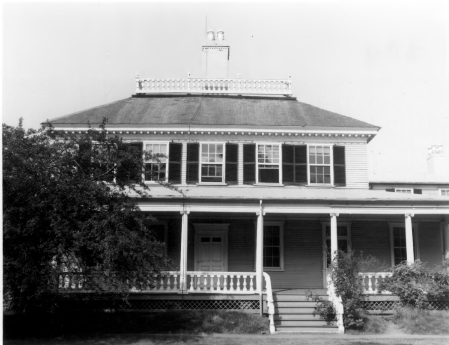
Vassall-Craigie-Longfellow House, 1759 East (side) elevation; rear service wing at right
