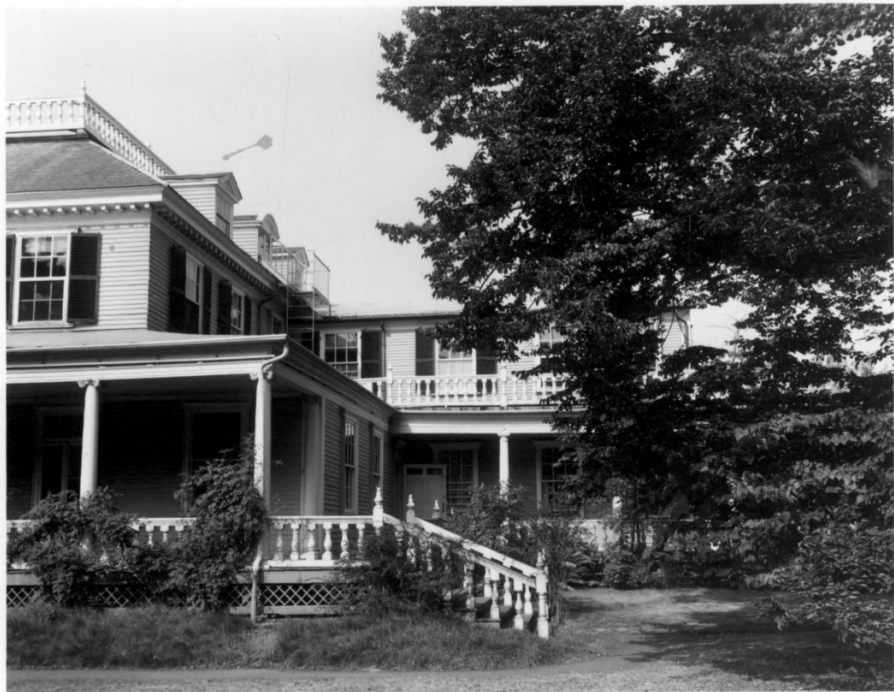
Vassall-Craigie-Longfellow House, 1759 Left--Part of east side; north (rear) elevation of main house, and (right) east side of rear service wing
