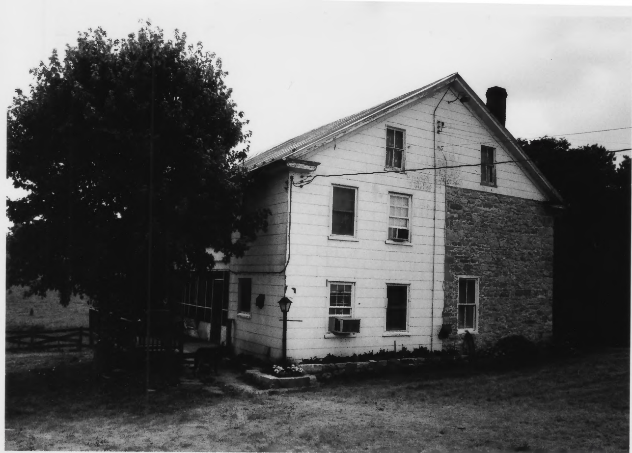
STRODE-MORRISON-TABLER HSE., Berkeley Co., WV
