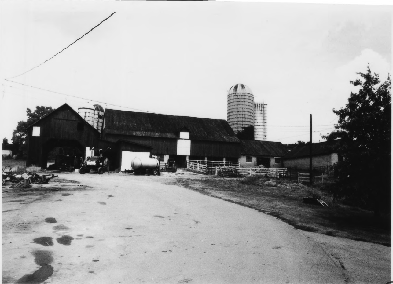
STRODE-MORRISON-TABLER HSE., BERKELEY CO., WV
