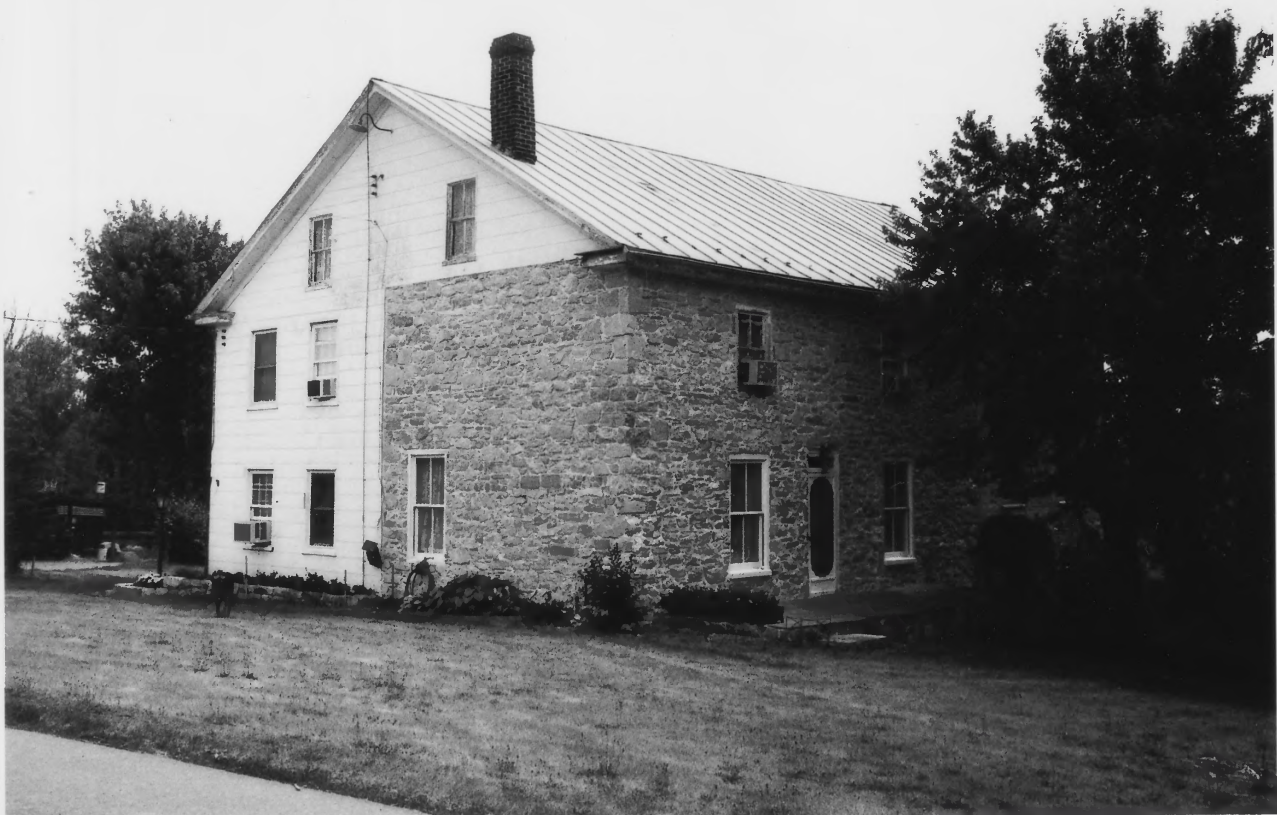
STRODE-MORRISON-TABLER HSE, Berkeley Co, WV
