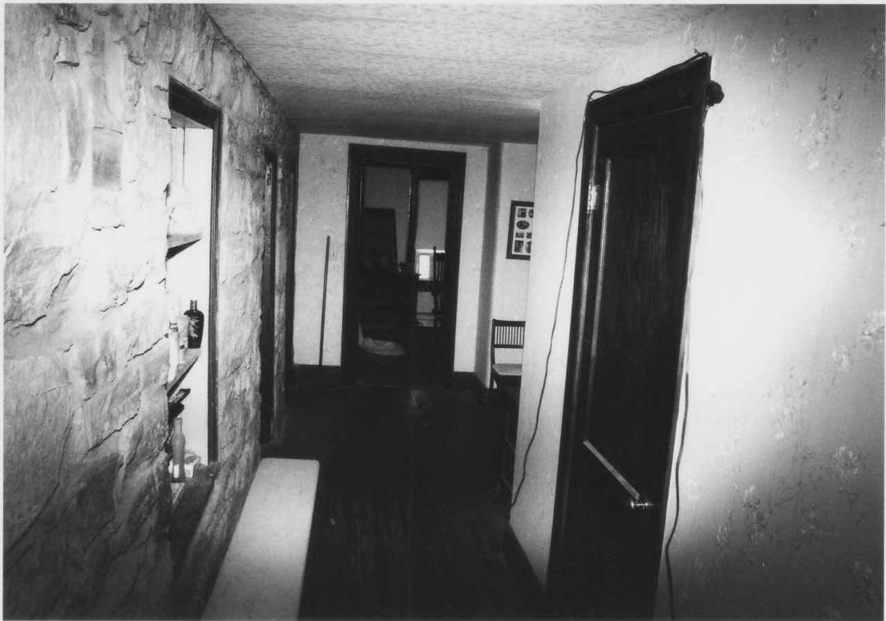
STRODE--MORRISON--TABLER HSE., Berkeley Co., WV
