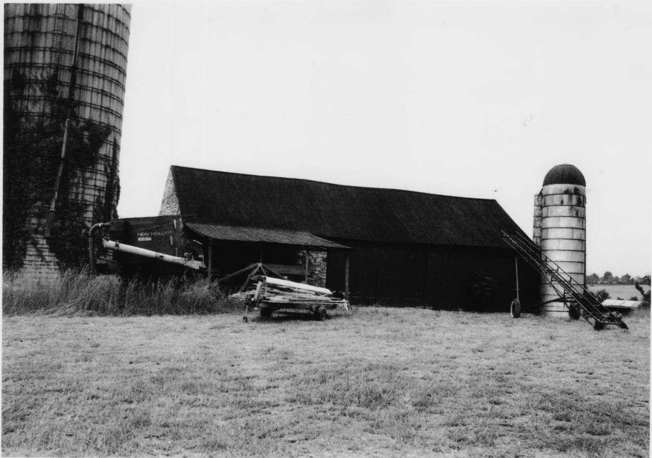
STRODE-MORRISON-TABLER HSE., Berkeley Co., WV
