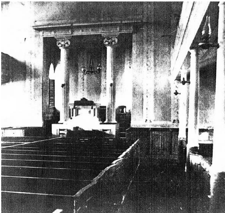
Figure 5: Historic (ca. 1875) interior photo of the Forks of the Brandywine Presbyterian Church, W. Brandywine Twp., Chester County. Built in 1761, remodeled in 1839 with recessed pulpit area identical to the Caernarvon Presbyterian Church in 1843. Forks of the Brandywine Church was demolished and replaced by a new Gothic Revival style church in 1875. (Chester County Historical Society)
