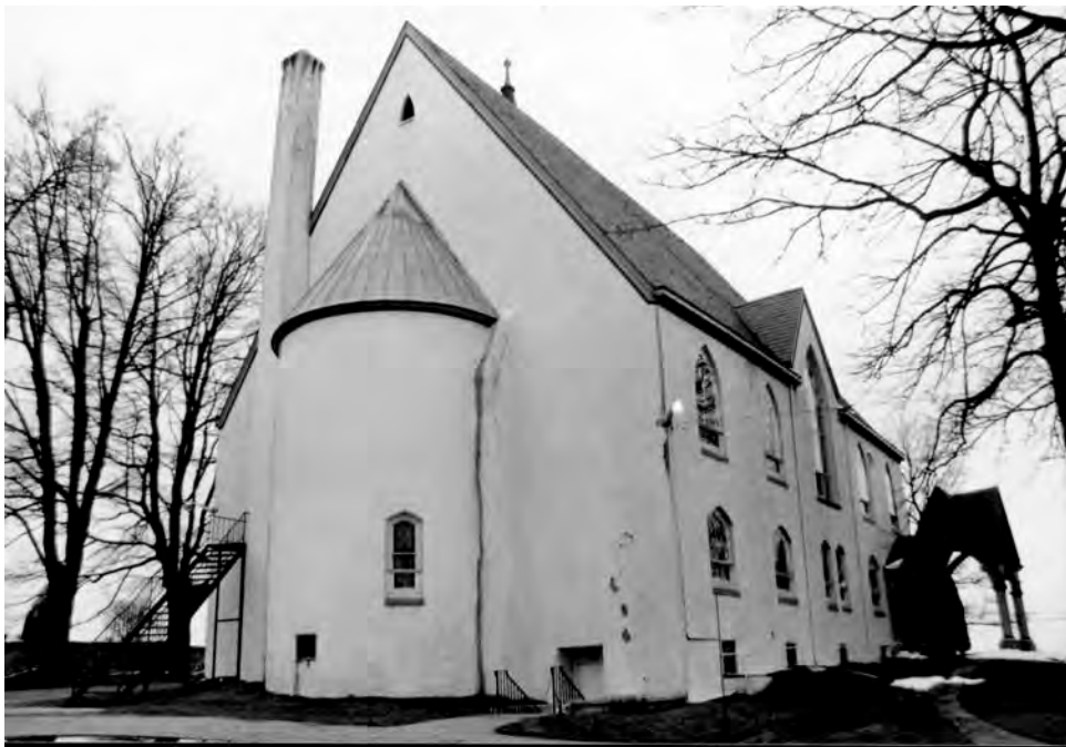
Figure 8: Forks of the Brandywine Presbyterian Church, West Brandywine Twp., Chester County, PA – built 1875 Rear elevation, highlighting continued use of rear apse (PA Historic Resource Survey File, Bureau for Historic Preservation – PHMC)
