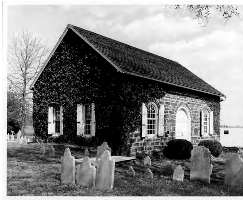
Figure 1: East Norriton Presbyterian Church, East Norriton Twp., Montgomery County, PA – NR Listed 1979 Built in 1698, the Church is an early colonial example of the Cottage Plan, typified by side entrance door. (National Register nomination form, files of the Bureau for Historic Preservation – PHMC)
