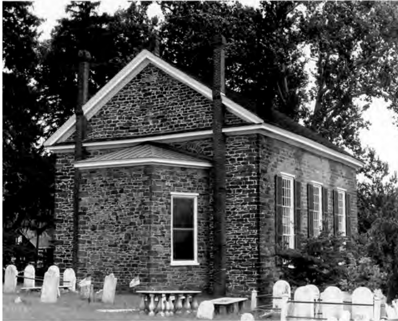
Figure 3: Newtown Presbyterian Church, Newtown Twp., Bucks County, PA – NR Listed 1987 Built in 1769. Rear view, highlighting apse addition constructed in 1842. (National Register nomination form, files of the Bureau for Historic Preservation - PHMC)
