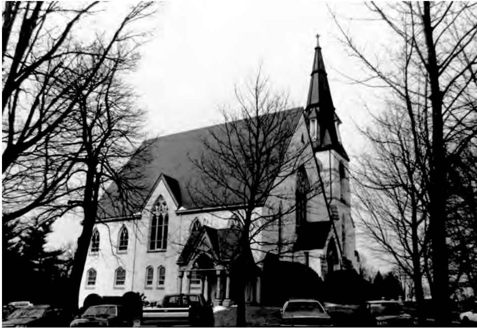
Figure 7: Forks of the Brandywine Presbyterian Church, West Brandywine Twp., Chester County, PA – built 1875 (PA Historic Resource Survey File, Bureau for Historic Preservation – PHMC)
