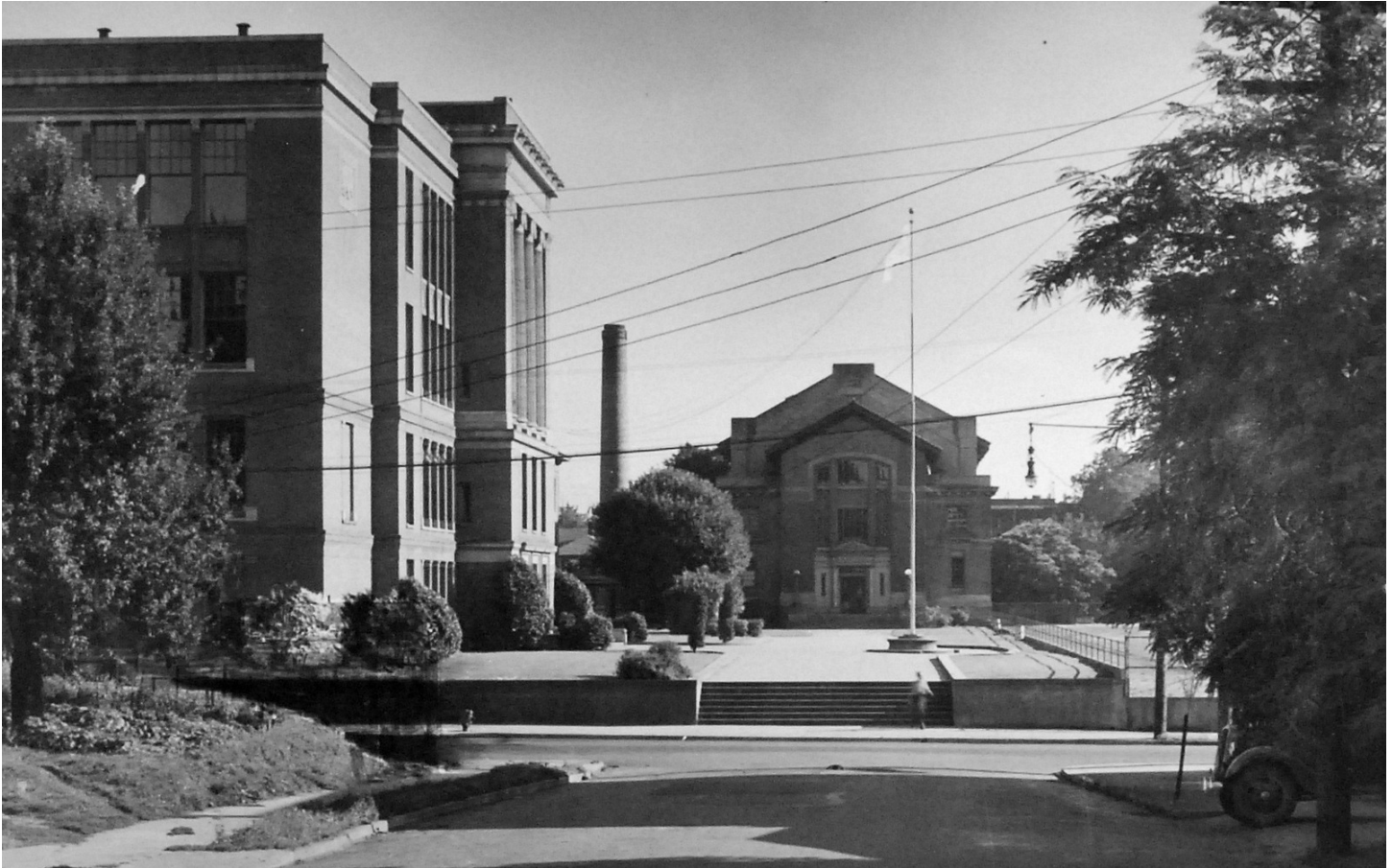
Figure 12: Historic photo showing Washington High School, boiler stack, and old gymnasium designed by Ellis Lawrence. Date of photo is unknown, but was taken after 1930 because the improvements to the athletic field have been made.
