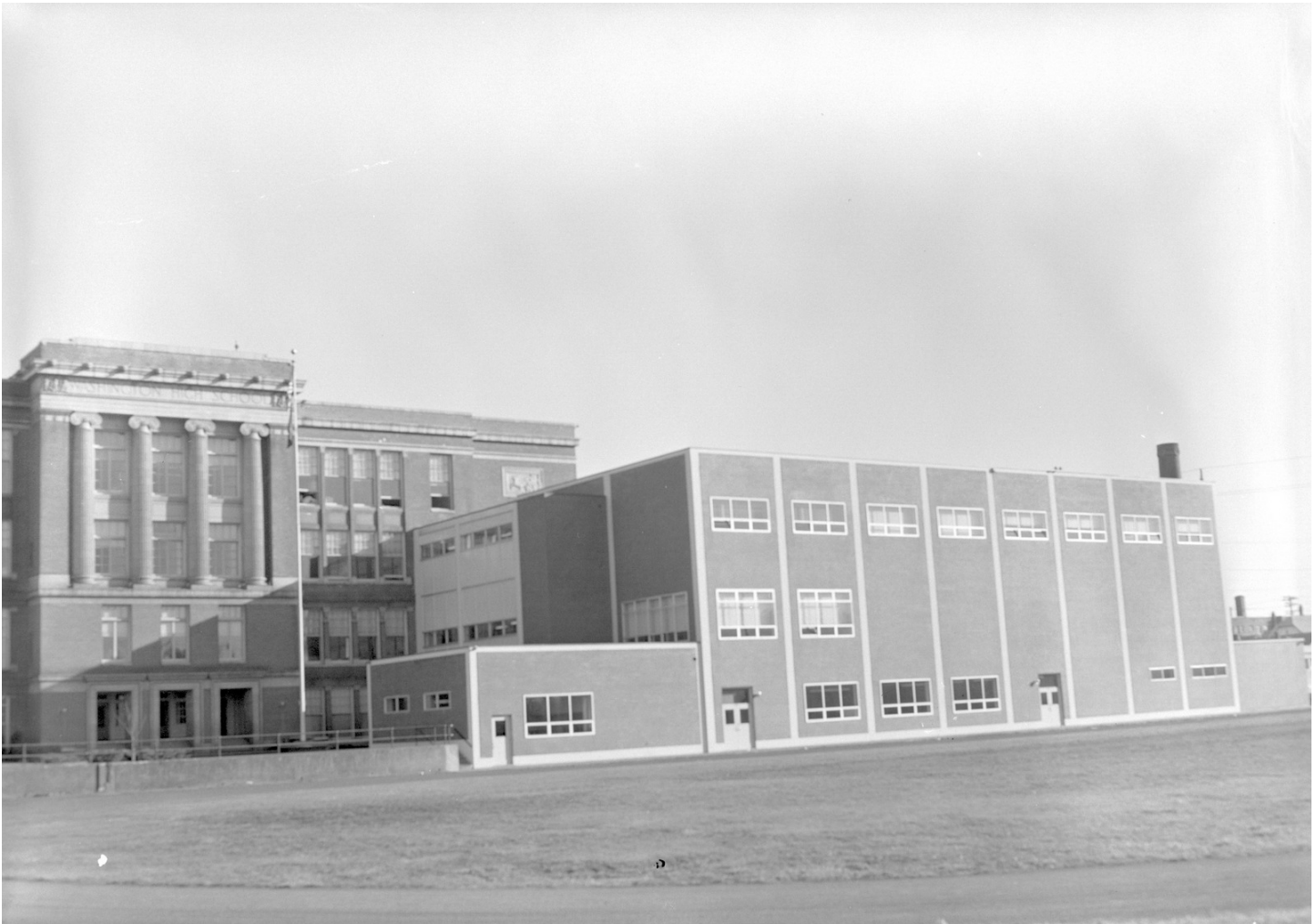
Figure 14: Historic photo c. 1960 showing the International Style "C Wing" addition at the building's west façade.
