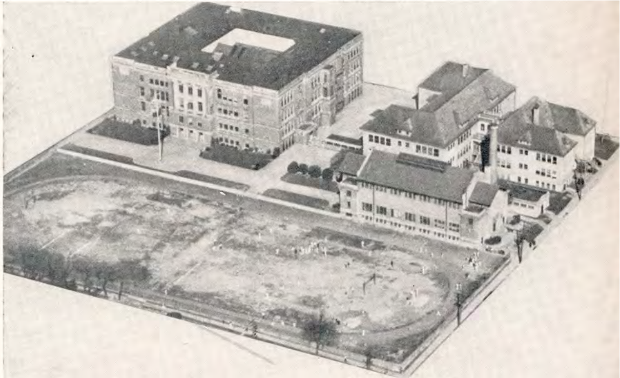
Figure 13: Historic campus aerial dating to 1939 showing the 1923 Washington High School, 1912 Boiler Building, 1910 Gymnasium, 1897 Hawthorne Grade School, and the athletic field.
