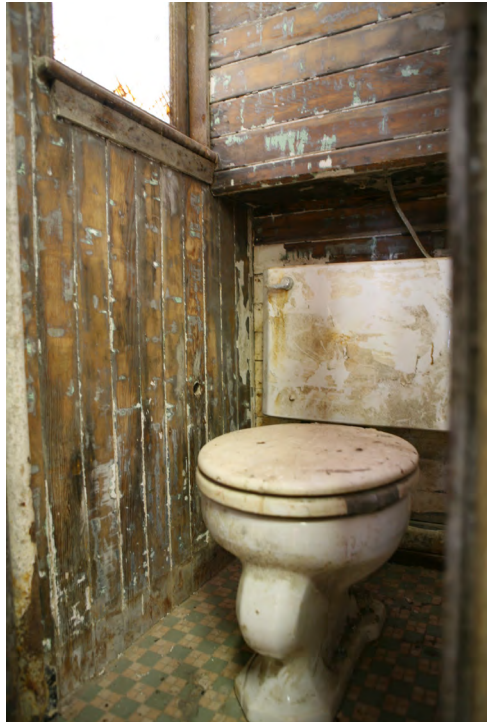
7 of 20. Western Flyer. Original head (restroom), at corner of deckhouse.
