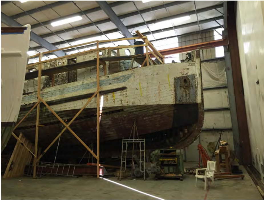
3 of 20. Western Flyer, at the Port Townsend Shipwright's Co-op, Port Townsend, WA. Looking from starboard to port across the bow (front). Photographer: Michael Sullivan, Artifacts Consulting, Inc., March 17, 2016.
