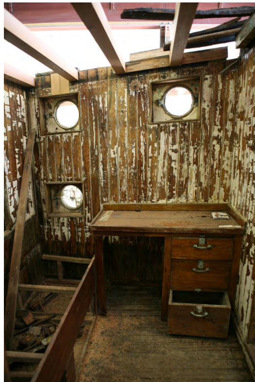
12 of 20. Western Flyer. Deckhouse, looking into captain's cabin from the corridor.
