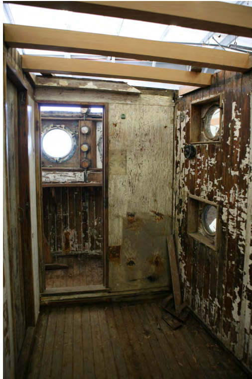
13 of 20. Western Flyer. Deckhouse, looking forward along corridor. Wheelhouse at far end, with the large port light visible.
