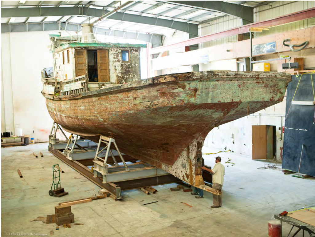
1 of 20. Western Flyer, at the Port Townsend Shipwright's Co-op, Port Townsend, WA. Looking forward and to starboard. Photo courtesy of Chris Chase, Port Townsend Shipwright's Co-op. Taken July 9, 2015.
