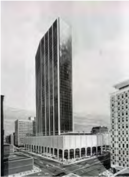
Figure 16 - First National Bank, Dallas; George L. Dahl and Thomas E. Stanley Joint Venture Architects Engineers. http://cityhallblog.dallasnews.com/2014/01/dallas-council-committee-to-vote-on-committing-50-million-in-tif-money-to-1401-elm-redo-with-strings.html/
