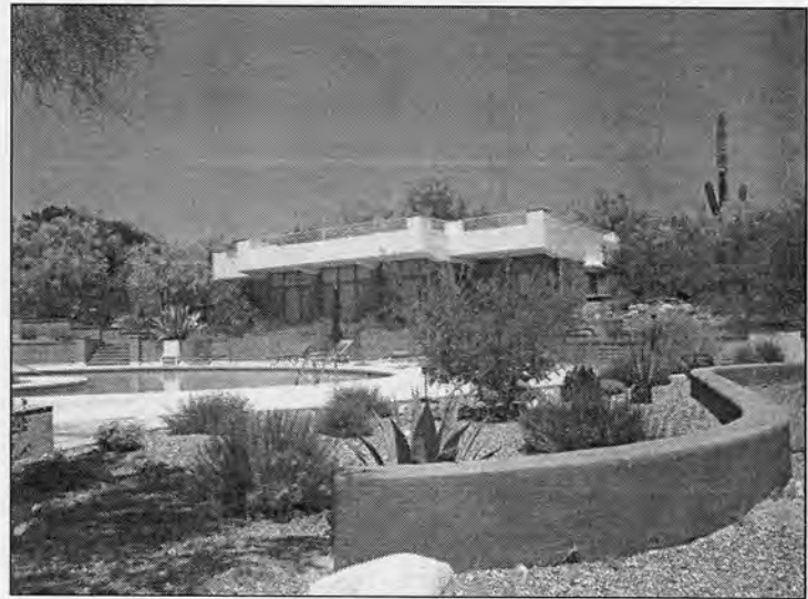
Photograph #6 Guest house west façade, camera facing northeast.
