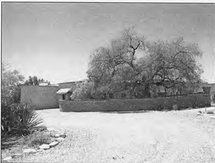
Photograph #3 East façade, camera facing southwest.
