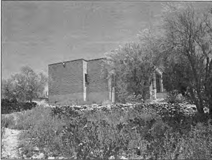
Photograph #5 West façade, camera facing northeast.
