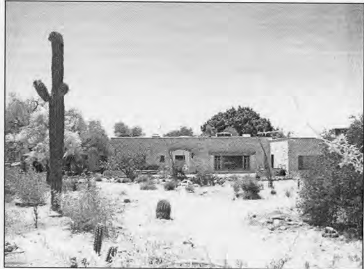
Photograph #2 North (front) façade, camera facing south.
