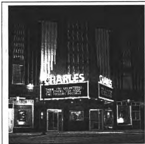
1934 Charles Theater – Exterior & Interior (Charles City Chamber of Commerce)
