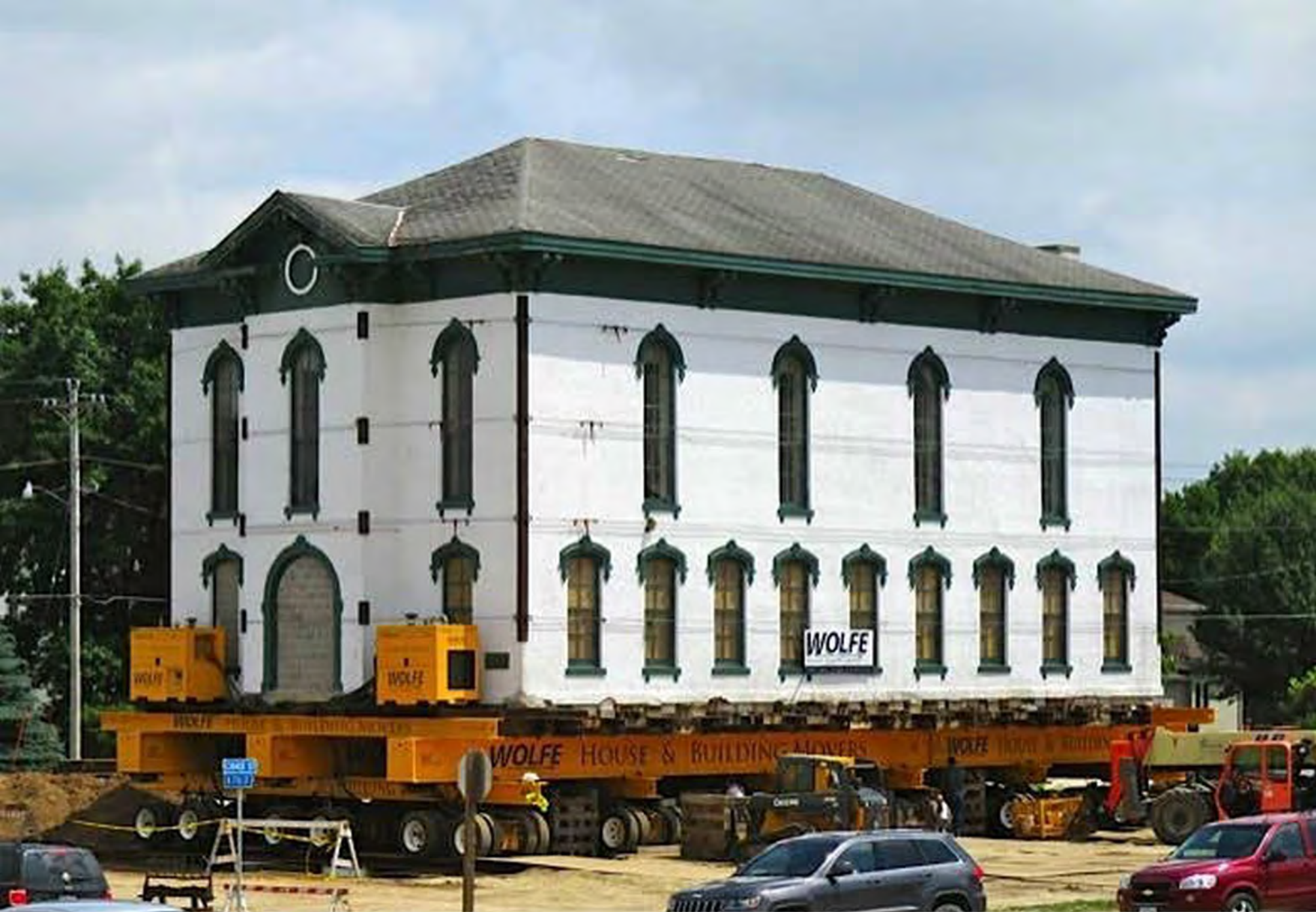
Cedar Valley Seminary Building, Osage IA, new building site, at NE corner of north 7th & Chase, at end of move on to cribbing.
