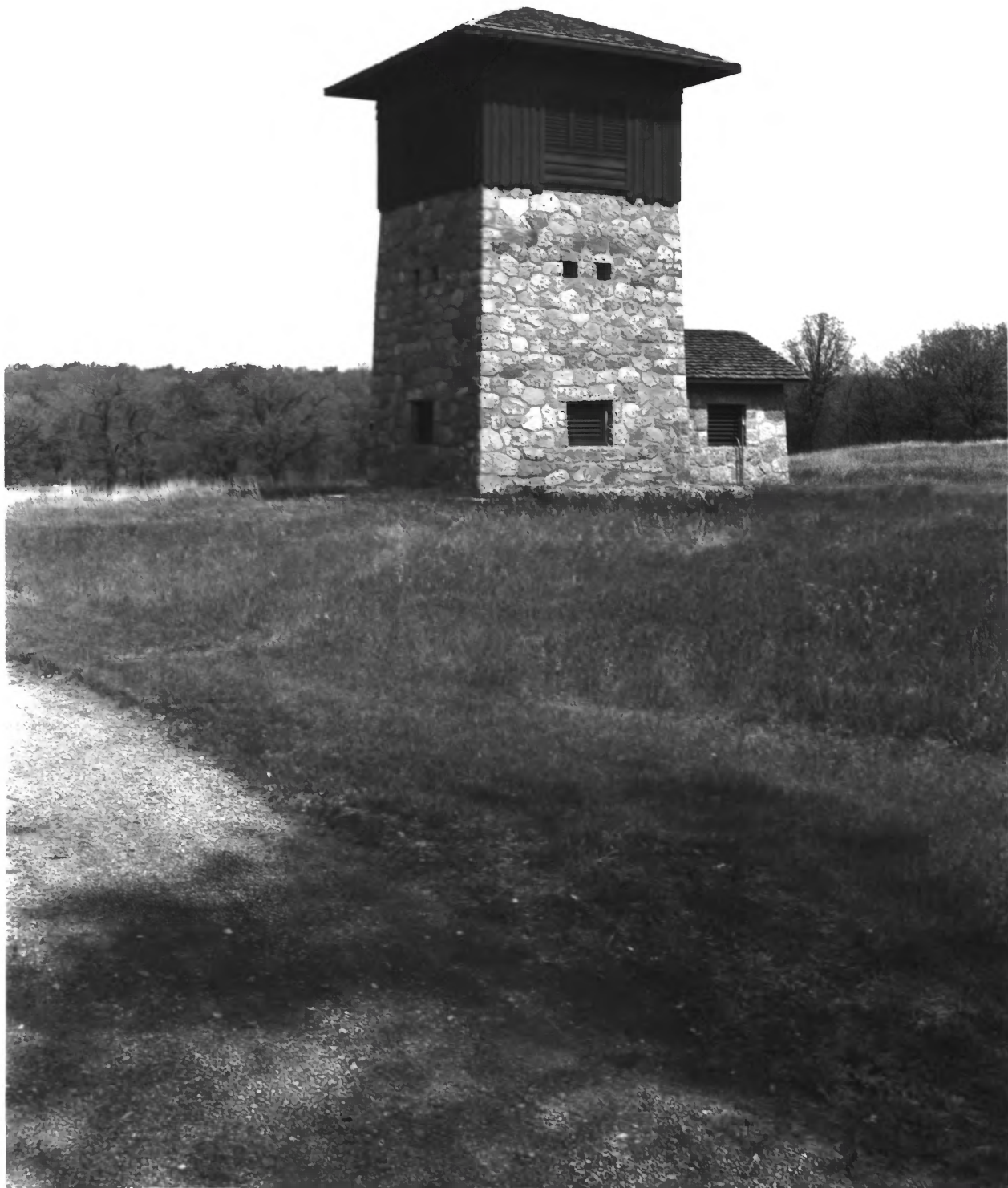
60 OLD MILL STATE PARK MARSHALL CO., MN STRUCTURE # 8 PHOTO I.D. 09782 # 13A
