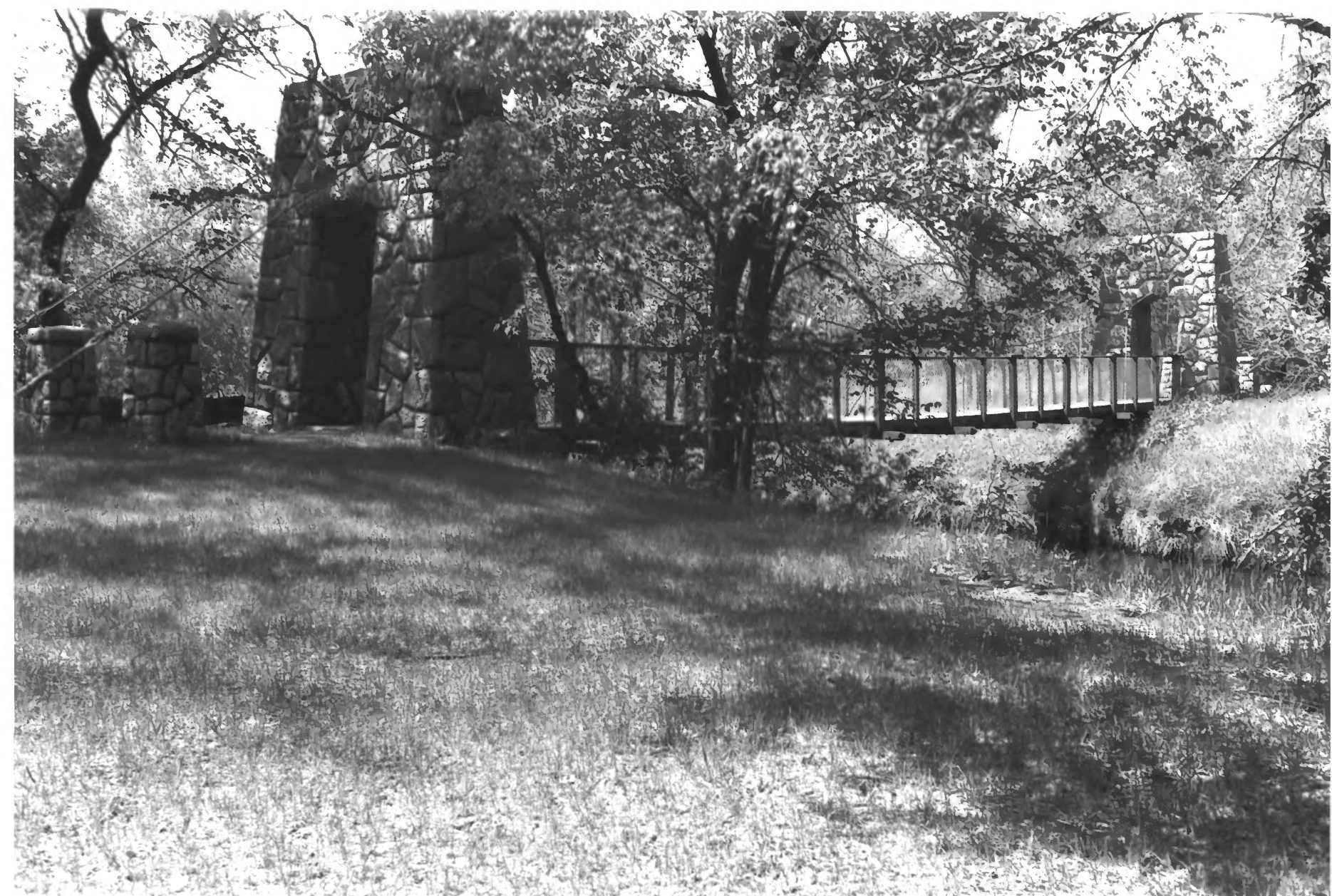
OLD MILL STATE PARK MARSHALL CO. MN STRUCTURE # 7 PHOTO I.D. 09782 # 21A
