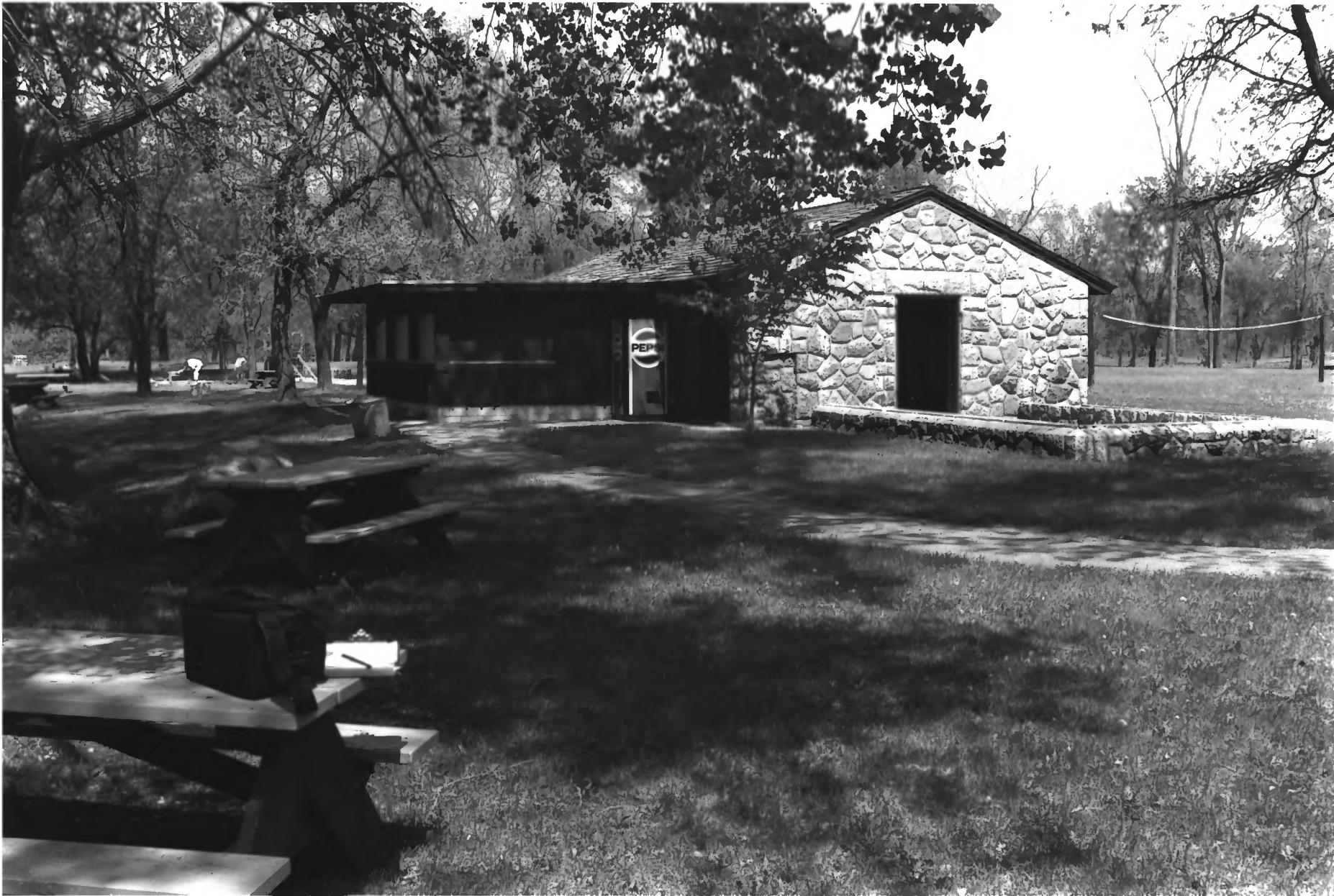
OLD MILL STATE PARK MARSHALL CO. MN BLDG # 3 PHOTO I.D. 09779 # 2
