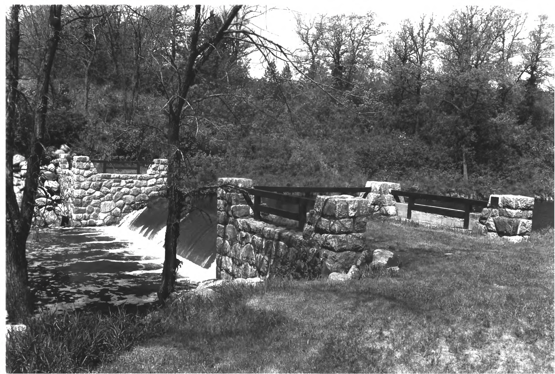
OLD MILL STATE PARK MARSHALL CO., MN STRUCTURE # 5 PHOTO I.D. 09779#1
