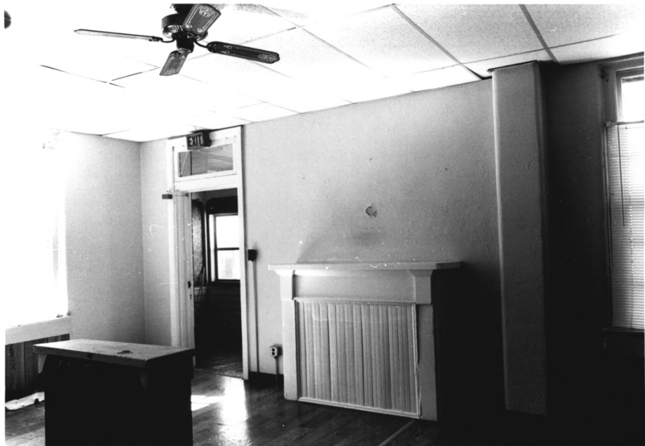
SULLIVAN COUNTY POOR HOME, SULLIVAN, SULLIVAN CO., IN
