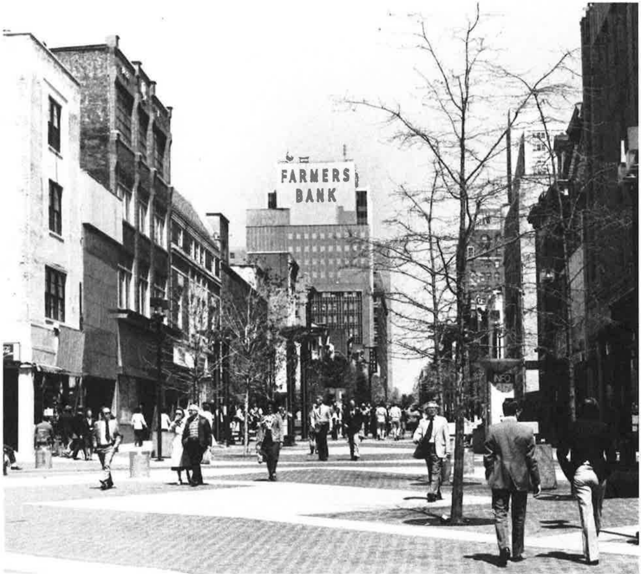
Fig. 21 – Market Street Mall, looking north from 6 th Street, c. 1980. (Historical Society of Delaware)
