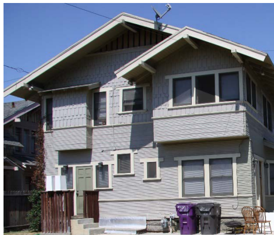
Figure 4, Photo 0002 West Elevation
