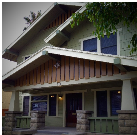
Figure 1, Photo 0014 Primary/East Elevation
