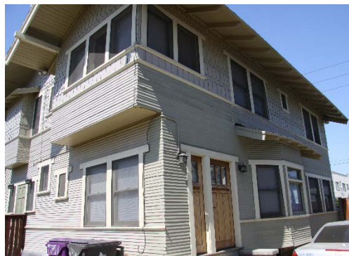
Figure 2, Photo 0003 South Elevation
