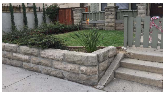
Figure 6. Photo 0010 Cast Stone Wall Detail
