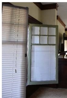
Figure 3, Photo 0021 North Elevation Casement Windows
