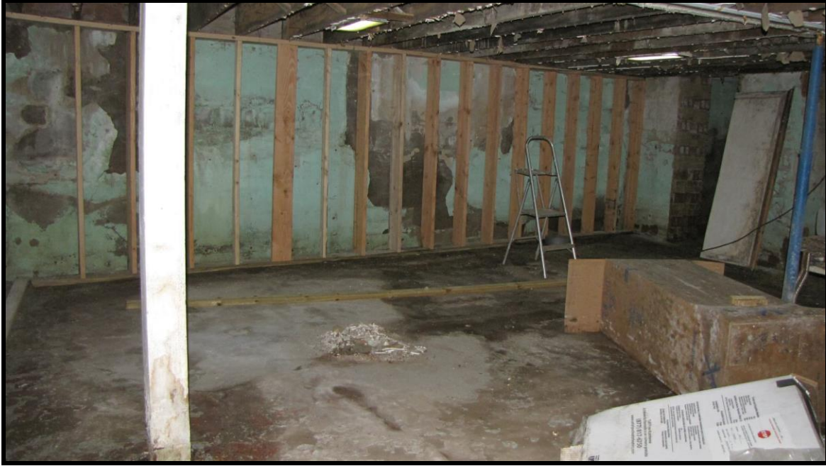
SD_Clark County_Raymond Bank_0013: Interior, basement, South wall, view to South West.
