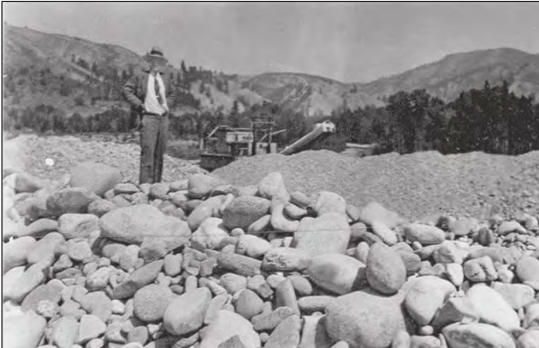
Figure 9. Dredge tailings at Featherville with the South Park Company's dredge in the background.
