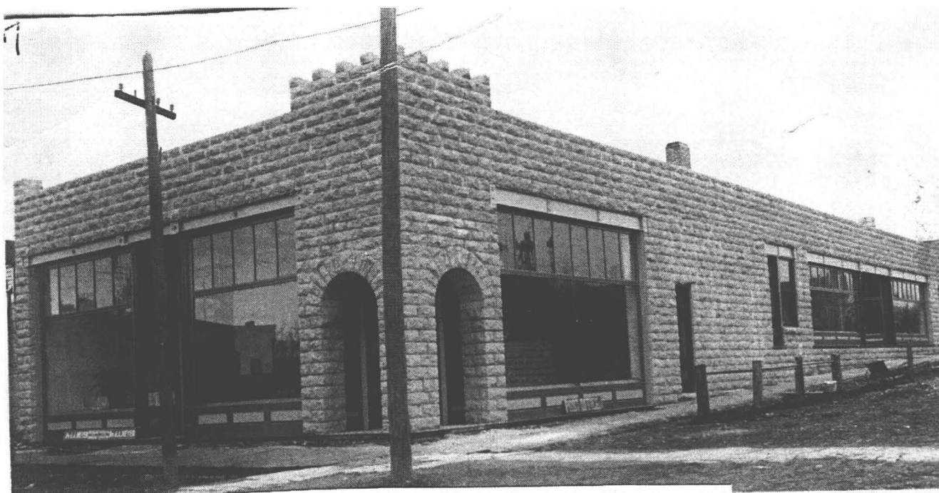
(Figure 5, View of Meyer Block, 227 Missouri, ca. 1906, from northeast.)
