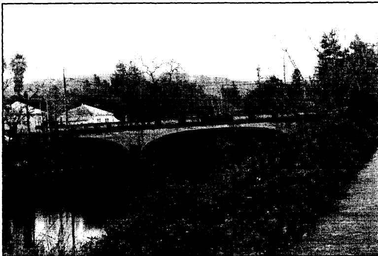
Photo No. 1 North elevation, from the northwest
