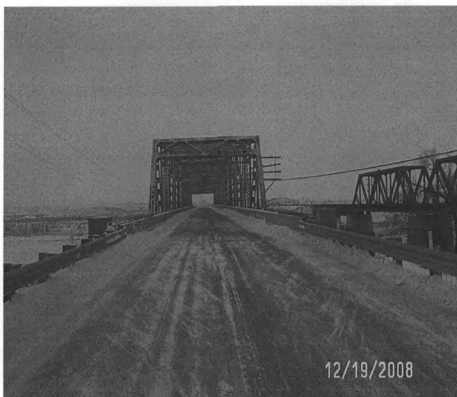
Photograph 0002. Powder River Bridge. East Portal. View to the west.
