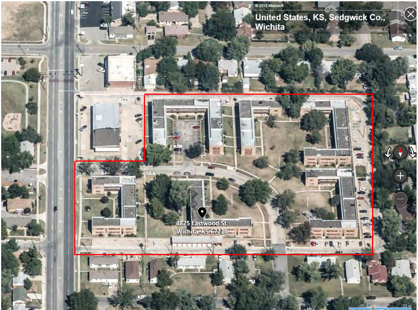
Figure 5 – Axonometric View of Site Eastwood Plaza Apartments 4802-4850 and 4825-4835 E. Eastwood and 616-626 S. Oliver Avenue Wichita, Sedgwick County, Kansas Lat/Long: 37.67576 -97.27950 Datum WGS84 Downloaded at Bing Maps 11 August 2018 © Microsoft Corporation 2018
