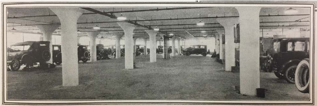
Figure 18 – Repair Shop, Fourth Floor ( Buick Bulletin , November 1925).
