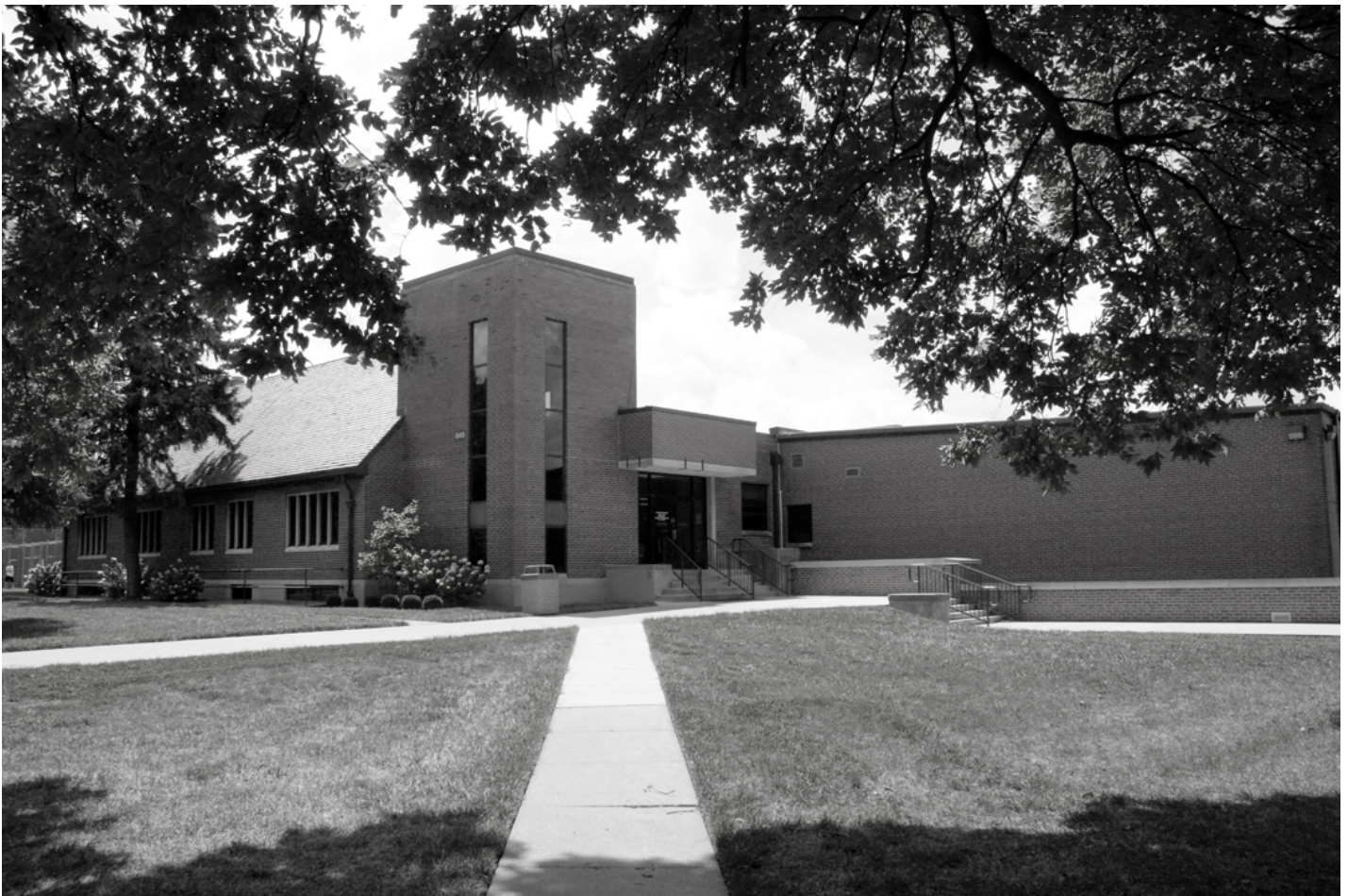
Photograph 13. Building 849, looking west, Field House/Gymnasium (non-contributing)
