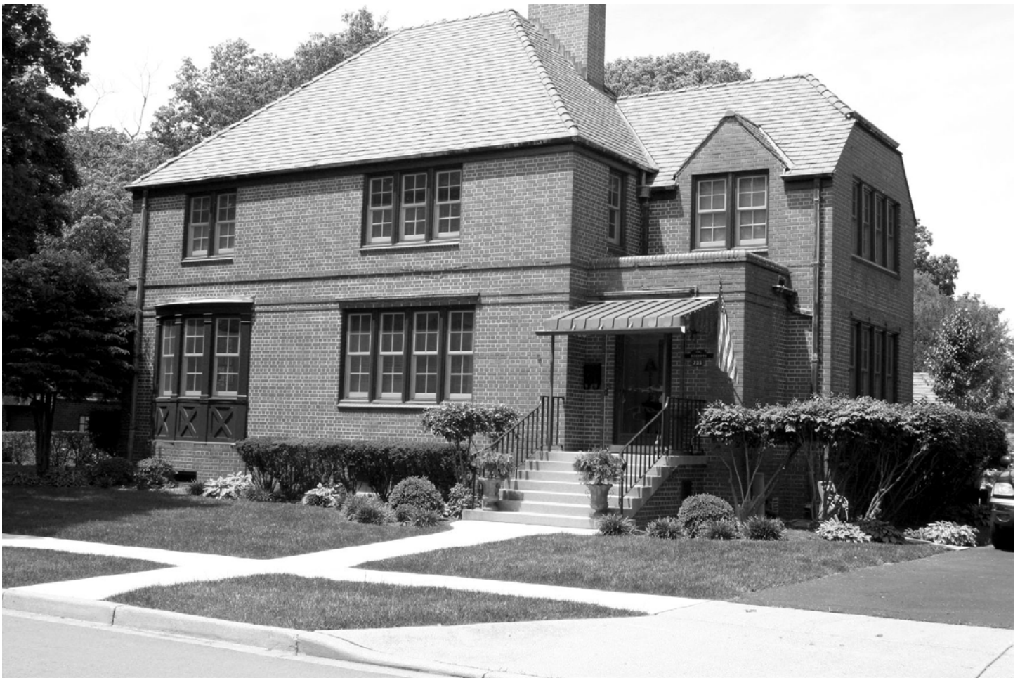
Photograph 7. Building 716 looking west, Type A
