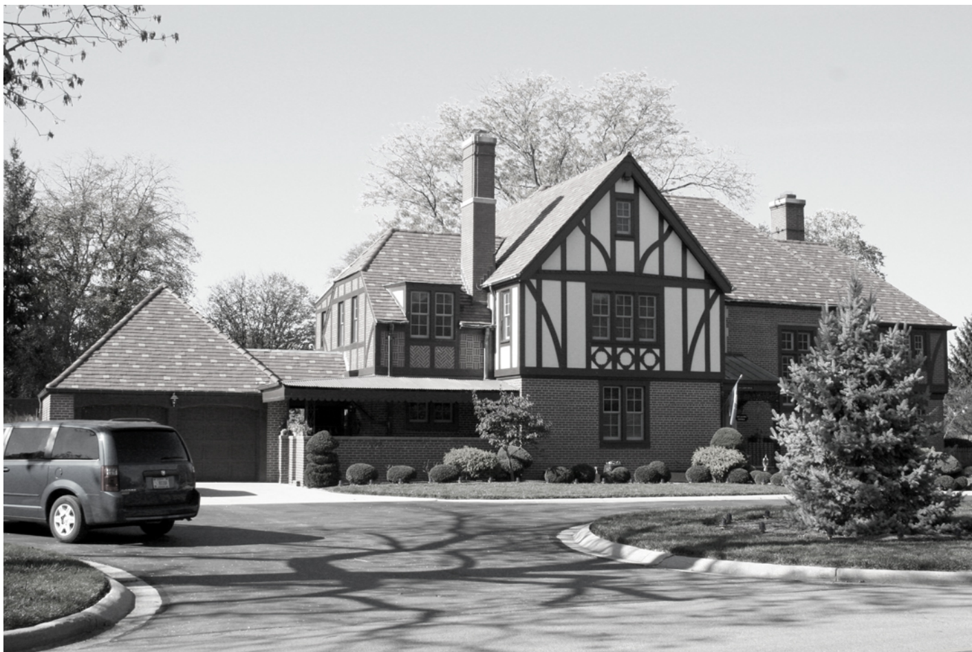
Photograph 10. Building 700, looking west, Commanding Officer's Quarters
