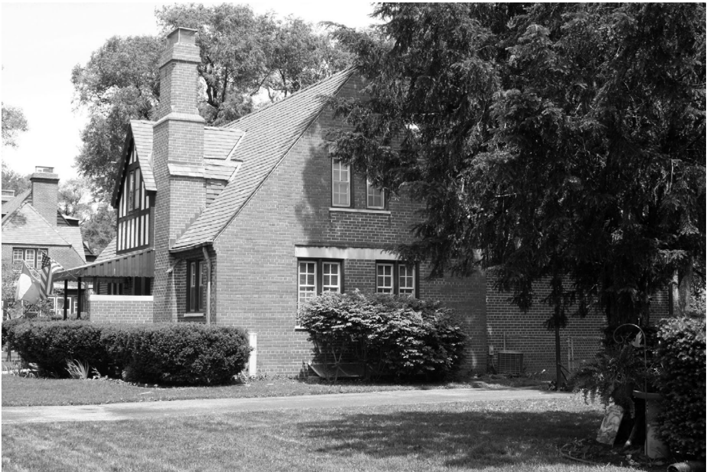
Photograph 8. Building 303 looking north, Type G
