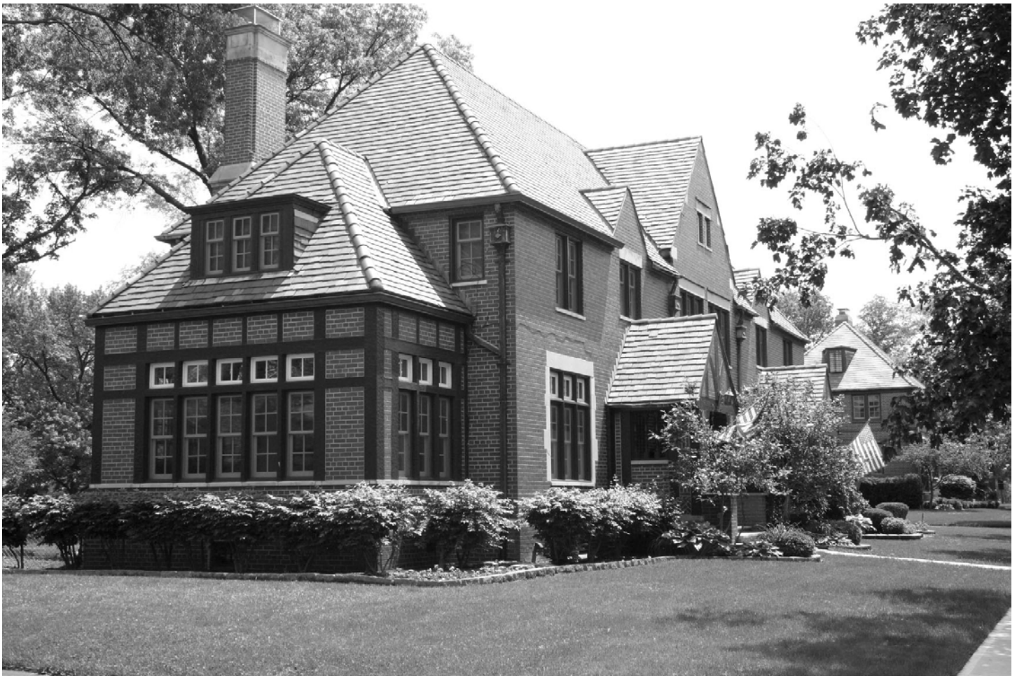
Photograph 6. Building 422 looking northeast, Type D
