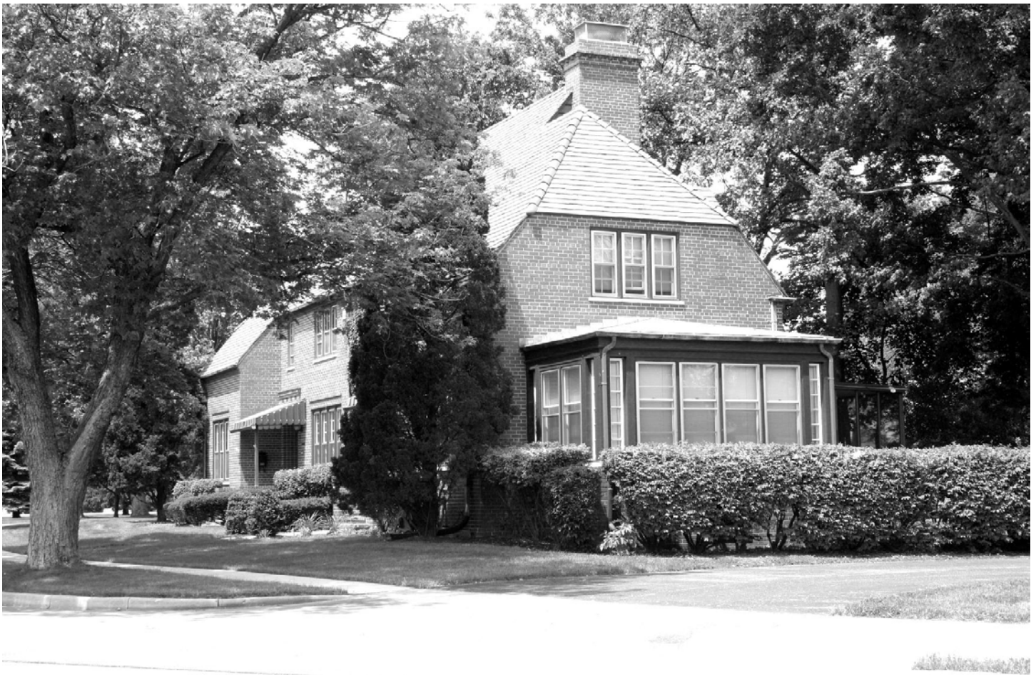
Photograph 4. Building 430 looking northwest, Type F.
