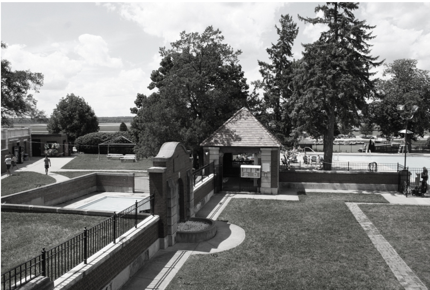
Photograph 12. Building 851 (non-contributing) and Brick Wall, looking west
