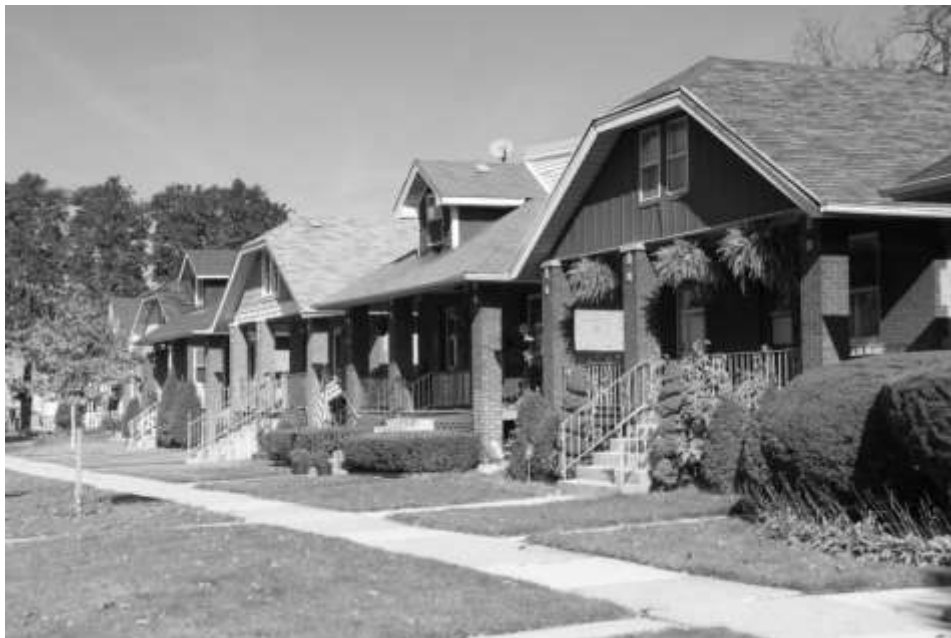
Figure 4 - View of typical Chicago bungalows with open porches. Source: Douglas Gilbert, AIA
