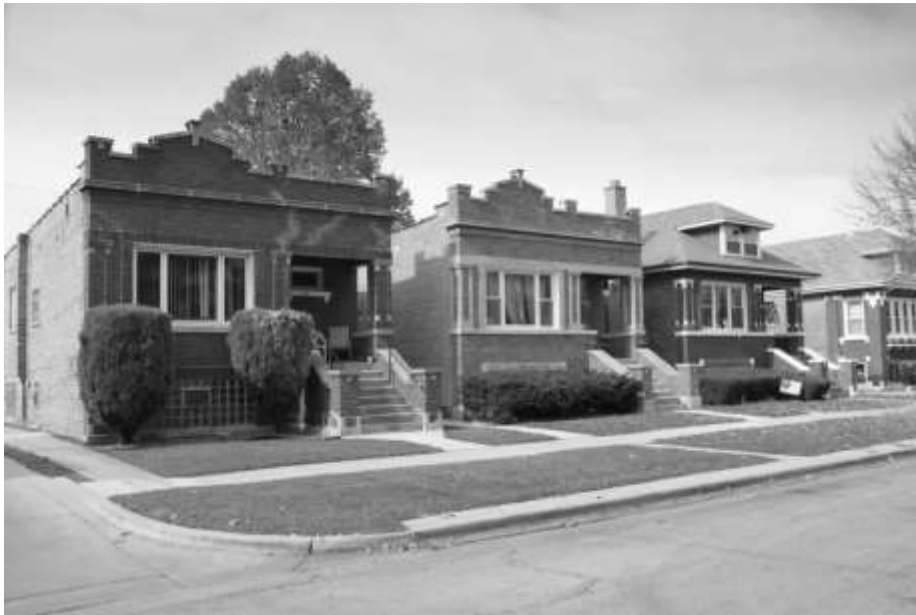
Figure 10 - Chicago bungalows with flat parapet fronts and with slight Romanesque Revival style details. Source: Douglas Gilbert, AIA
