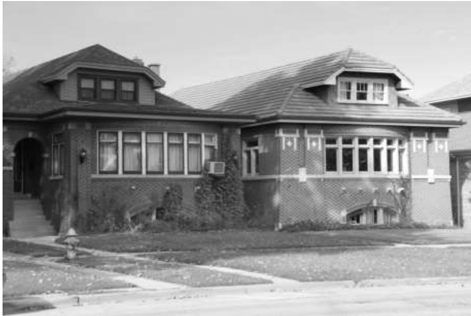
Figure 15 - Two Chicago bungalows that exhibit influence from the Prairie style. Source: Douglas Gilbert, AIA
