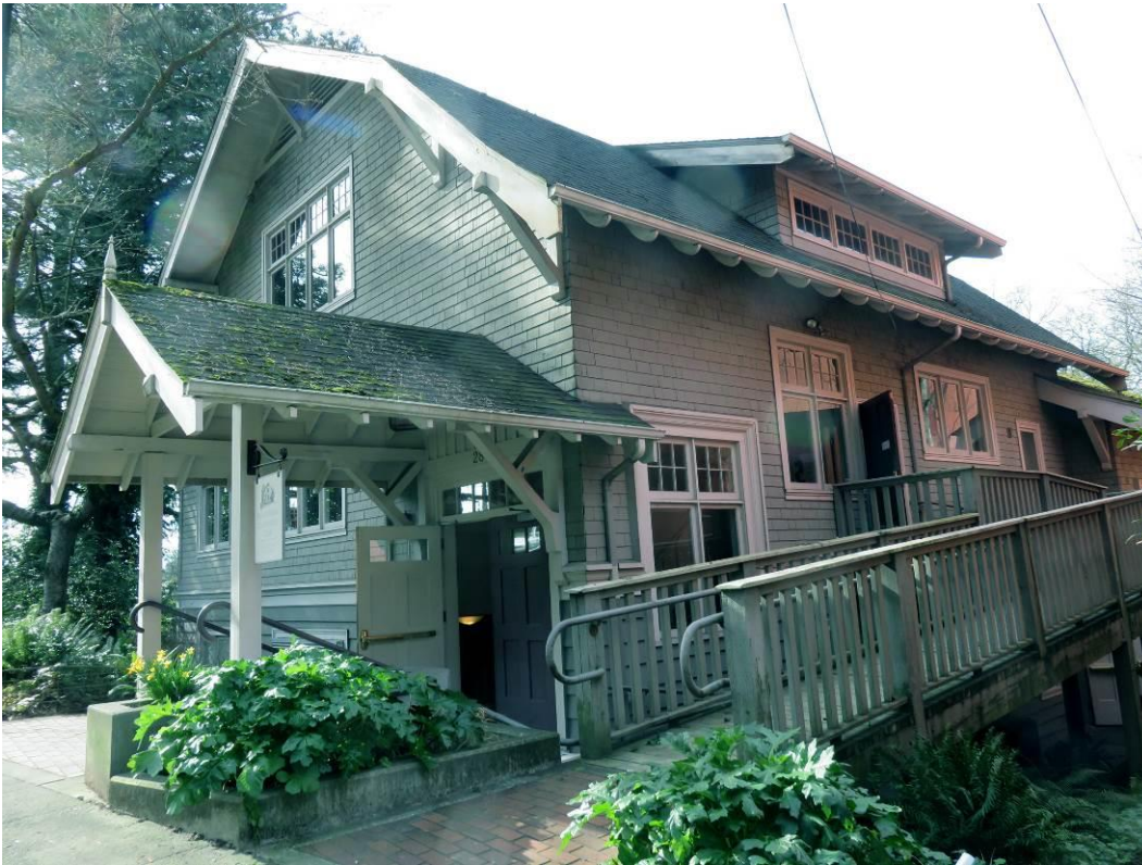
2 of 13 clubhouse exterior NE corner
