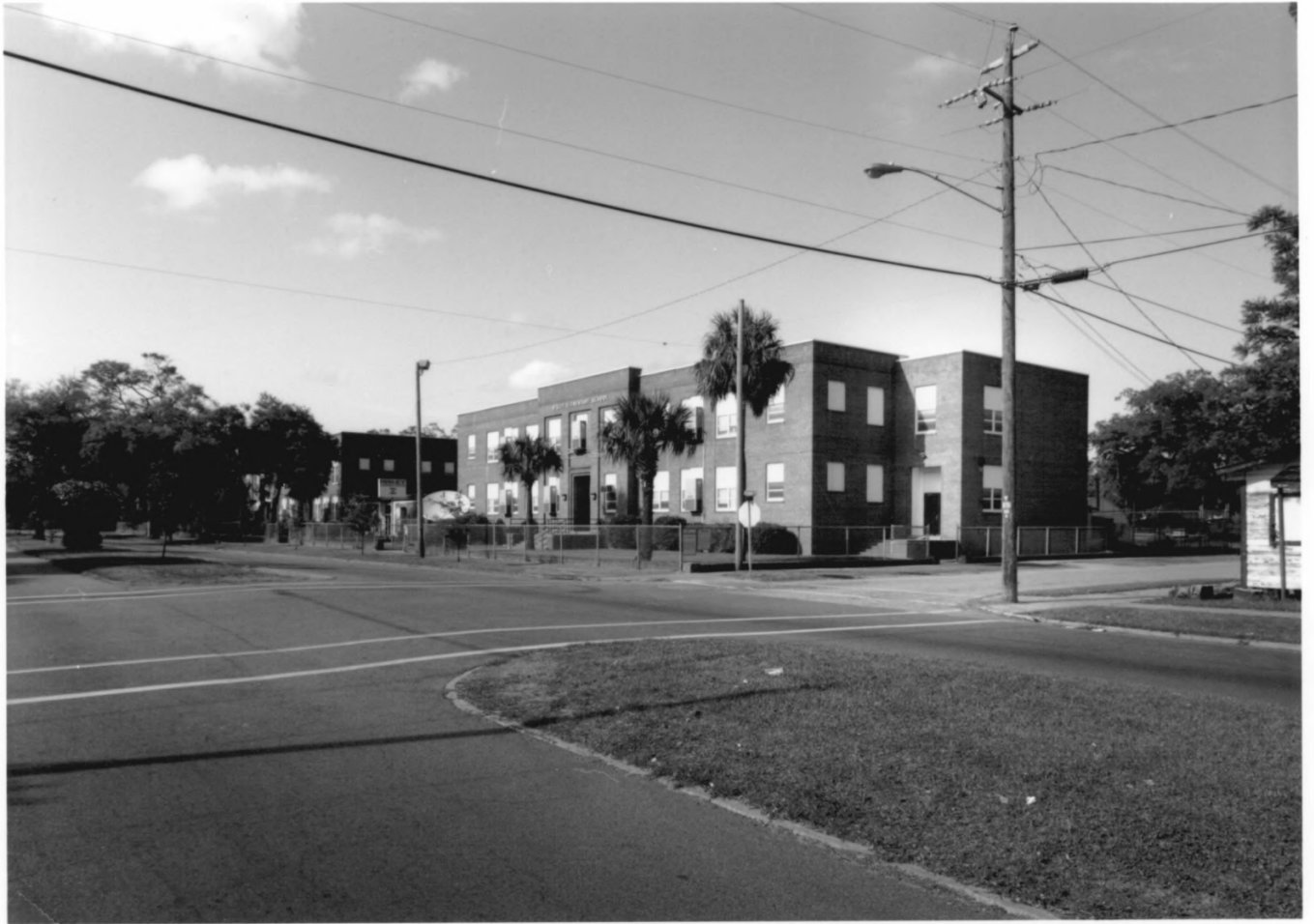
COLORED MEMORIAL SCHOOL/RISLEY HIGH SCHOOL BRUNSWICK, GLYNN COUNTY, GEORGIA PHOTOGRAPH 16 OF 18
