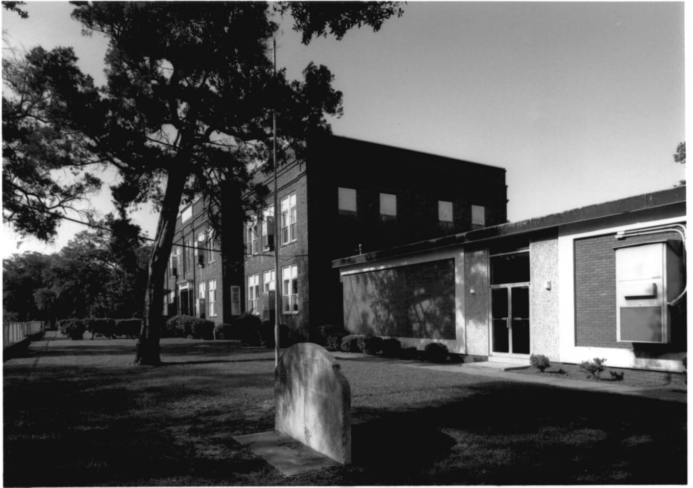
COLORED MEMORIAL SCHOOL/RISLEY HIGH SCHOOL BRUNSWICK, GLYNN COUNTY, GEORGIA PHOTOGRAPH 3 OF 18
