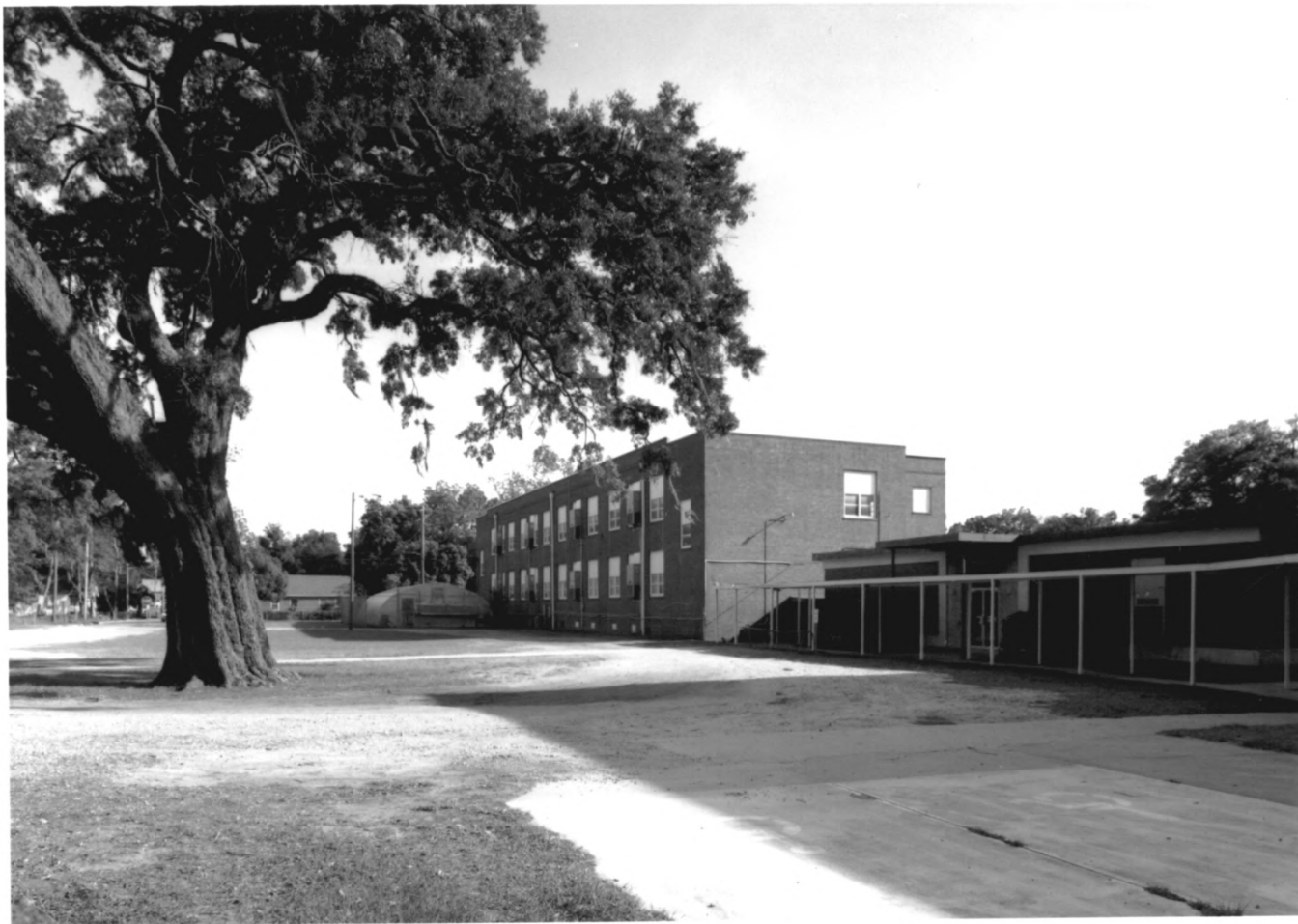
COLORED MEMORIAL SCHOOL/RISLEY HIGH SCHOOL BRUNSWICK, GLYNN COUNTY, GEORGIA PHOTOGRAPH 11 OF 18
