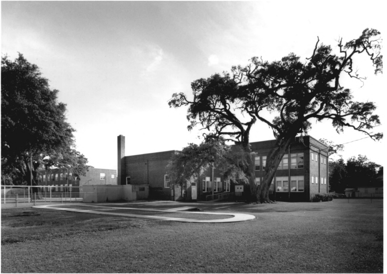
COLORED MEMORIAL SCHOOL/RISLEY HIGH SCHOOL BRUNSWICK, GLYNN COUNTY, GEORGIA PHOTOGRAPH 2 OF 18
