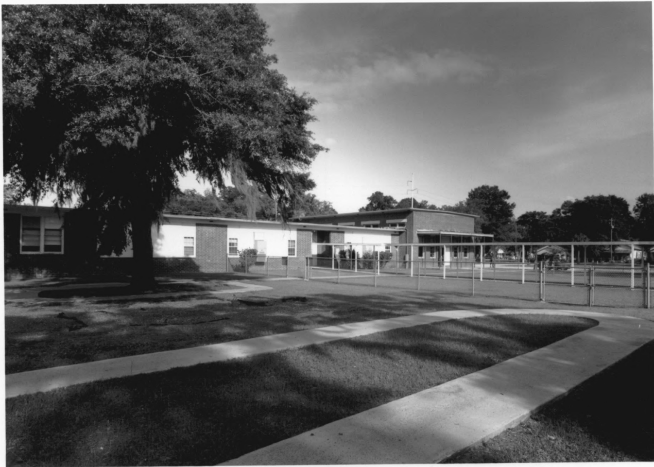
COLORED MEMORIAL SCHOOL/RISLEY HIGH SCHOOL BRUNSWICK, GLYNN COUNTY, GEORGIA PHOTOGRAPH 17 OF 18
