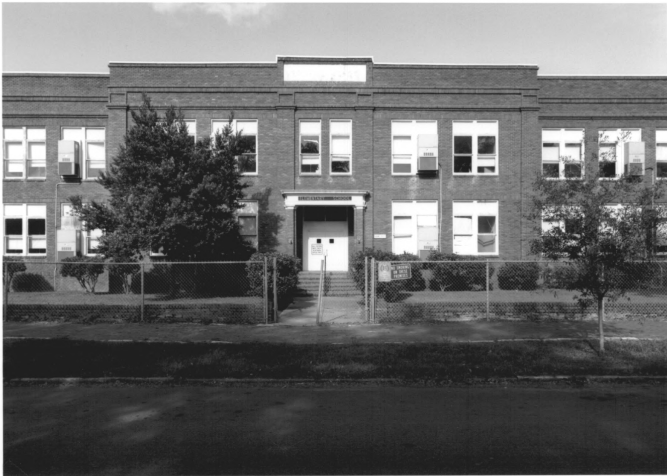
COLORED MEMORIAL SCHOOL/RISLEY HIGH SCHOOL BRUNSWICK, GLYNN COUNTY, GEORGIA PHOTOGRAPH 1 OF 18
