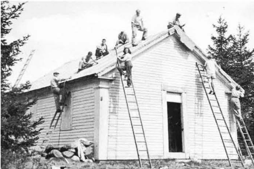
Figure 4. Roofing Bee, 1946. Courtesy of Petersham Historical Society.
