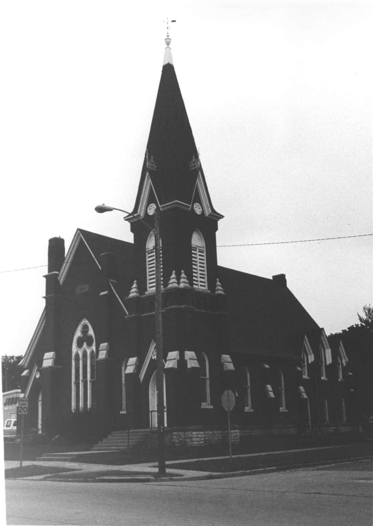
First Congregational Church N and E Elevations Camera Facing SW
