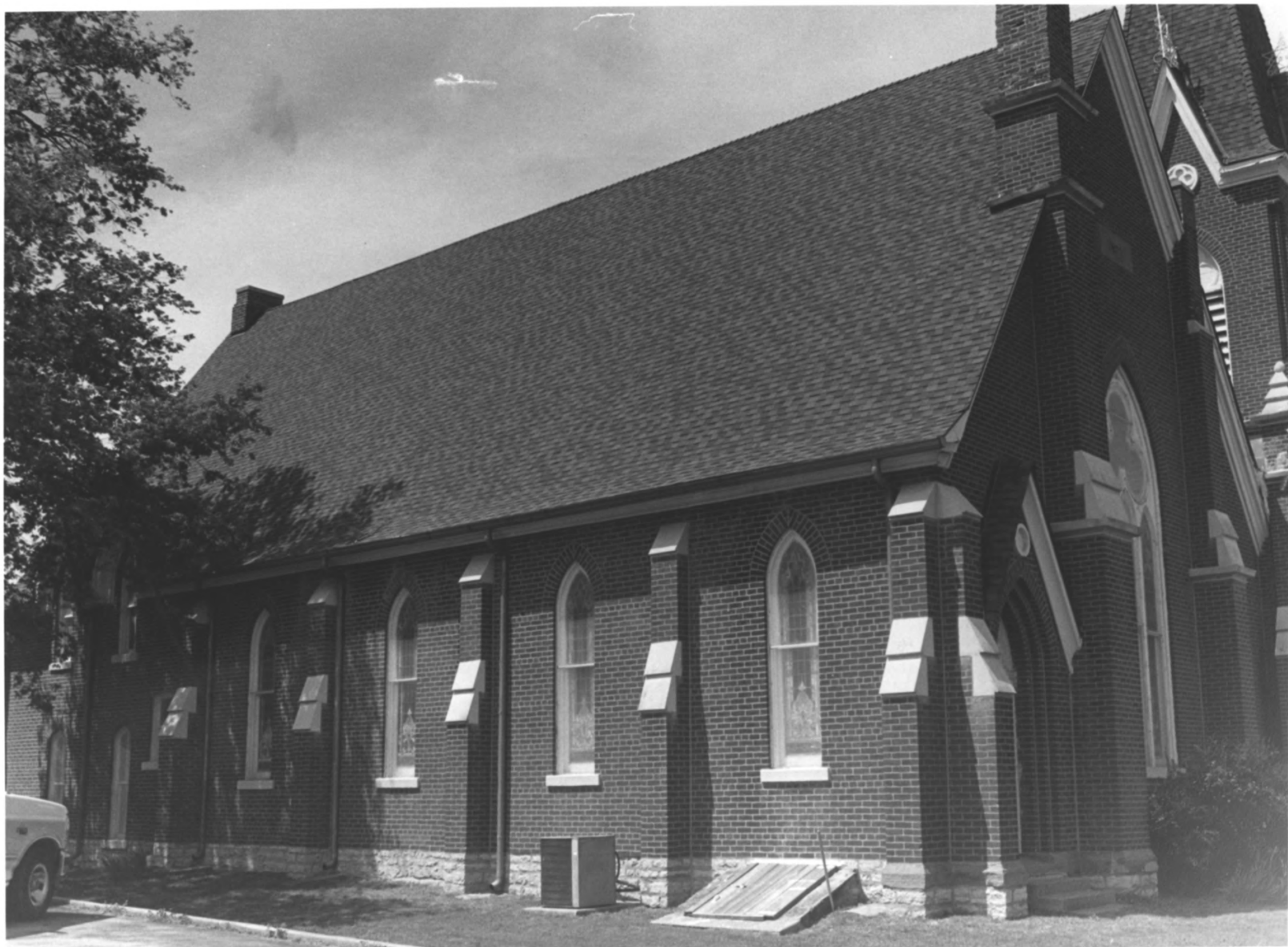
First Congregational Church Southeast elevation Camera facing NW
