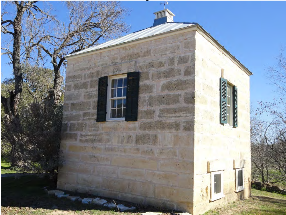
Photo 8 (TX_GillespieCounty_FellerBarsch_0008) Feller-Barsch Homestead (Resource 2) Cistern. West and south elevations looking northeast.
