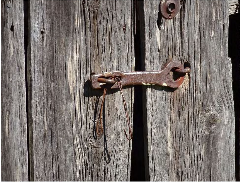
Photo 19 (TX_GillespieCounty_FellerBarsch_0019) Feller-Barsch Homestead (Resource 6) Two-story barn. Hardware on south elevation. (2017)
