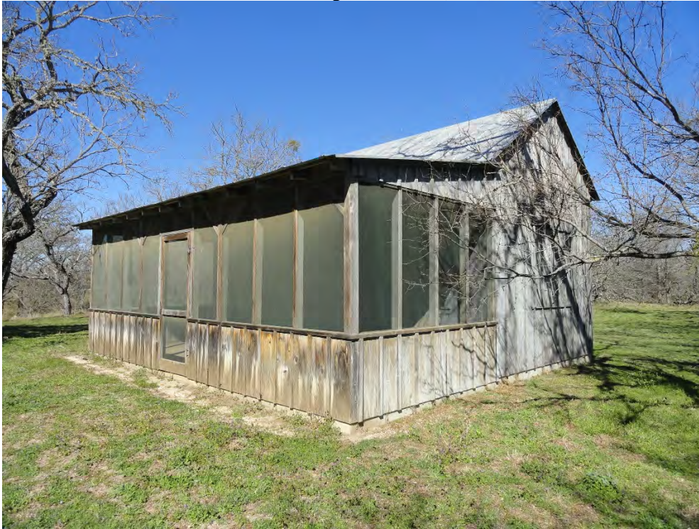
Photo 27 (TX_GillespieCounty_FellerBarsch_0027) Feller-Barsch Homestead (Resource 12) Cabin. South and east elevations looking northwest. (2015)
