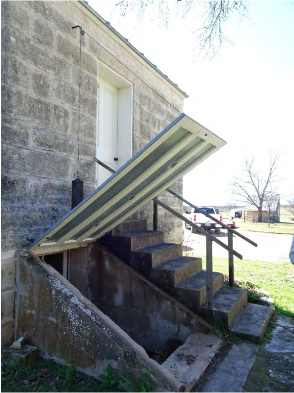
Photo 9 (TX_GillespieCounty_FellerBarsch_0009) Feller-Barsch Homestead (Resource 2) Cistern. East elevation looking west.
