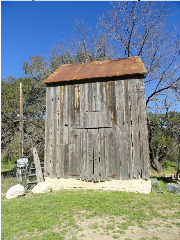
Photo 18 (TX_GillespieCounty_FellerBarsch_0018) Feller-Barsch Homestead (Resource 6) Two-story barn. South elevation looking north. (2015)
