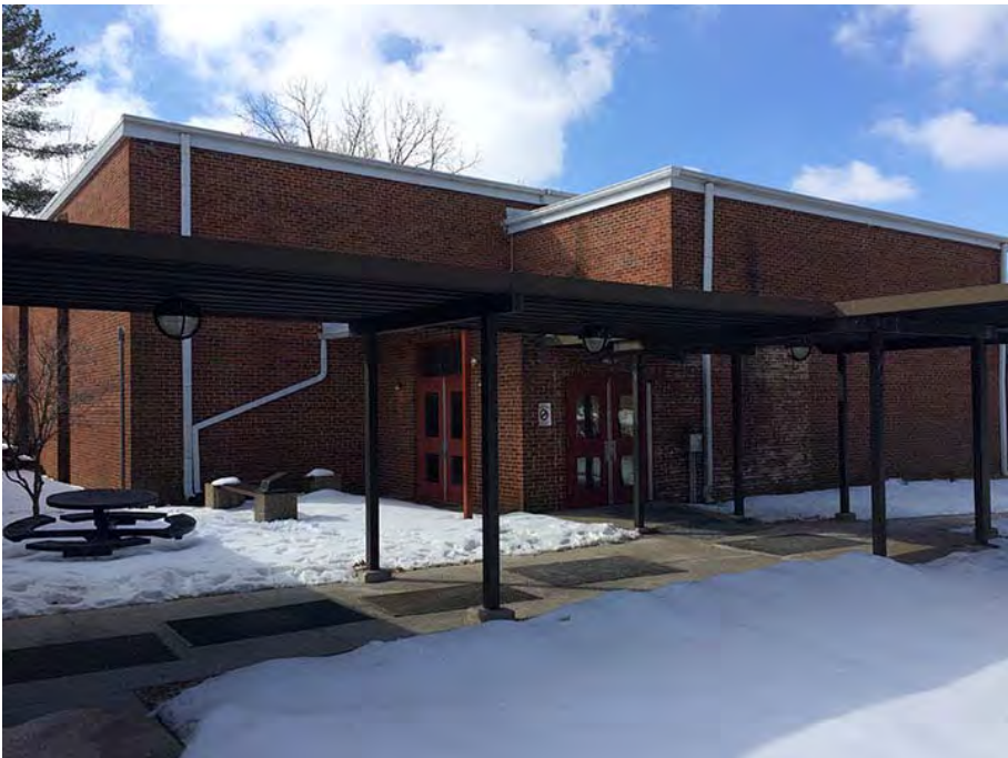
11 – Cafeteria-Gymnasium, rear entry
