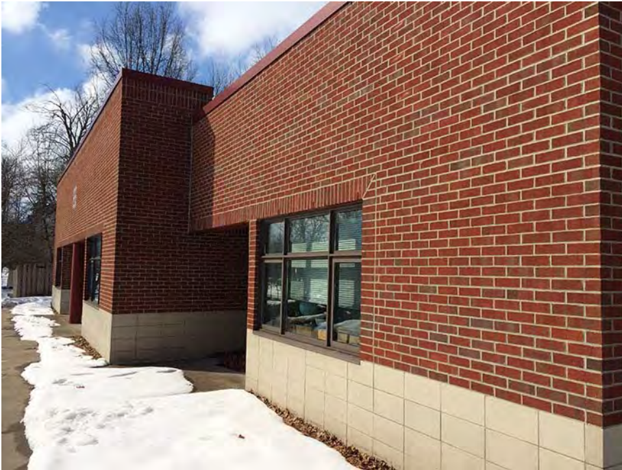
9 – Close Up-Safe Harbor Academy
