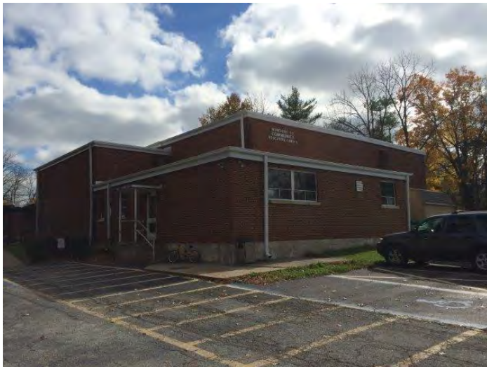
Photo 5: Cafeteria and Gym
