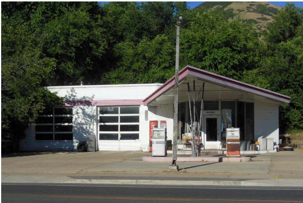
Photograph 4 West elevation of service station. Camera facing east.
