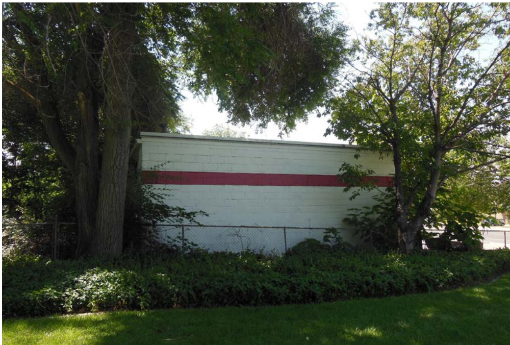
Photograph 6 North elevation of service station. Camera facing south.
