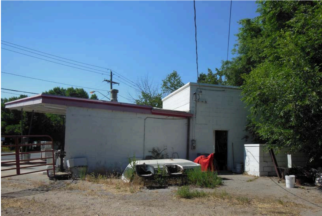
Photograph 5 East (rear) elevation of service station. Camera facing northwest.
