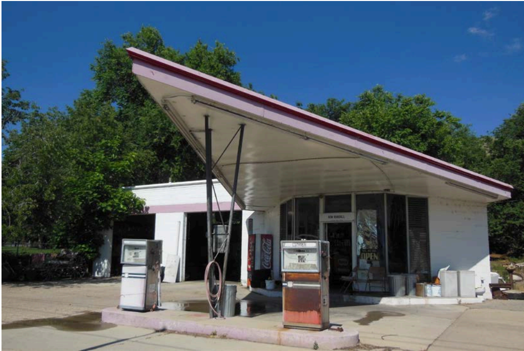
Photograph 1 West elevation of service station. Camera facing northeast.
