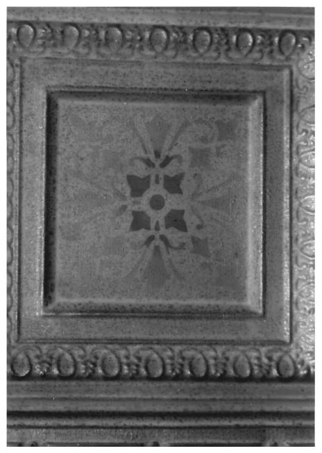
Security State Bank, Eskridge, KS. Photo credit: NP Small Neg. on file: K.S.H.S. detail of stenciled pressed metal ceiling in bank
