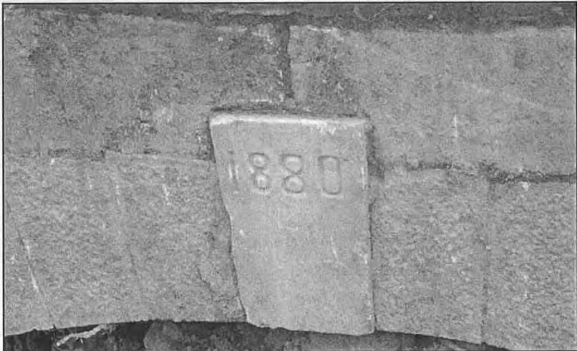
FIGURE 28: Close-up View of Keystone
