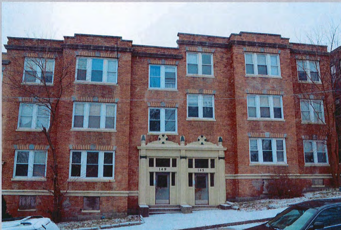
7. 145-159 Intervale Street, looking southwest
