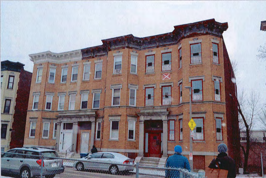
3. 123-127 Intervale Street, looking southeast
