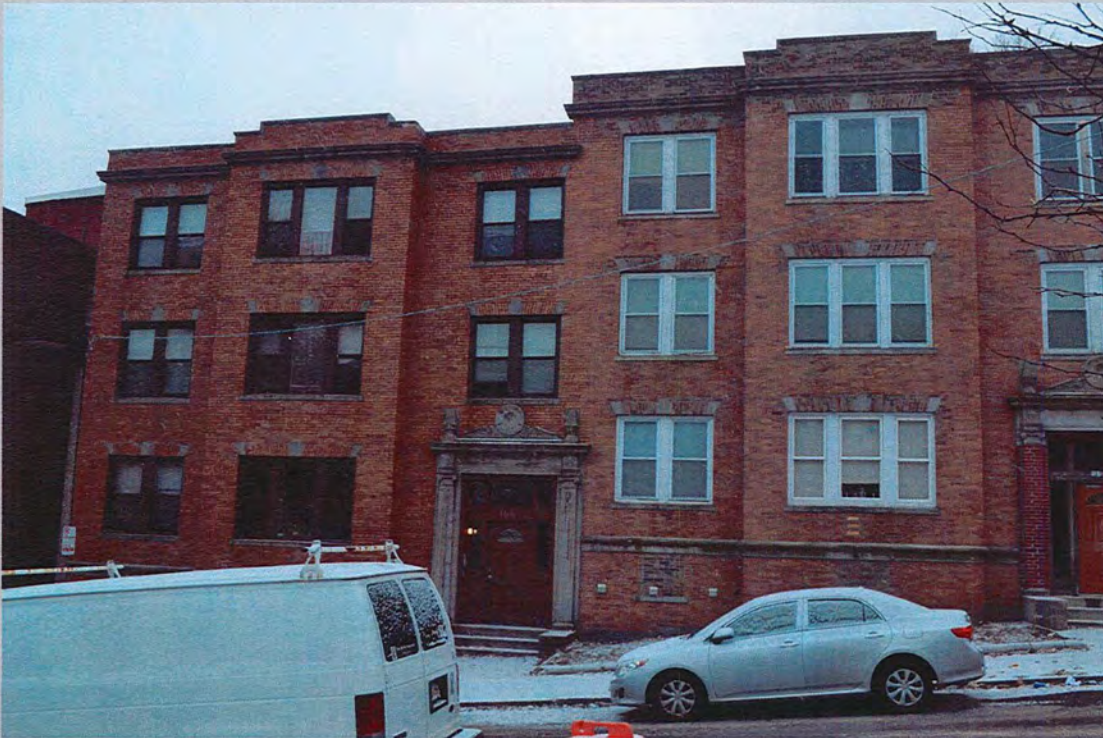
9. 145-159 Intervale Street, looking southwest
