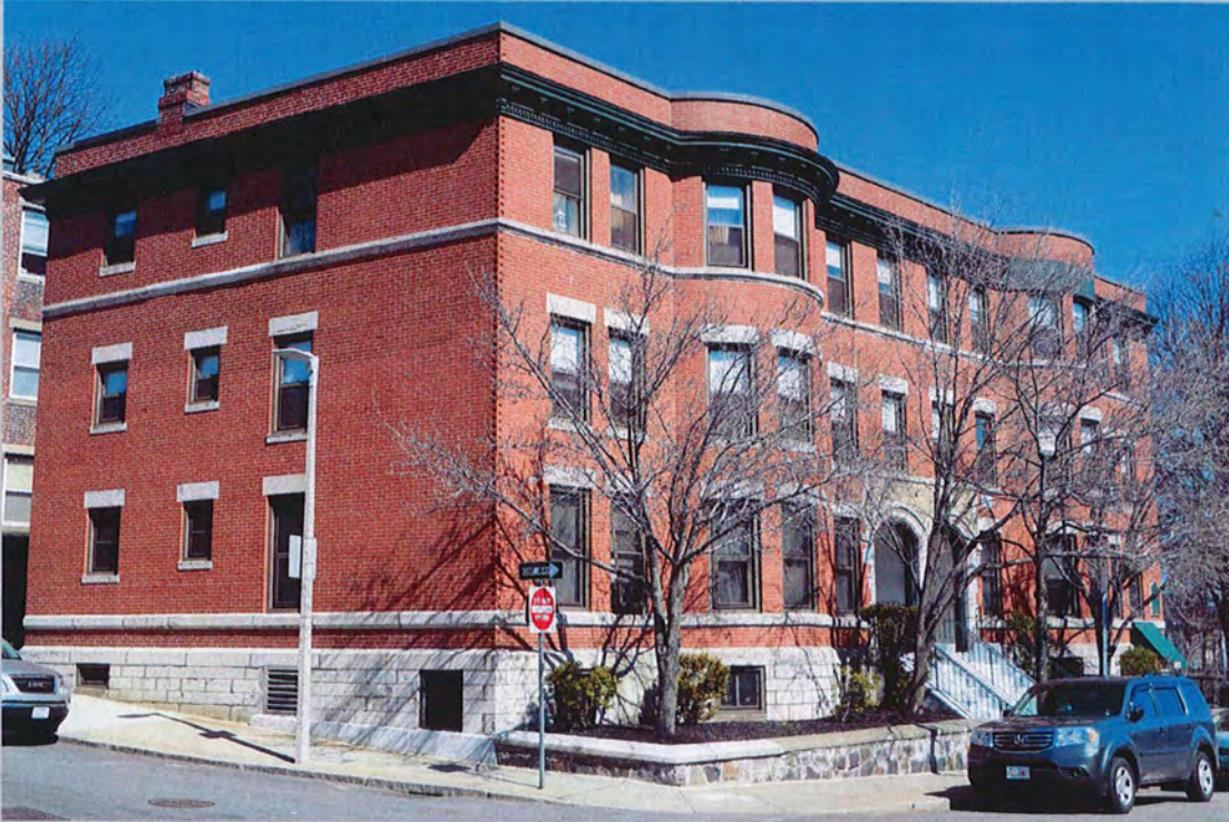
13. 286-288 Columbia Road, looking north (March 2017)
