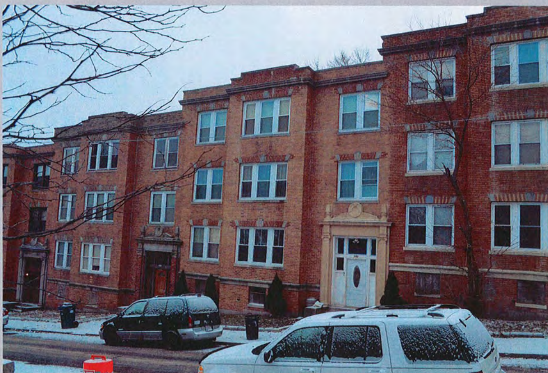
8. 145-159 Intervale Street, looking southeast
