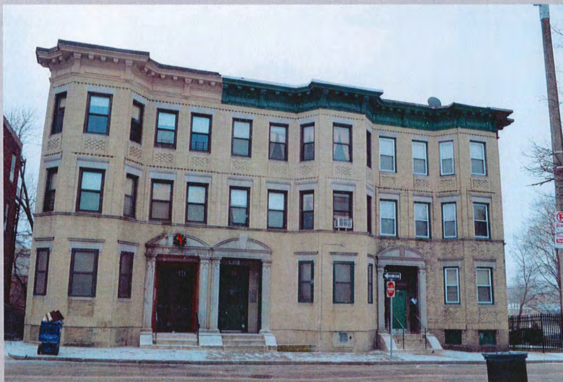
2. 117-121 Intervale Street, looking southwest
