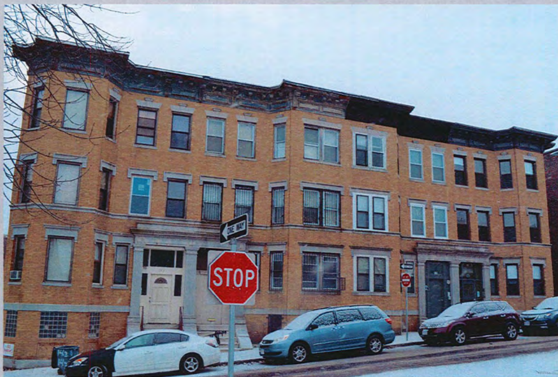
6. 137-143 Intervale Street, looking southwest
