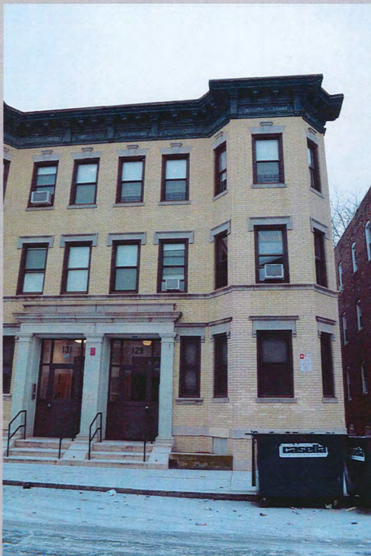
5. 129-135 Intervale Street, looking southwest
