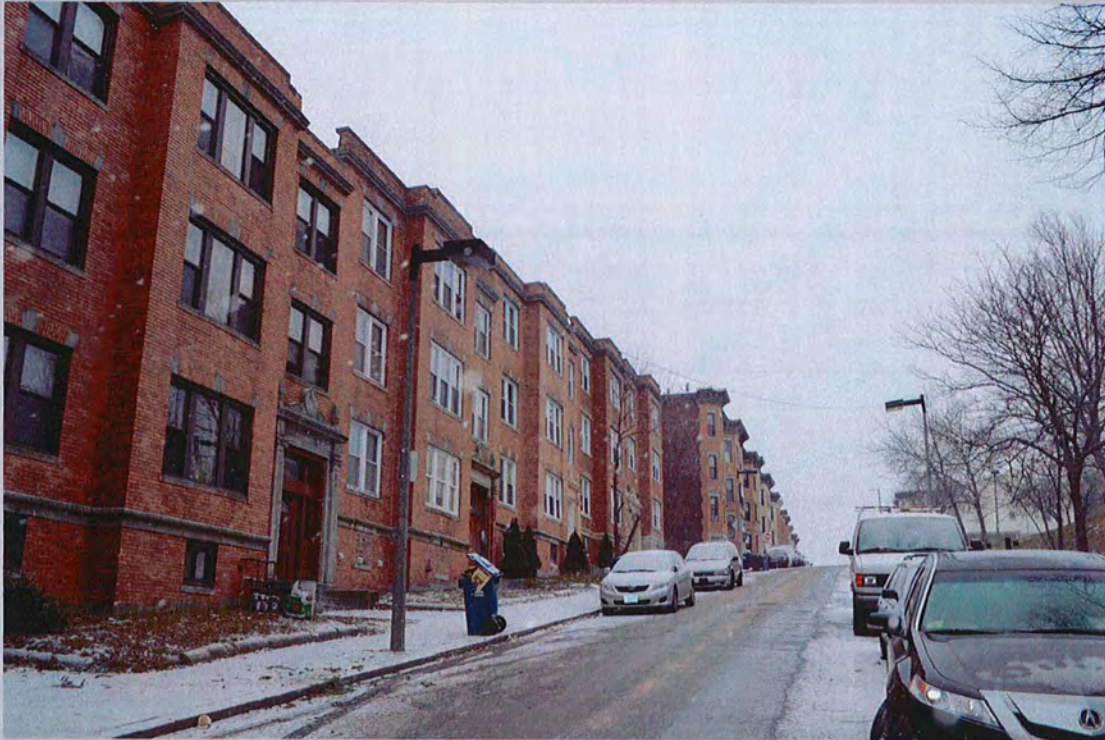
15. Intervale Street streetscape from 145-159 Intervale Street, looking northwest
