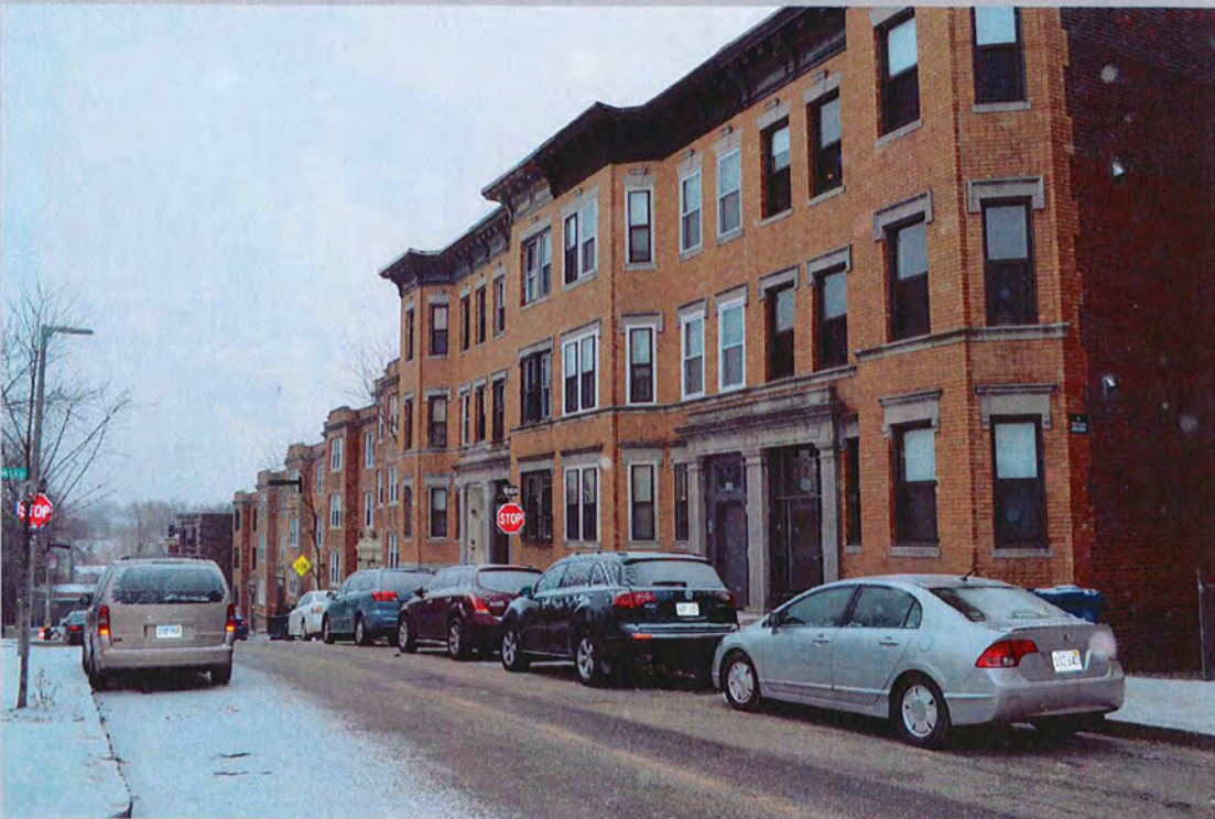
14. Intervale Street streetscape from 137-143 Intervale St., looking southeast (Jan 2015)
