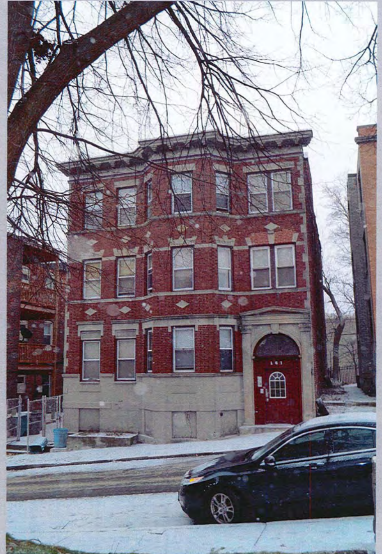
10. 161 Intervale Street, looking southwest
