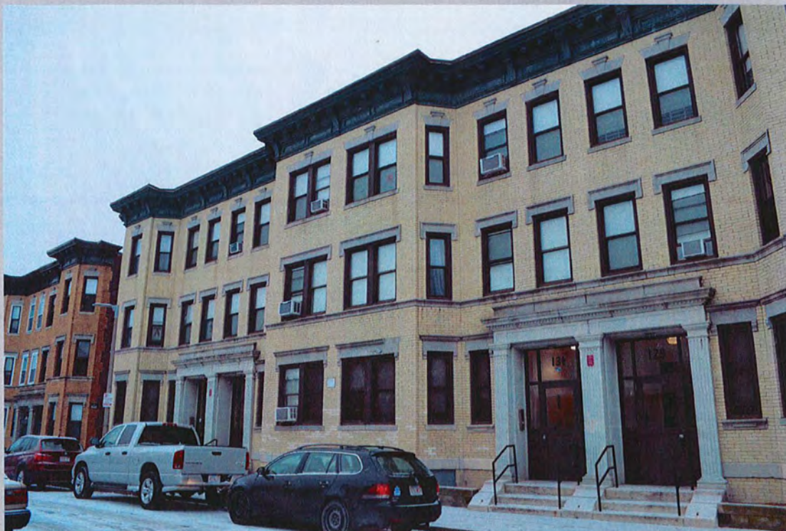
4. 129-135 Intervale Street, looking southeast
