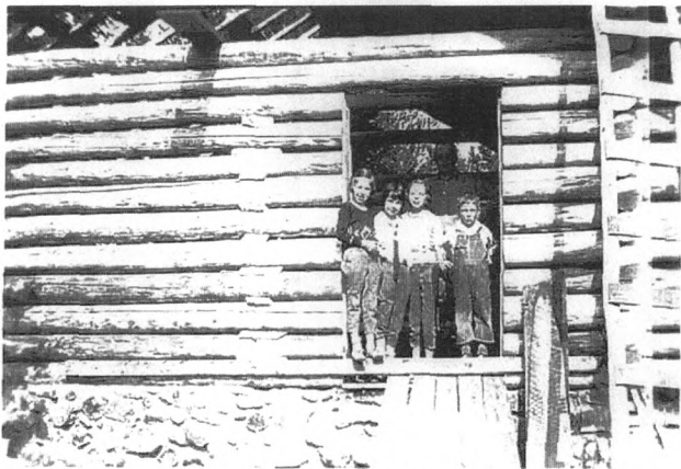
Under construction, c. 1932
