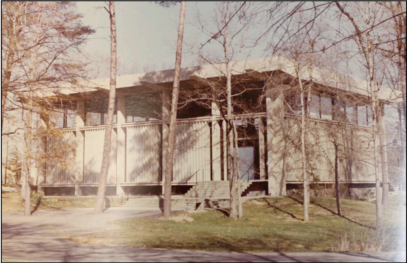
Image 27: Photograph of the west elevation of the Sanctuary, ca. 1964. From the Archives of the Unitarian Universalist Church of Arlington.
