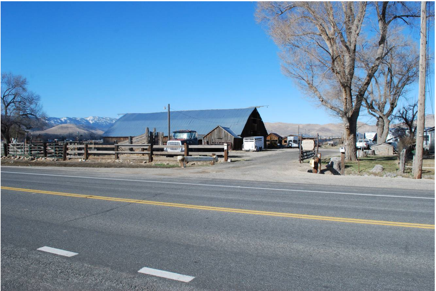
The Lompa Ranch barn and ancillary structures along Fifth Street in Carson City. Nevada SHPO, July 7, 2016.
