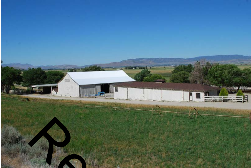
The barn (left) and accompanying equipment shed (center) at the Oscar T. Van Sickle/Pope Valley Ranch north of Mottsville, Nevada SHPO, July 7, 2016.
