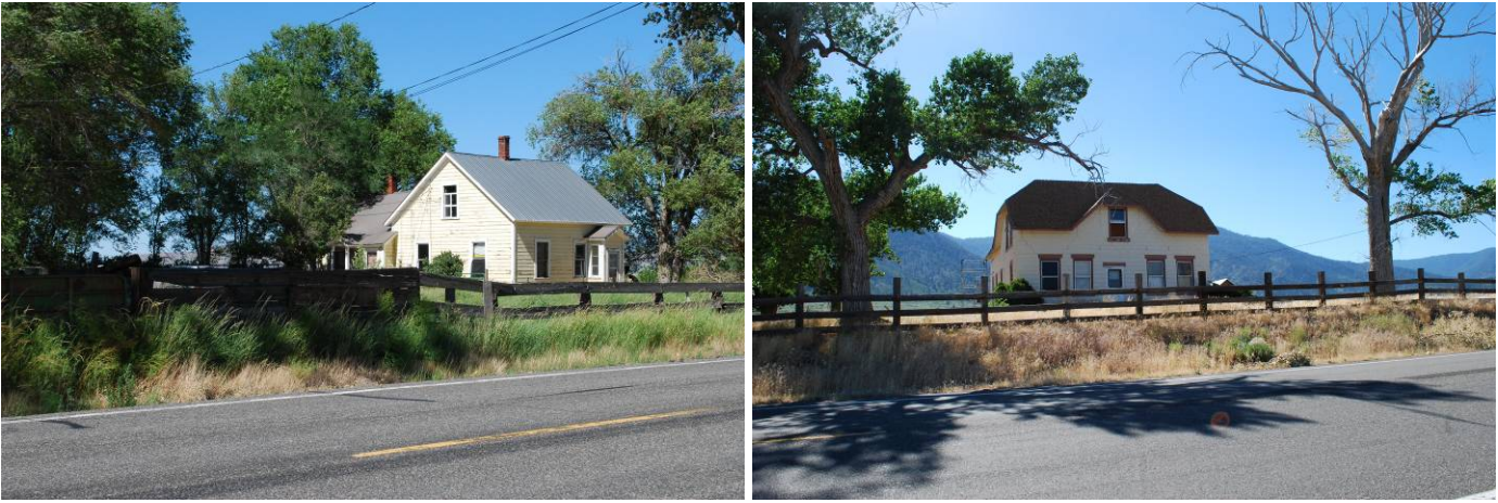
A standard Side-Gabled hall-parlor ranch house on the Muller Ranch (left) and the Johnson Ranch/BIA ranch house along Jack's Valley Road (right). Nevada SHPO, July 7, 2016.
