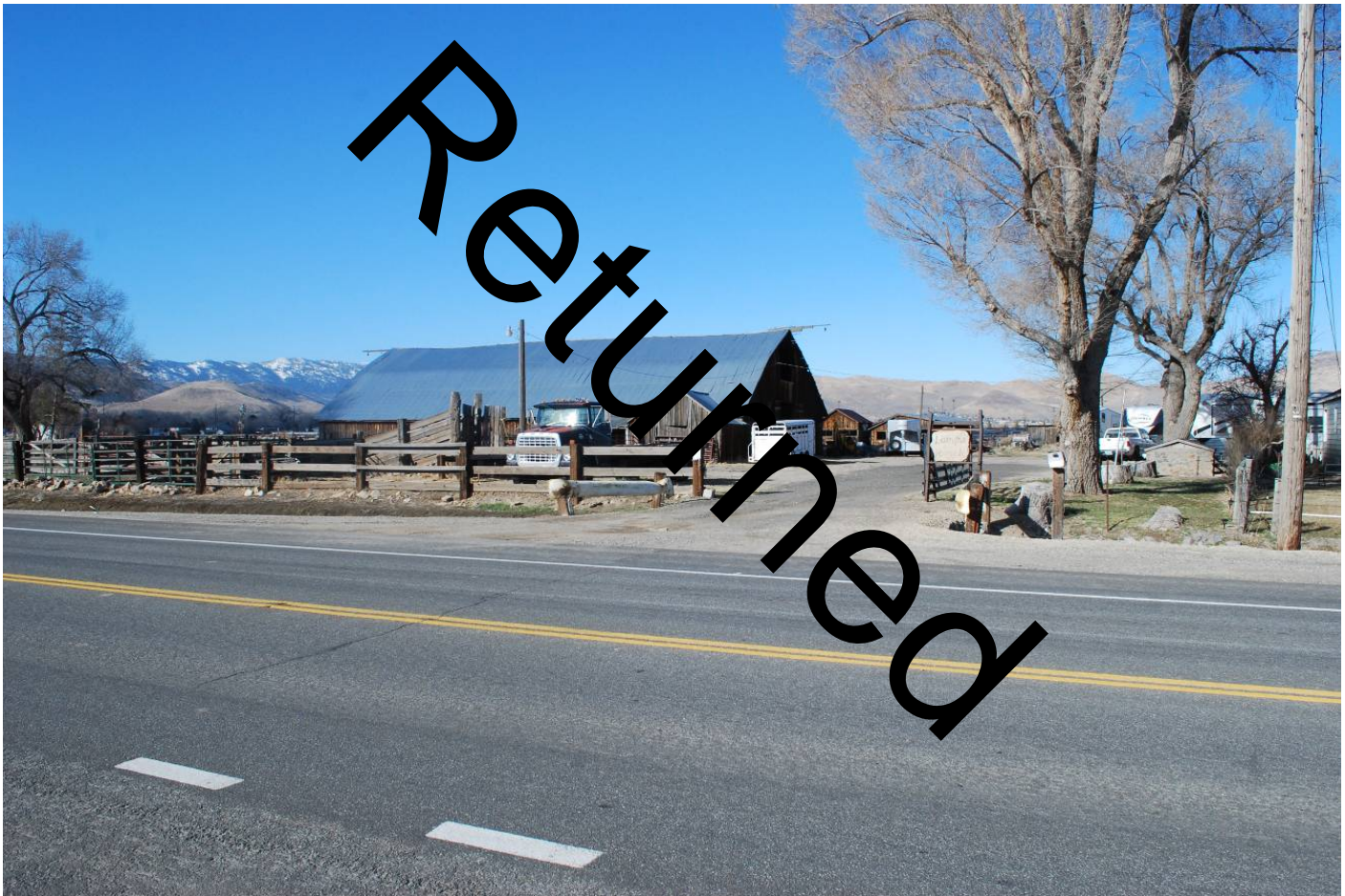
The Lompa Ranch barn and ancillary structures along Fifth Street in Carson City, Nevada SHPO, July 7, 2016.
