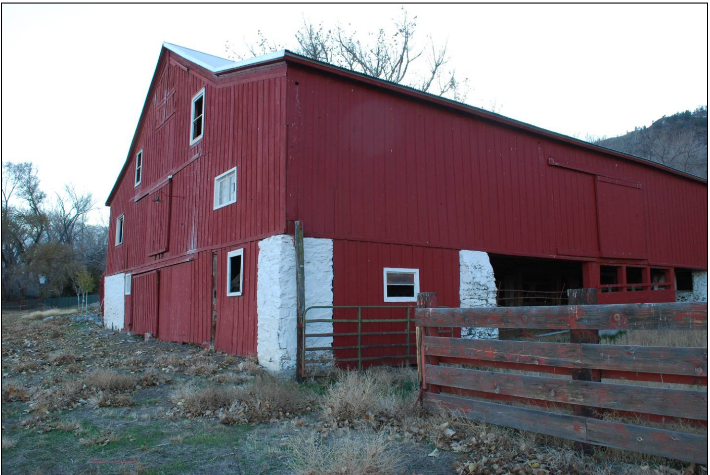
The Van Sickle Station Barn along Foothill Road, and the only known barn in Carson Valley to strictly follow German-style Bank Barn construction. Note the three levels, with a basement-level livestock space (right), a reinforced main floor for wagons and equipment (entry is centered on the south elevation not shown, with a graded dirt entry), and a hay loft above. Nevada SHPO, November 24, 2015.
