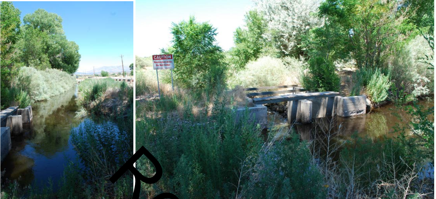
New Virginia Ditch remnant north of Tolson Avenue Nevada SHPO, July 7, 2016.
