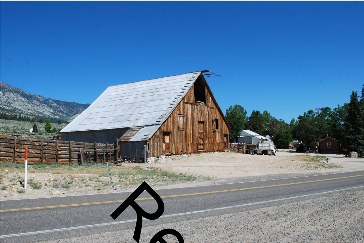
Scossa Barn along Foothill Road, an example of a High Barn. Nevada SHPO, July 7, 2016.
