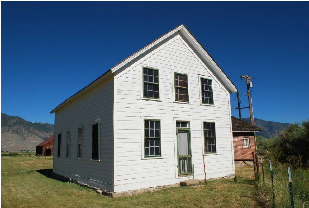
Bunk House at the Dangberg Home Ranch. Nevada SHPO, July 22, 2016.
