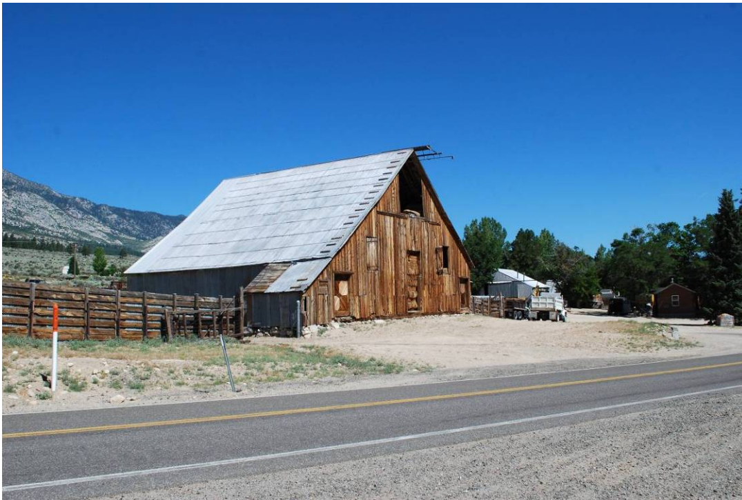
Scossa Barn along Foothill Road, an example of a Transverse Crib Barn with a flush roof. Nevada SHPO, July 7, 2016.
