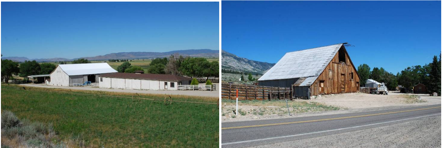
Left: The barn (left) and accompanying equipment shed (center) at the Oscar T. Van Sickle/Pope Valley Ranch north of Mottsville; Right: The Miller/Scossa Barn along Foothill Road south of Sheridan. Nevada SHPO, July 7, 2016.
