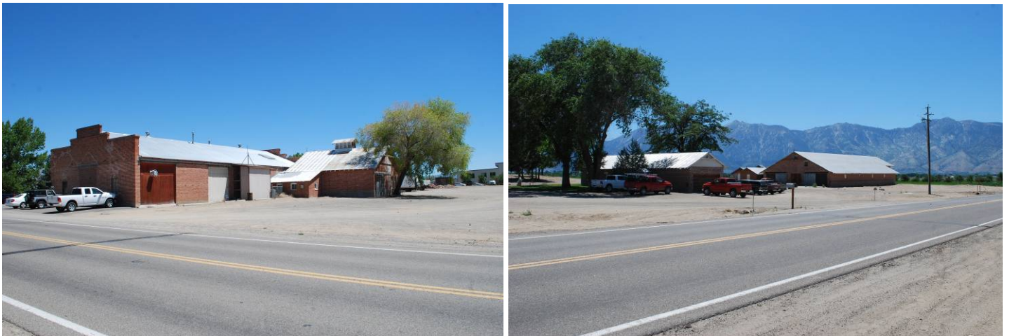
The former Buckeye Ranch property run by the Dangberg family, now owned by Bently Enterprises. Left: The storage warehouse (left) and blacksmith shop (right); Right: Housing and equipment staging area for ranch hands west of the warehouse and shops. (Both NVSHPO, July 7, 2016).
