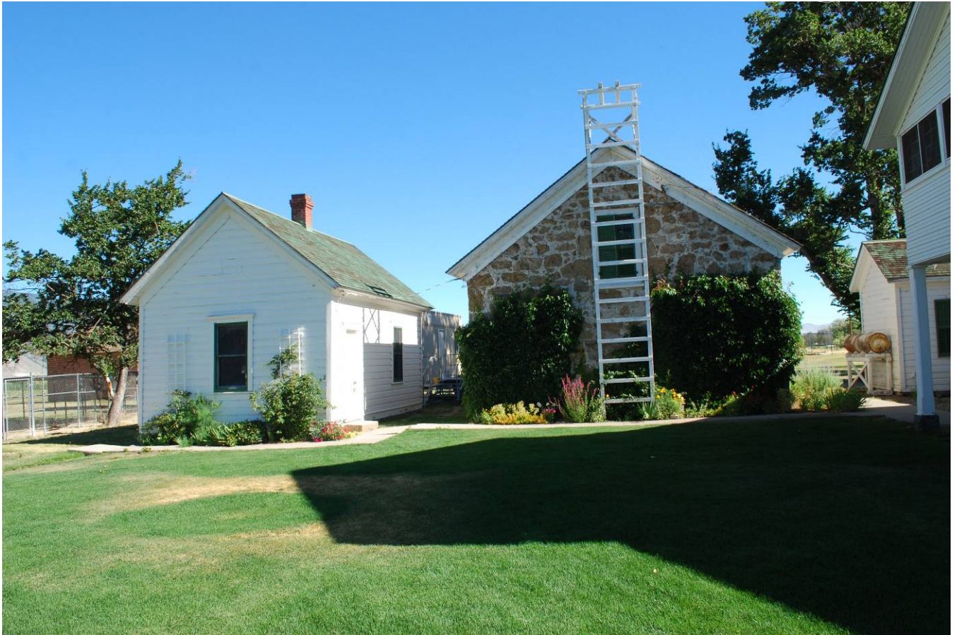
Kitchen House and Stone Cellar west of the main house, Dangberg Home Ranch south of Minden, Nevada SHPO, July 22, 2016.
