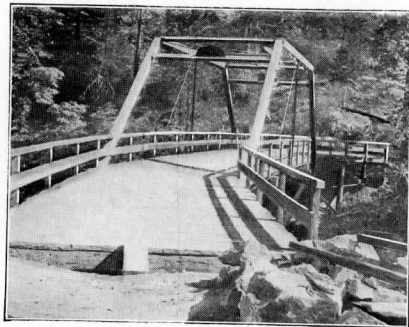
THE MARBLE FORK BRIDGE.
