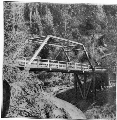
THE MARBLE FORK BRIDGE.
