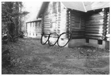
SOUTH SIDE REPAIR WORK OR BEAM POCKETS SHOWN FILLED WITH TWO VENT HOLES LEPTOPEN. ALSO THIS SIDE WILL TAKE BACKFILL HOELY AS WILL THE SOUTH east and east St. John the Evangelist Roman Cartalic Church Clockamus Co, Origon
