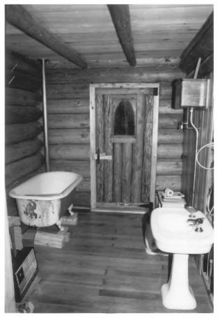
BATH WING PARTIALLY COMPLETED BATH AREA USING OLD FIXTURES OF CHURCH ERA. NOTE EXPOSED CUPPER VENT PIPE BEHND TUB. IT WAS NECESSARY TO WEET CODE BUT TASTEFULLY DONE. It. John the boungelist Roman
