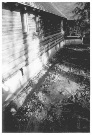
SOUTH SIDE shows Approximately HOW DRAINAGE TRENCH WILL RUY. DRAIN PIPE WILL LAY IN TRENCH FILLED WITH MEAIN ROCK AND THEN APPROX 18" OF FILL DIRT
