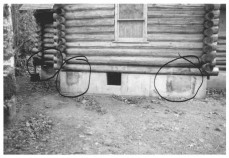
NORTH WING THREE OF THE BEAM POCKETS I POURED IN PREPARATION For rockwork and BACKFILL. ELECTRICAL PANELS
