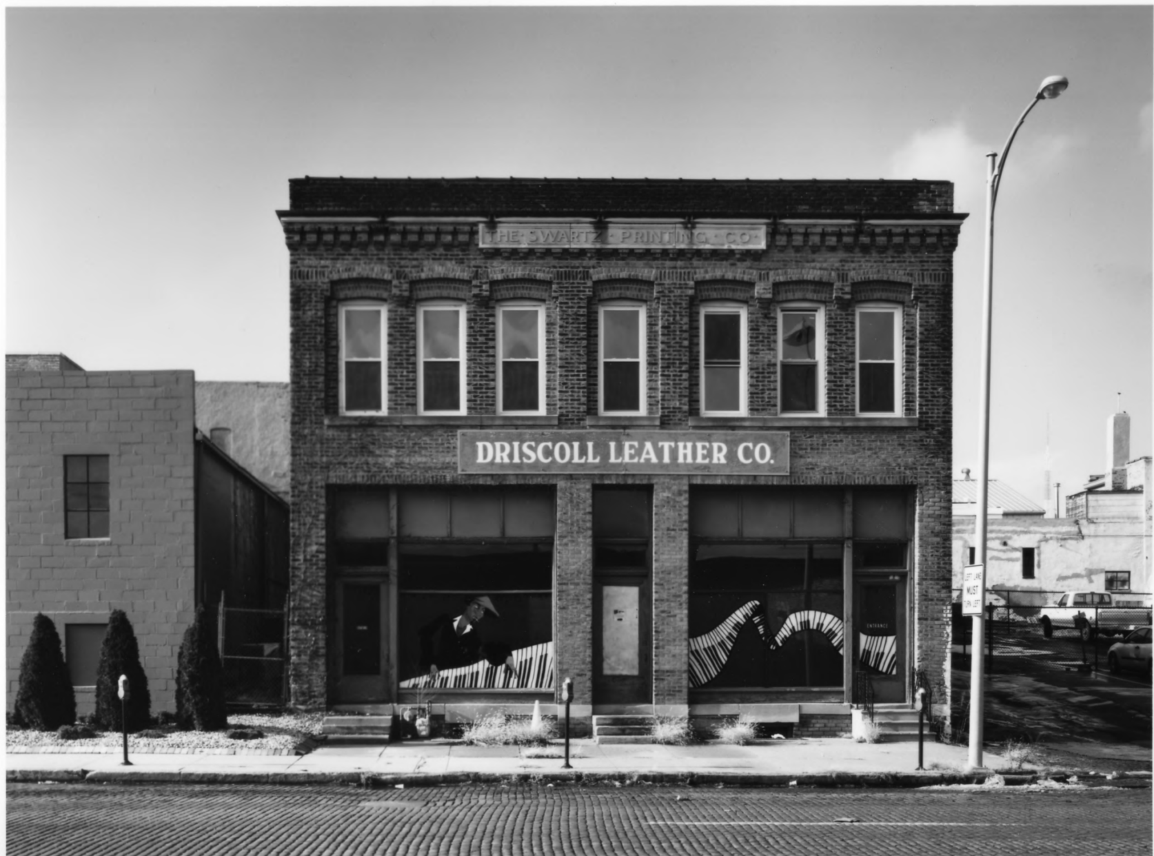
SWARTZ PRINTING COMPANY BUILDING DOUGLAS COUNTY, NEBRASKA PHOTO 1 OF 7
