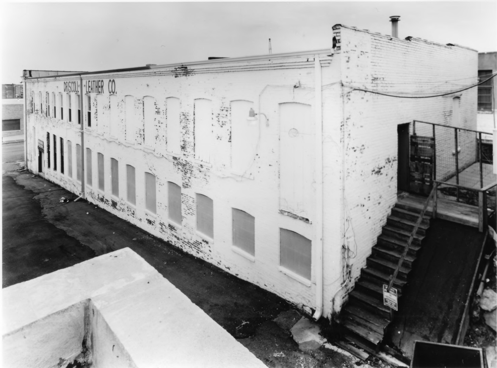
SWARTZ PRINTING COMPANY BUILDING, DOUGLAS COUNTY, NEBRASKA PHOTO 3 OF 7
