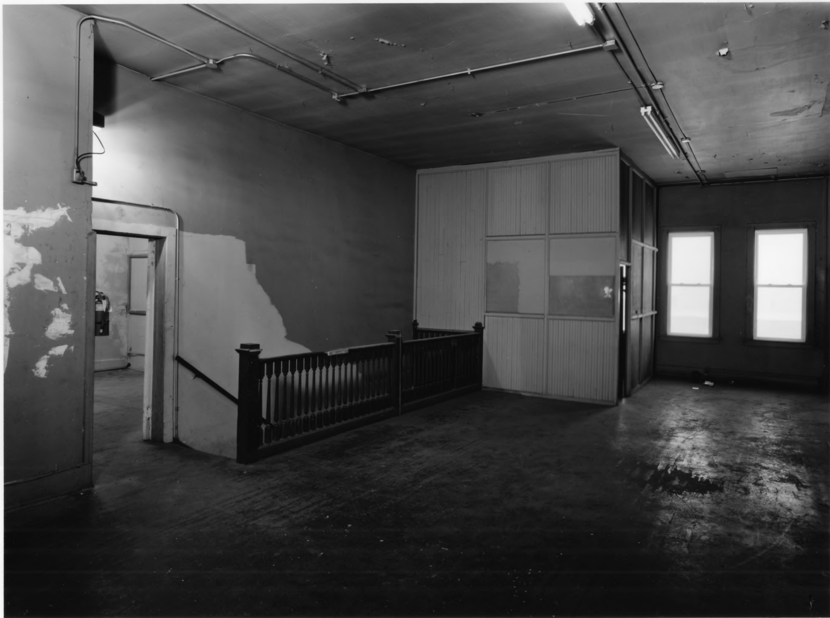
SWARTZ PRINTING COMPANY BUILDING, DOUGLAS COUNTY, NEBRASKA PHOTO 7 OF 7
