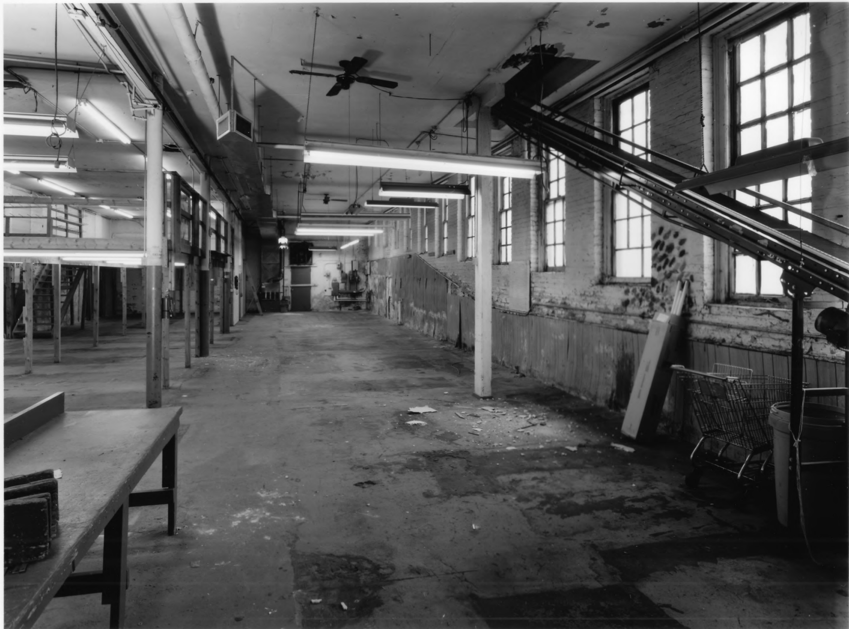
SWARTZ PRINTING COMPANY BUILDING DOUGLAS COUNTY, NEBRASKA PHOTO 4 OF 7
