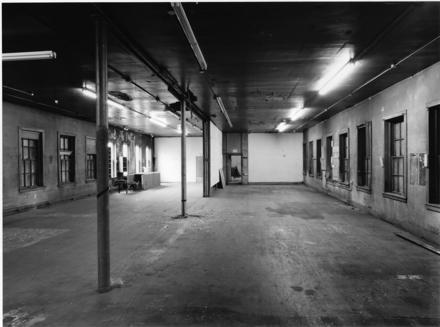
SWARTZ PRINTING COMPANY BUILDING DOUGLAS COUNTY, NEBRASKA PHOTO 6 OF 7
