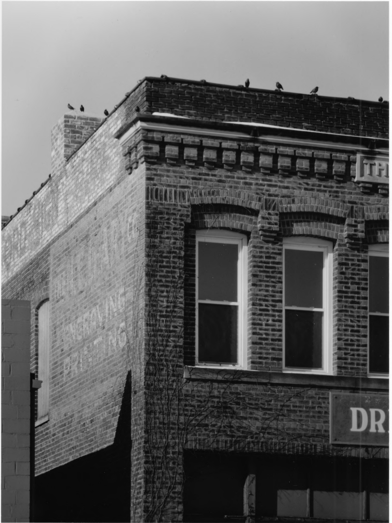
SWARTZ PRINTING COMPANY BUILDING DOUGLAS COUNTY, NEBRASKA PHOTO 2 OF 7
