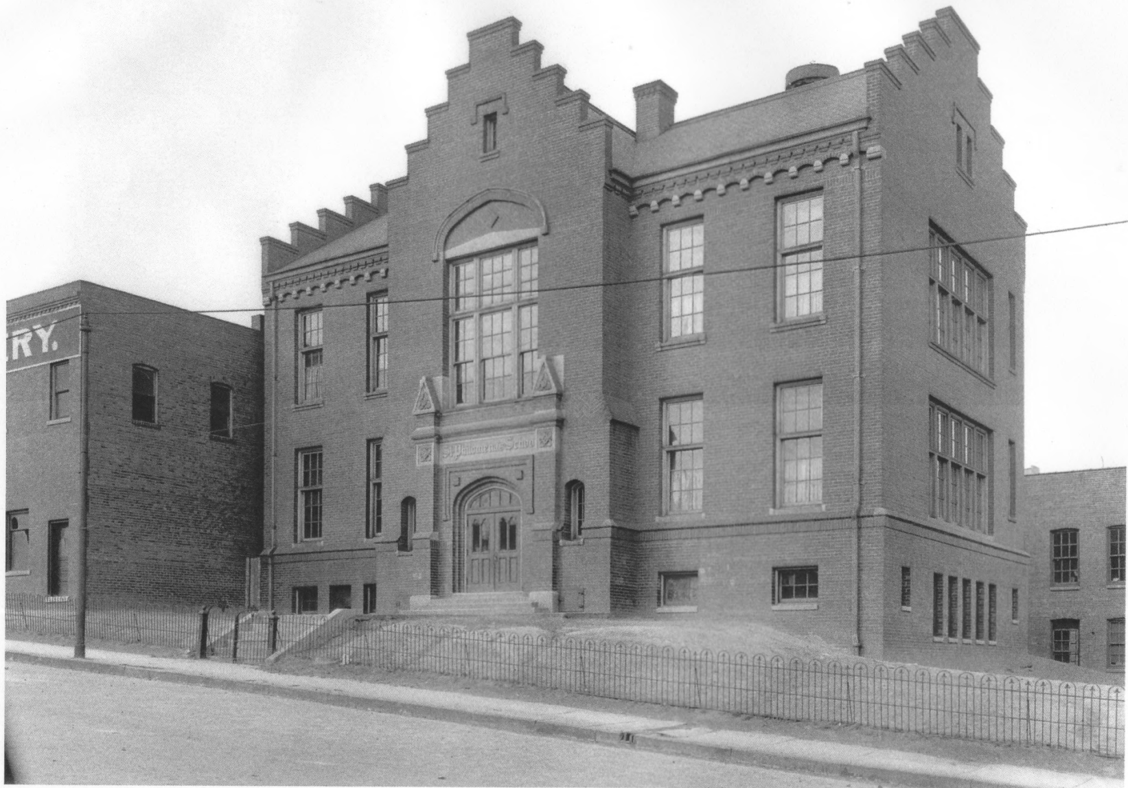
Swartz Printing Company Building Douglas County, Nebraska Supplemental Photo 3 of 4
