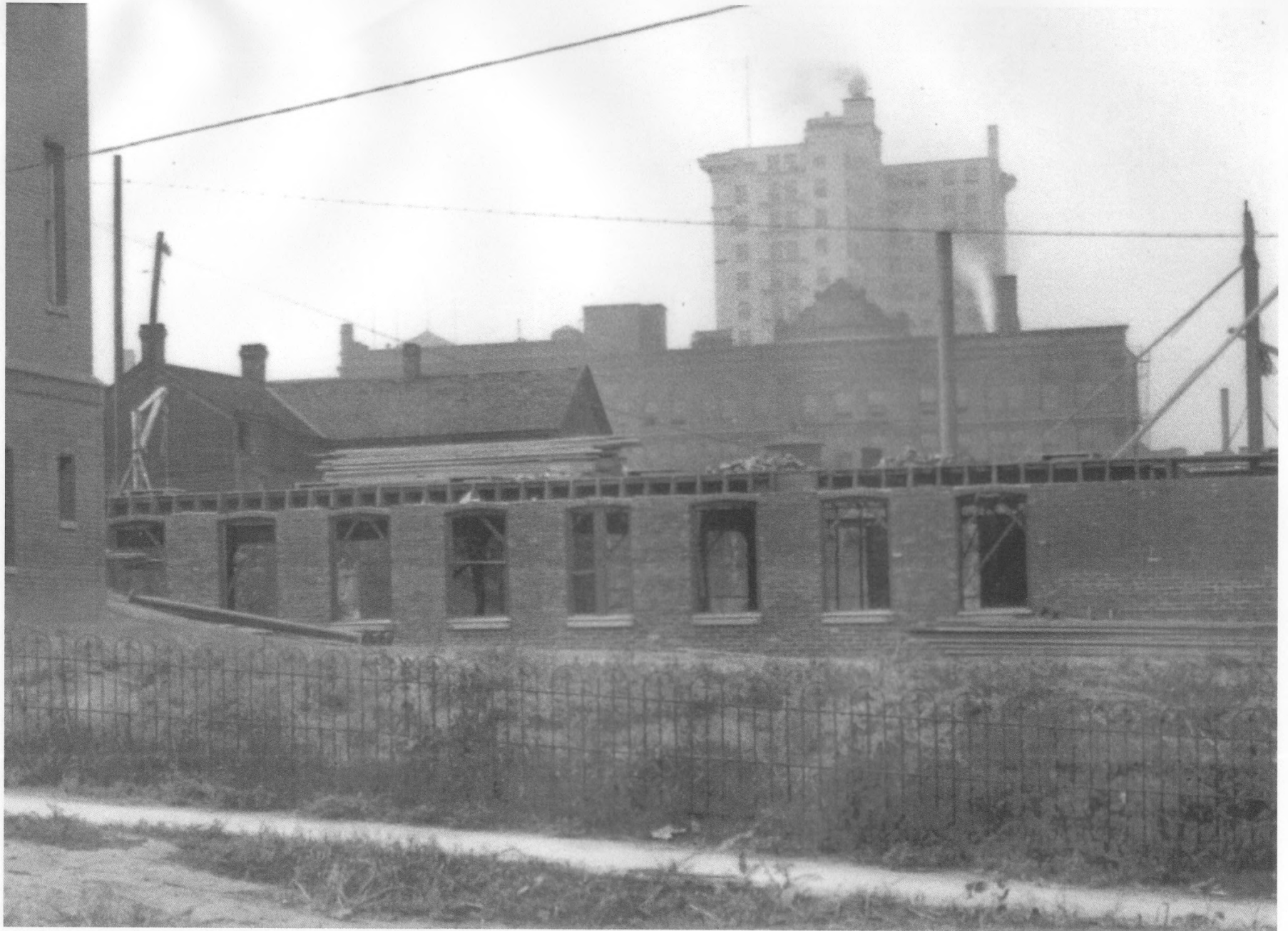
Swartz Printing Company Building Douglas County, Nebraska Supplemental Photo 2 of 4
