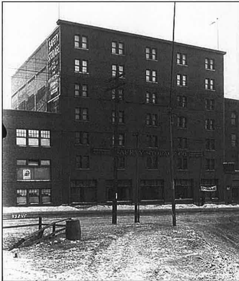
Figure 1: A historic photograph showing the west and north walls of 708 Central. Photograph by Charles H. Hibbard, 1923. Source: Minnesota Historical Society.
