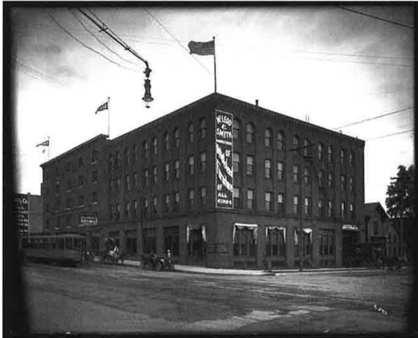
Figure 2: A historic photograph showing the west (left) and south (right) facades. Photograph by Charles P. Gibson, 1913-1914. Source: Minnesota Historical Society.
