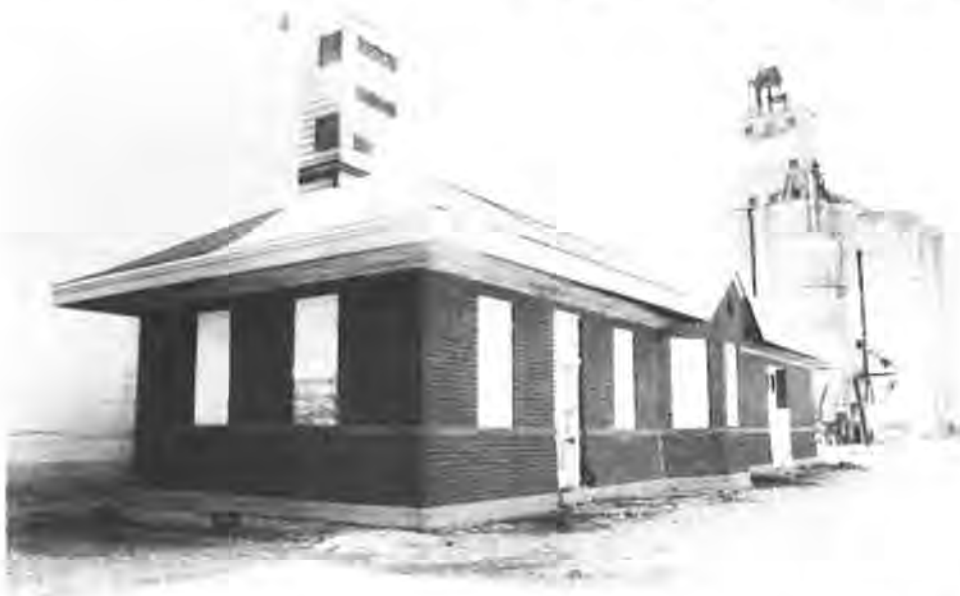
Figure 1: View of the south side and east facade of the Minburn Depot at the original location, camera pointed to the north/northwest. Photo taken on July 26, 2013 by Sheriffa Jones.
