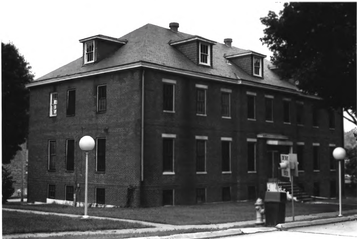
TN SCHOOL FOR THE DEAF HISTORIC DISTRICT KNOX CO., TN # 2056
