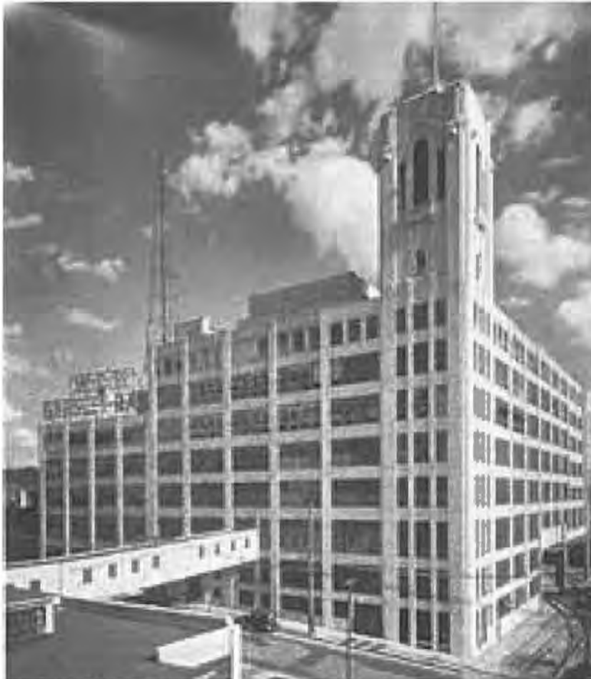
Photo 1 --Historic Photo showing the elevated connector and construction complete. Source: Crosley Automobile Club, Inc. 307 Schoefer Rd. Blandon, PA
