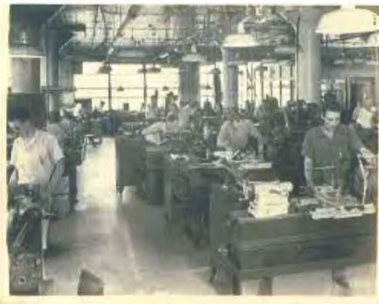
Photo 3 -- Historic Interior view of the building. Source: Crosley Automobile Club, Inc. 307 Schoefer Rd., Blandon, PA
