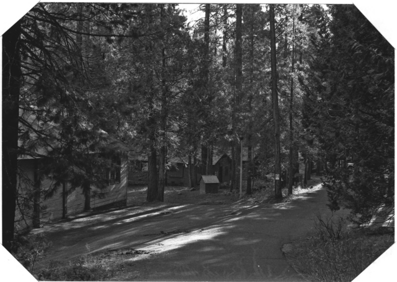
1 Setting. Overview of east end of Stanislaus Branch Station. Corner of warehouse (Building 2220) in foreground, left, and dormitory (Building 1346) visible among the trees. View toward southwest (210°).
