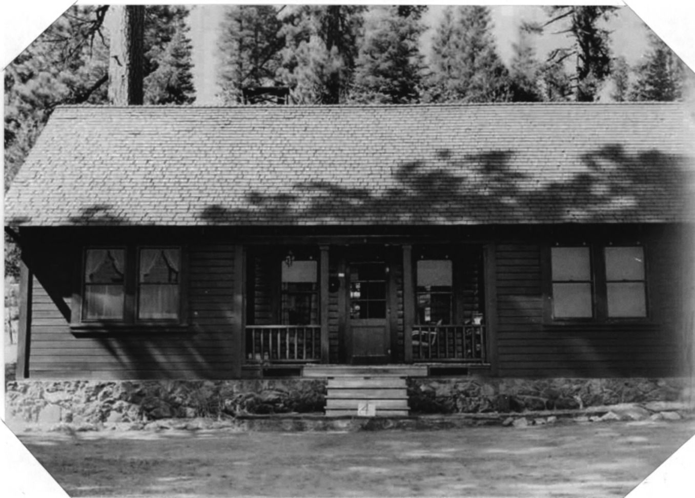
Caretaker's residence, front façade, 1958. Building 1110.
