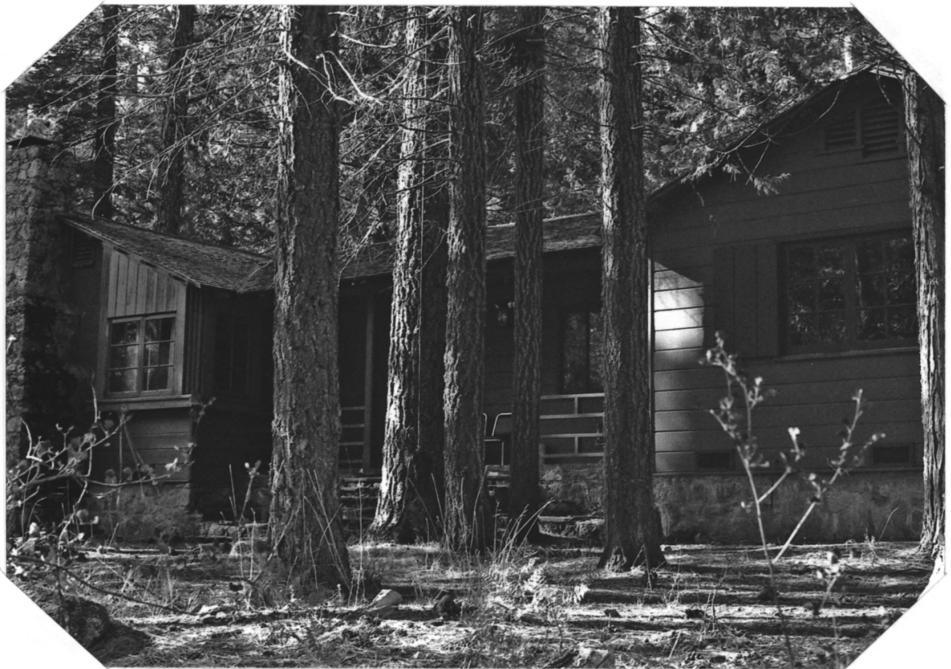
10 Dormitory, front (porch faces South Fork Stanislaus River). Building 1346. View toward northwest (290°).
