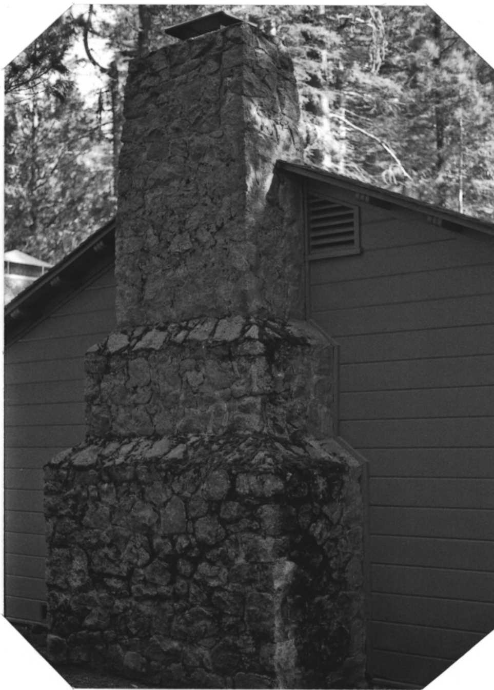
16 Dormitory, rear of west wing; chimney detail. Building 1346.
