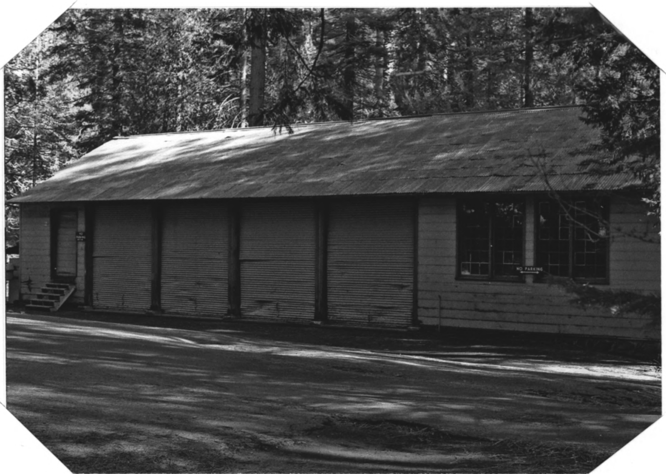
7 Warehouse, front. Building 2220. View toward east (90°).
