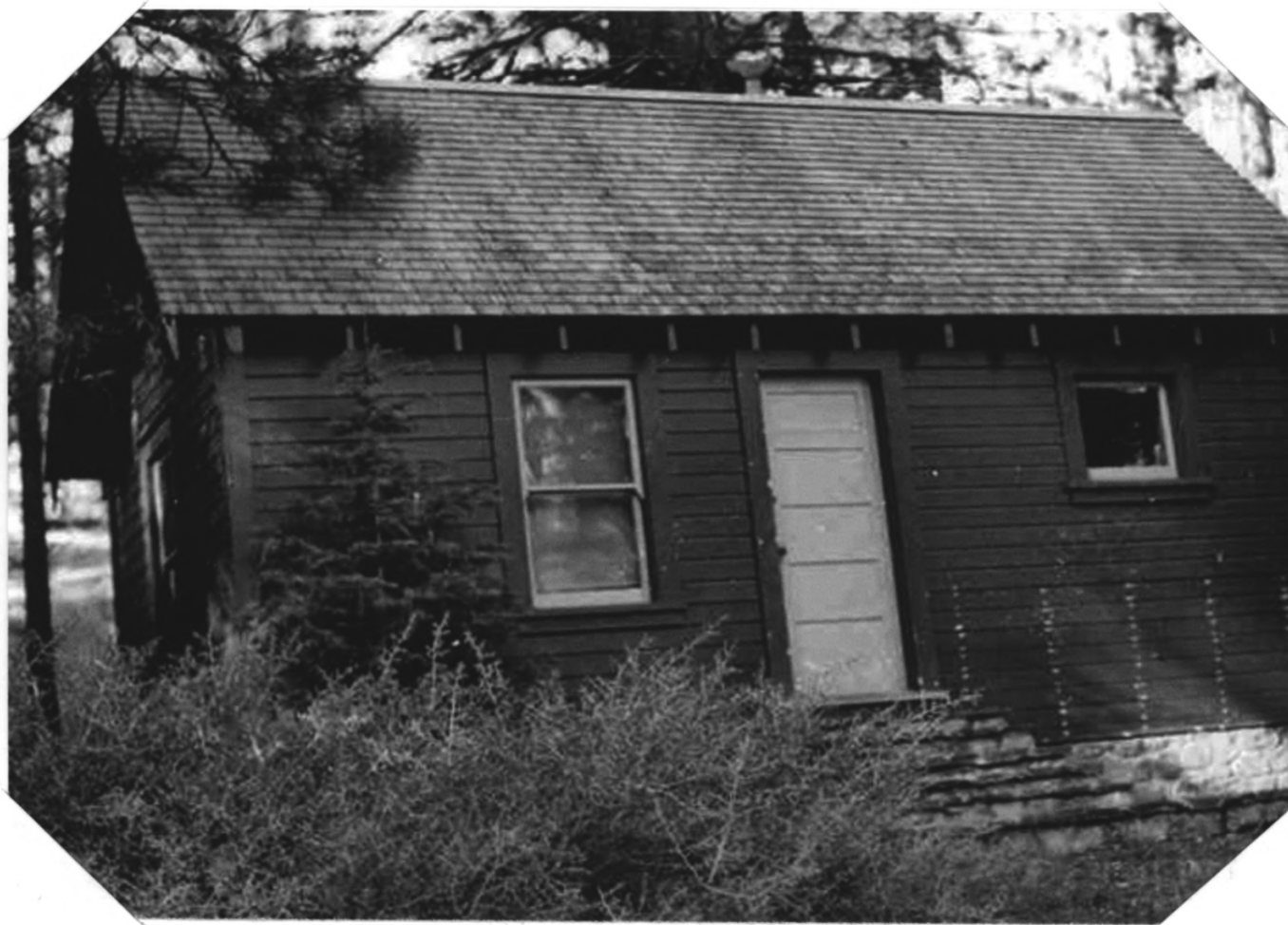
Cabin (original laboratory) front façade, 1931. Building 1218.
