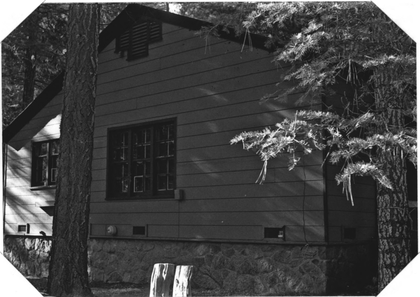
21 Laboratory, south gable end. Building 1111. View toward northwest (280°).
