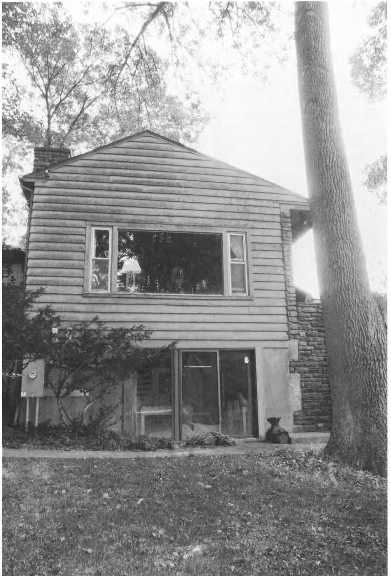
901 Mt. Lebanon Road, New Castle County, DE North elevation of rear den section with sliding door to lower level and stone retaining wall for elevated rear patio area looking south
