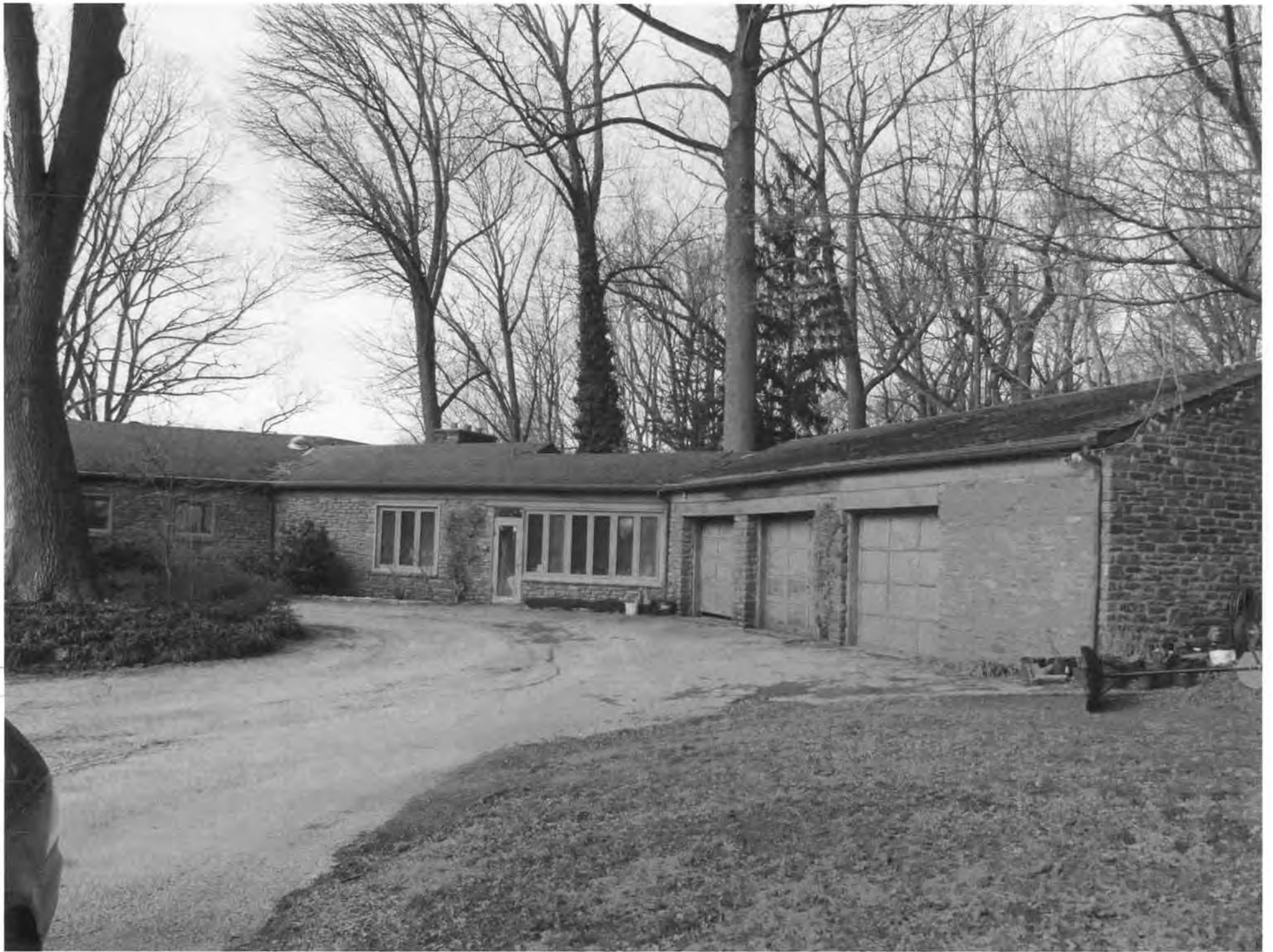
901 Mt. Lebanon Road_New Castle County_DE Southeast elevation of kitchen section, garage wing, and driveway looking northwest
