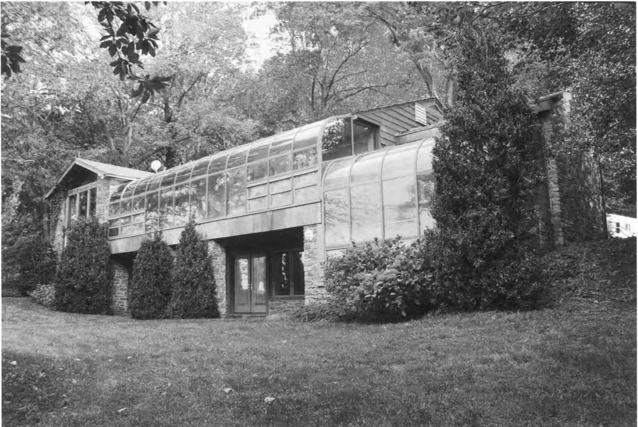
901 Mt. Lebanon Road, New Castle County, DE West elevation of den section, bedroom wing, sunroom addition, recessed entrance to lower level bedrooms looking northeast
