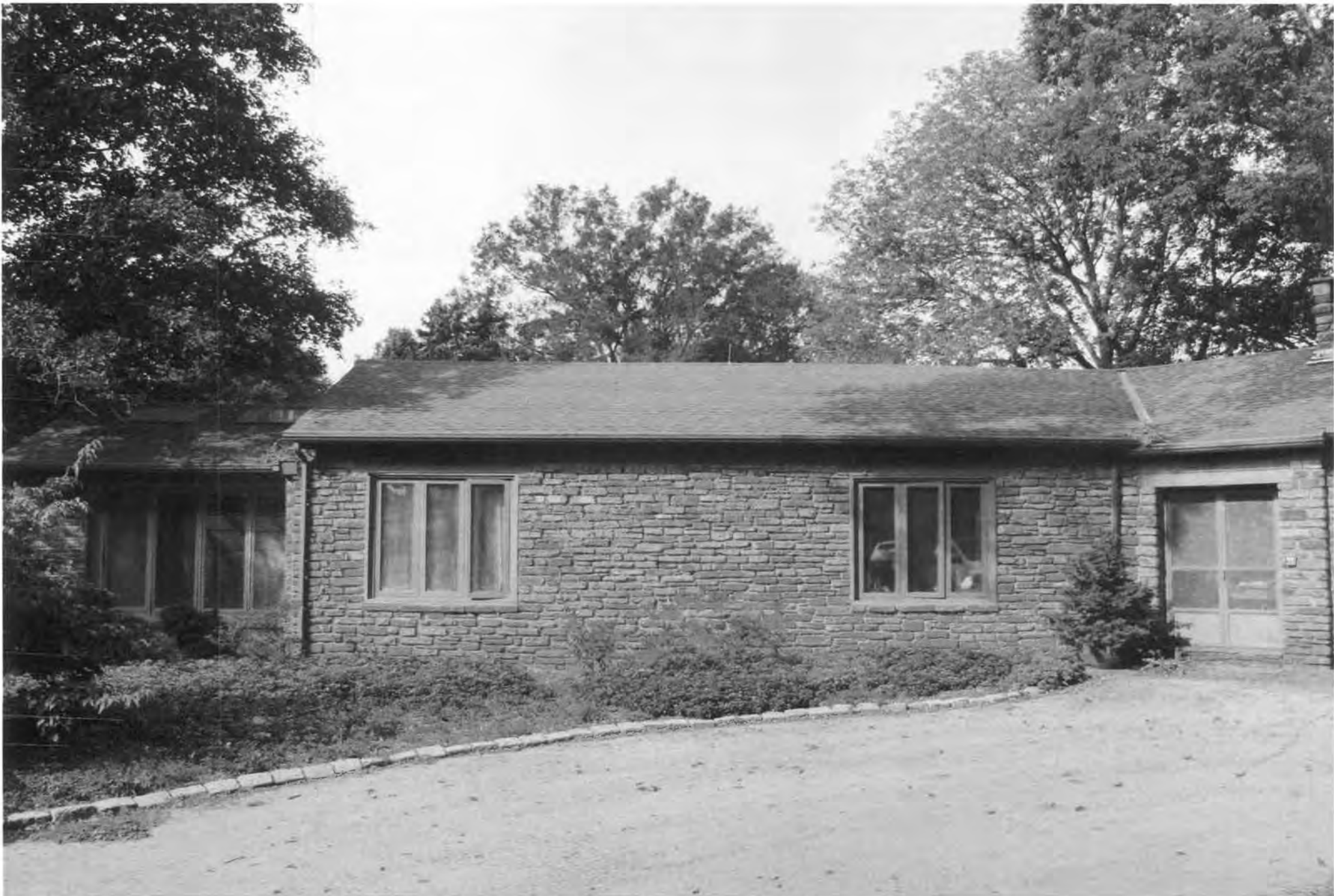
901 Mt. Lebanon Road_New Castle County_DE East elevation of bedroom wing looking west
