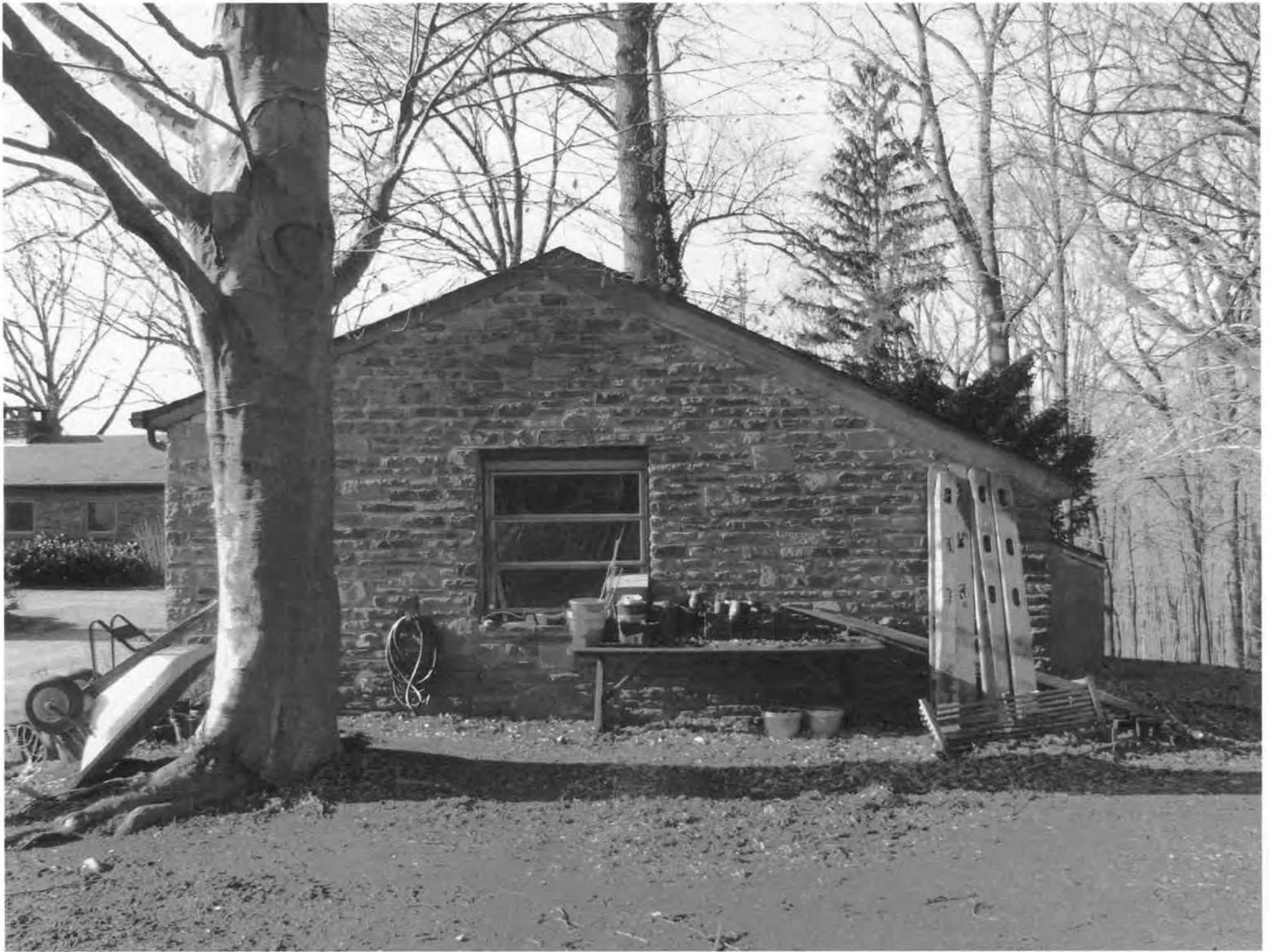
901 Mt. Lebanon Road_New Castle County_DE Southeast elevation of three-bay garage
