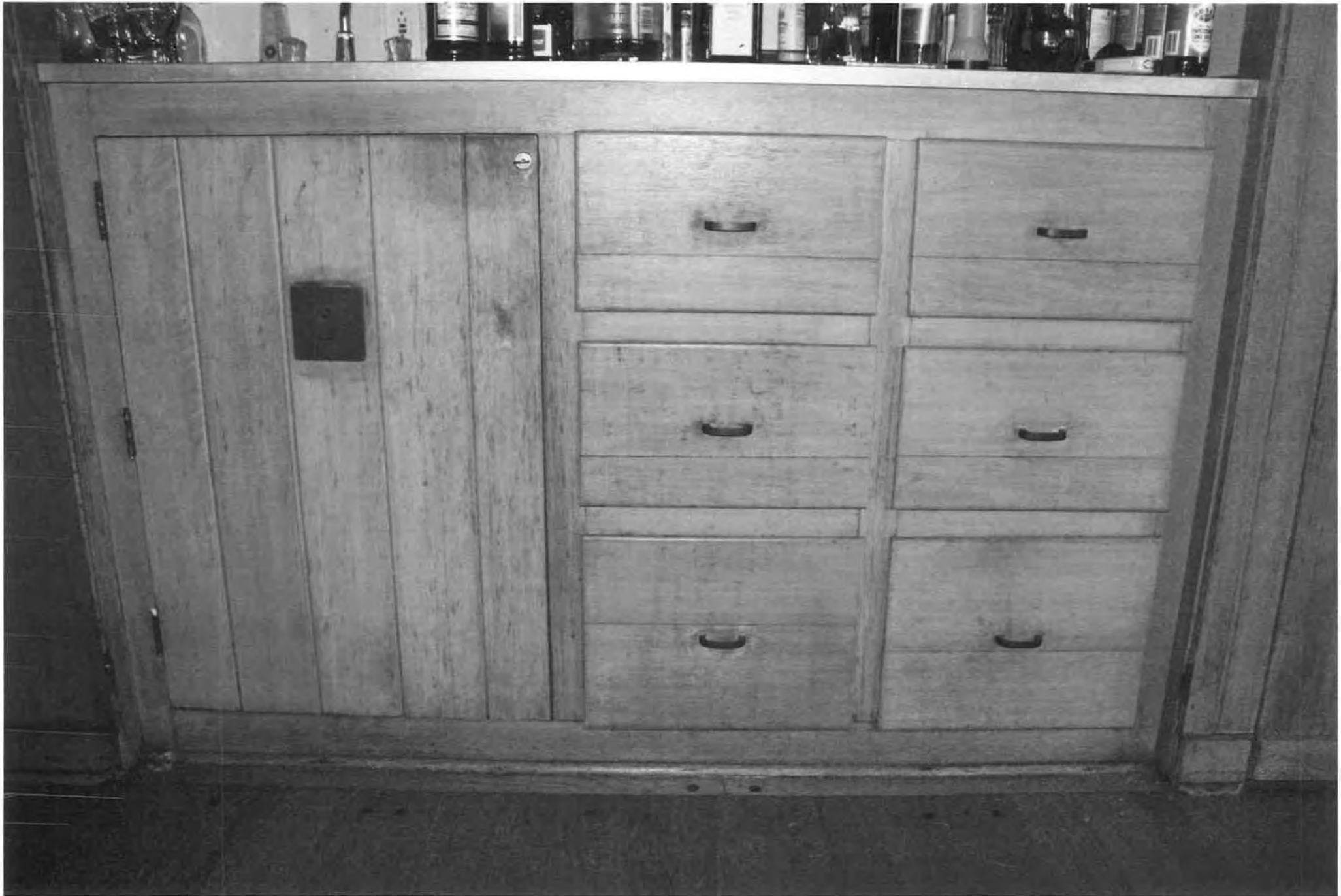
901Mt. Lebanon Road_New Castle County_DE First floor den, detail view of south wall showing wetbar, original built-ins and hardware
