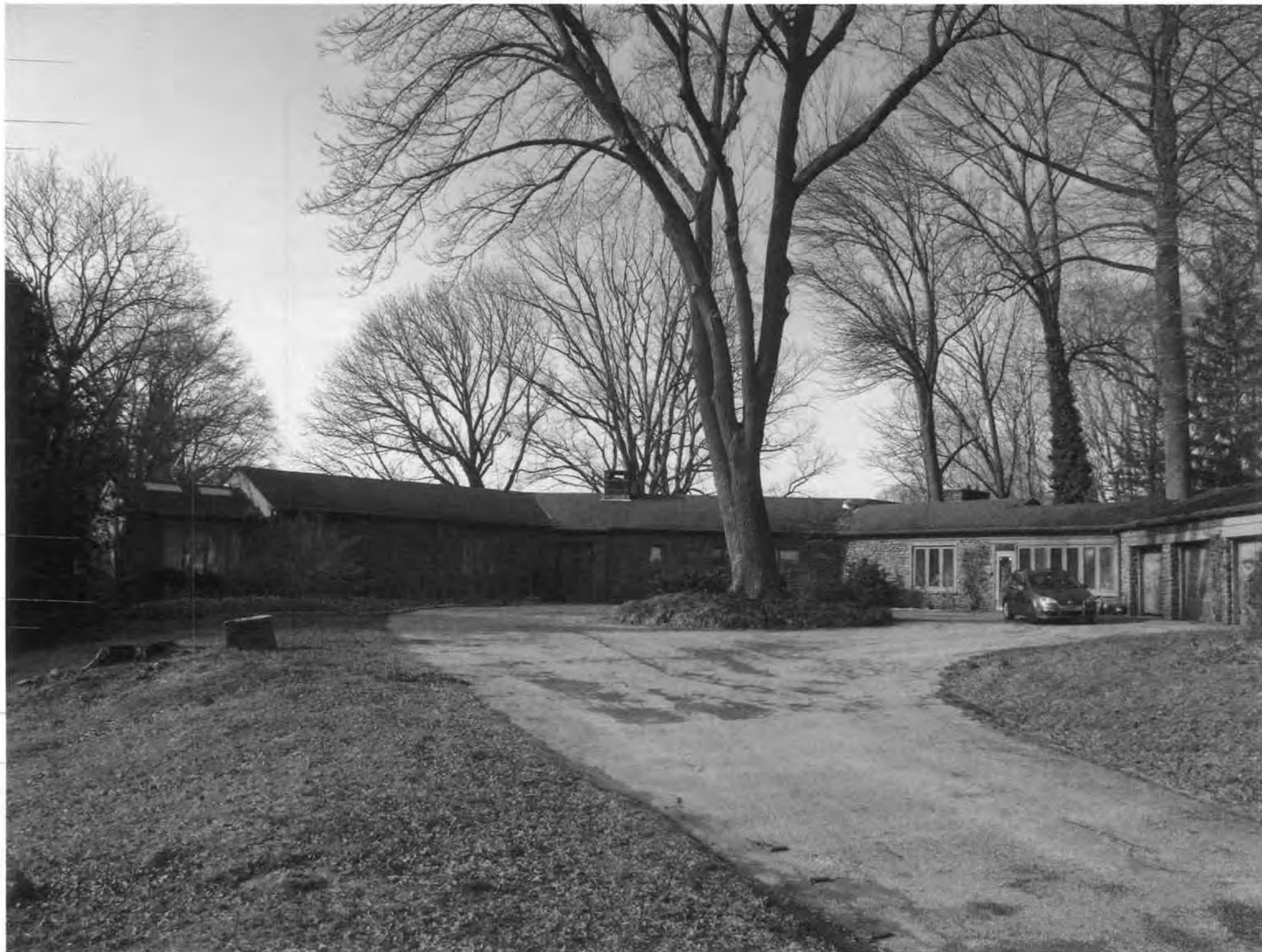
901 Mt. Lebanon Road_New Castle County_DE Perspective view of house on Mt. Lebanon Road side looking northwest (bedroom wing, living room, kitchen, garage, circle driveway) 03 of 39
