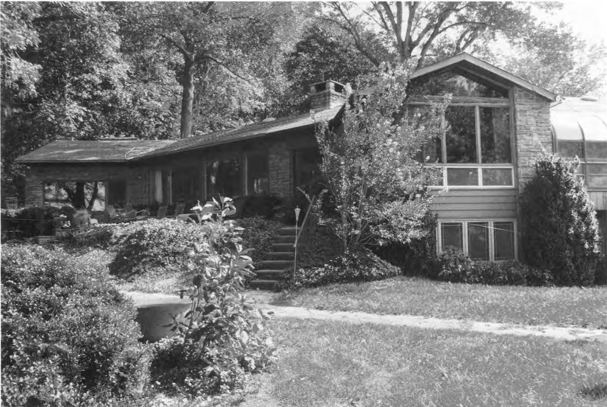
901 Mt. Lebanon Road_New Castle County_DE West elevation of den section, northwest elevation of living room section, rear patio area, and west elevation of rear office area looking east 13 of 39
