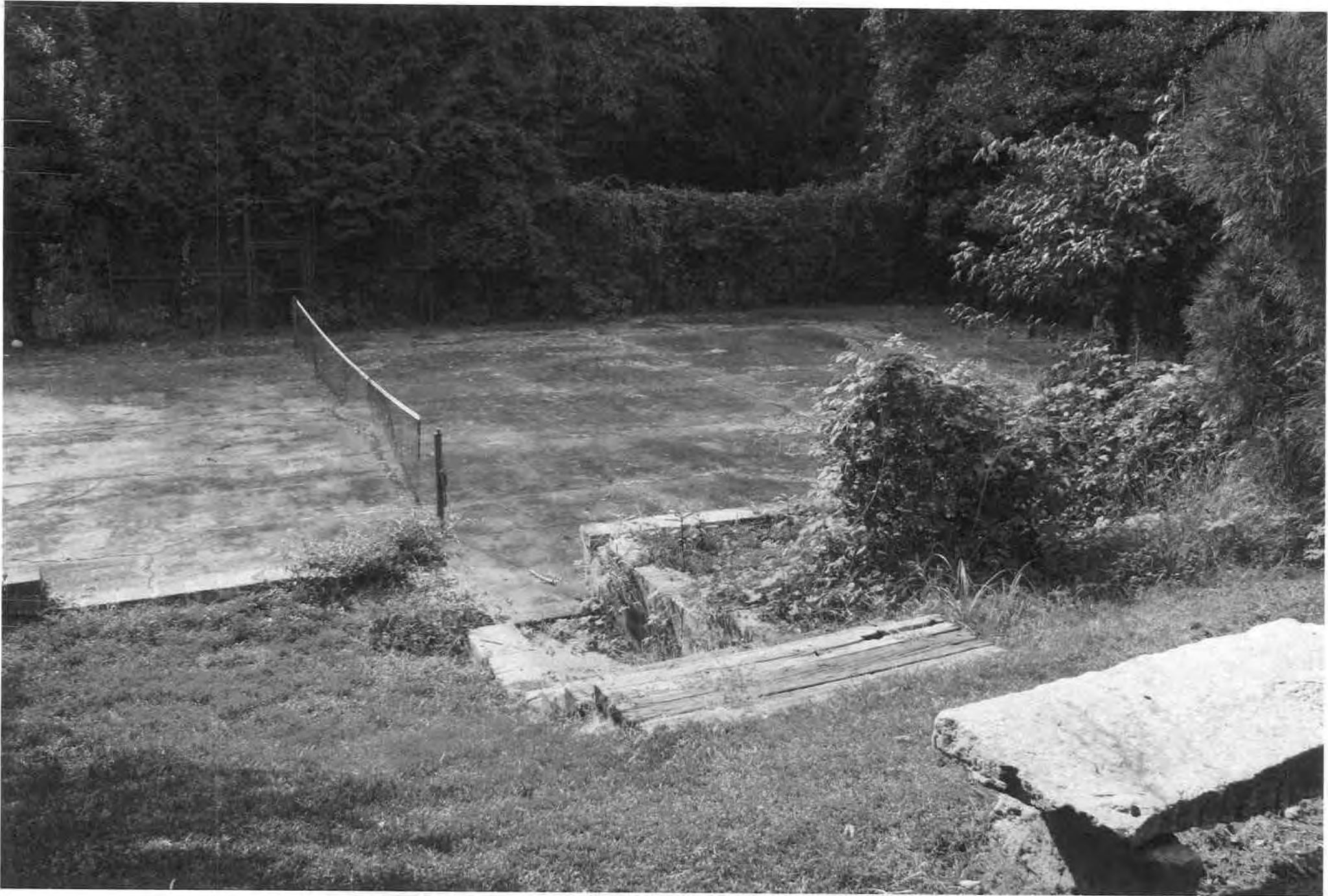
901 Mt. Lebanon Road_New Castle County_DE Tennis court at north corner of property looking south
