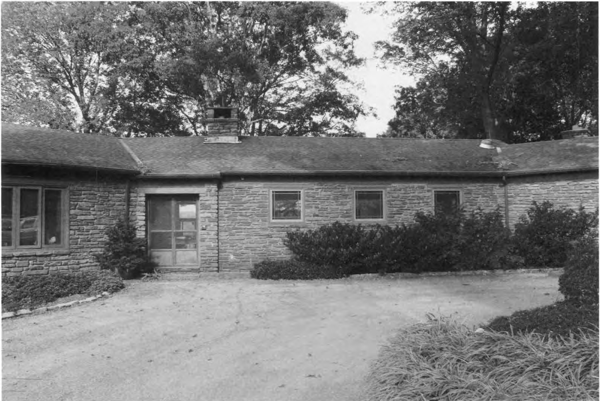
901 Mt. Lebanon Road_New Castle County_DE Southeast elevation of the central living room section with main entrance and circle driveway looking northwest
