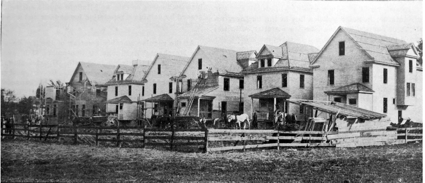
“New Houses in Course of Erection on West Delavan Ave.” (1902)
