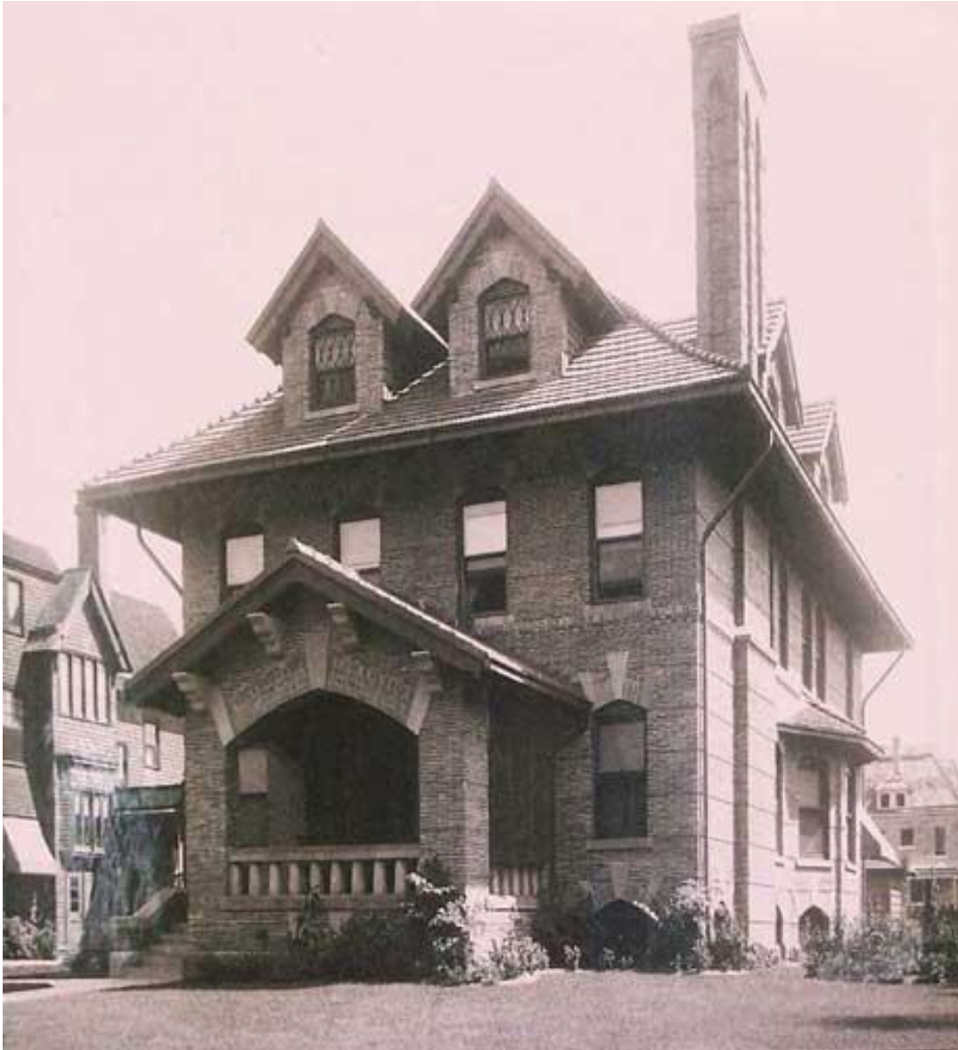
Edward H. Webster House, 781 West Ferry, ca. 1908
