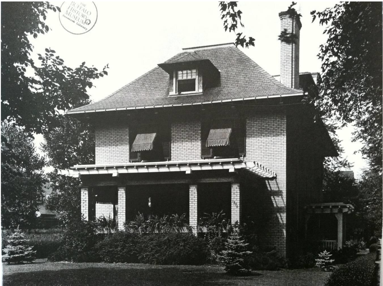
Emanuel Boasberg House, 1296 Delaware Avenue, ca. 1911
