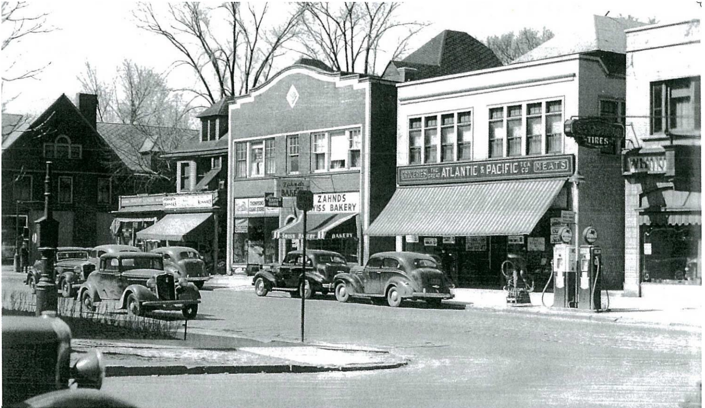
Elmwood Avenue looking south-west from Cleveland Avenue, by Willard T. Baldy (1940)
