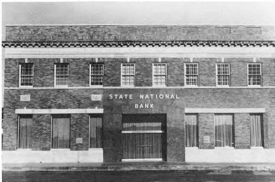
Figure -11 State National Bank after façade renovations, ca 1960. Photograph from Garland, Its Premiere Century .
