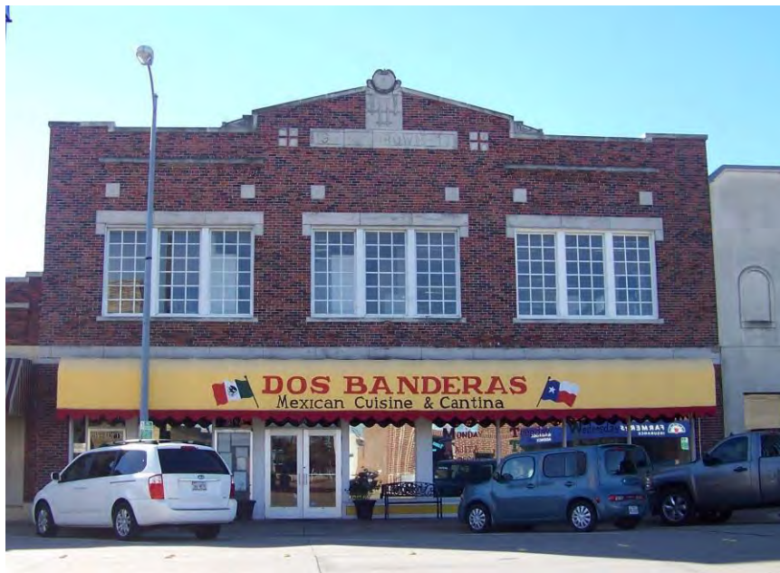
Photo – 16 View of C.M. Brown building, 614 Main Street, with three bays, each with three windows at the second floor with a stone header and sill. Note articulated parapet and decorative stone ornamentation above windows. Contributing building.
