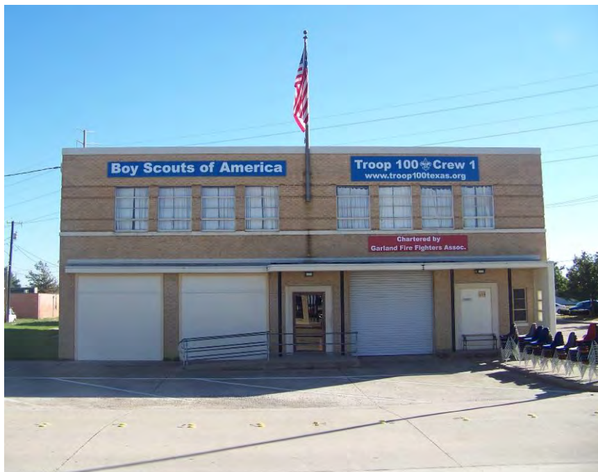
Photo – 24 View looking east at the former Garland Fire Department building at 116 South 6 th Street. Contributing building.
