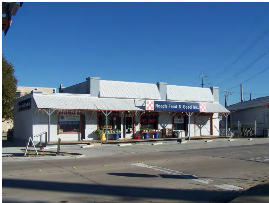
Photo – 19 View looking north on Main Street of Roach Feed and Seed at 409 Main Street. Contributing building.
