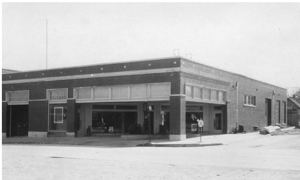
Figure -10 Morrison's Garage, constructed in 1920 to replace the earlier wood structure. Photograph courtesy Garland Landmark Society.
