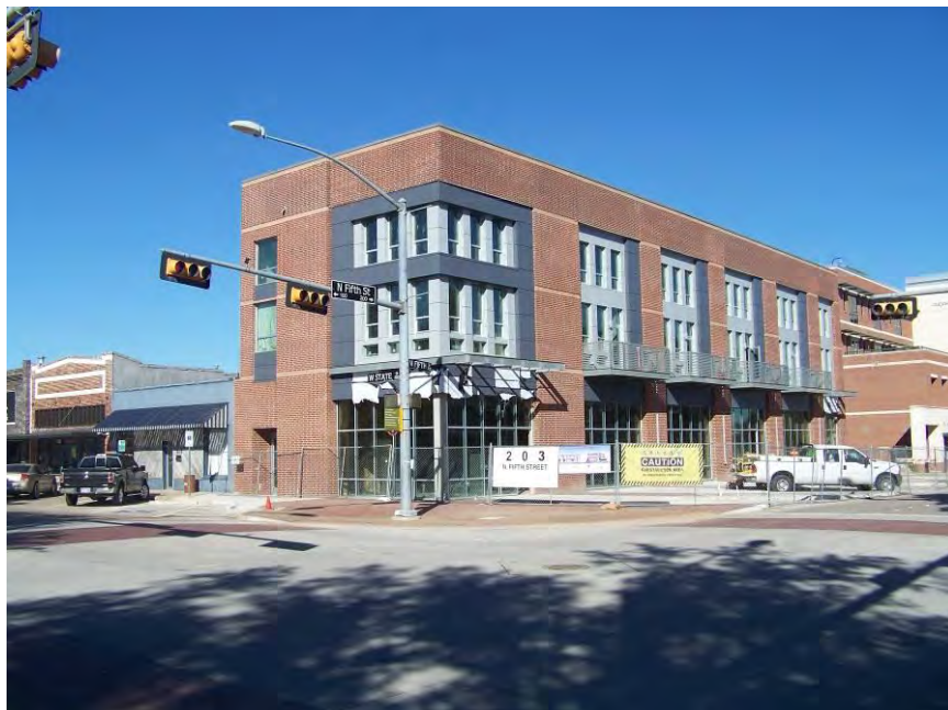
Photo – 10 View of 203 North 5 th Street, non-contributing multi-use building.
