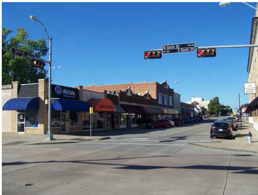
Photo – 3 View west on Main Street, photograph taken from intersection of Main and 6 th Streets. The two-story structure visible in the photograph is the C.M. Brown building.
