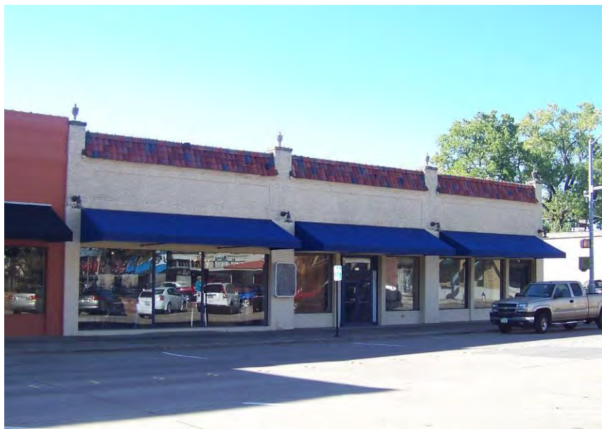
Photo – 17 View of 532 Main Street. Note the terra cotta tile and urns at the top of the parapet. These features were used on other prominent Garland buildings like the Williams Funeral Home and Garland High School. Contributing building.
