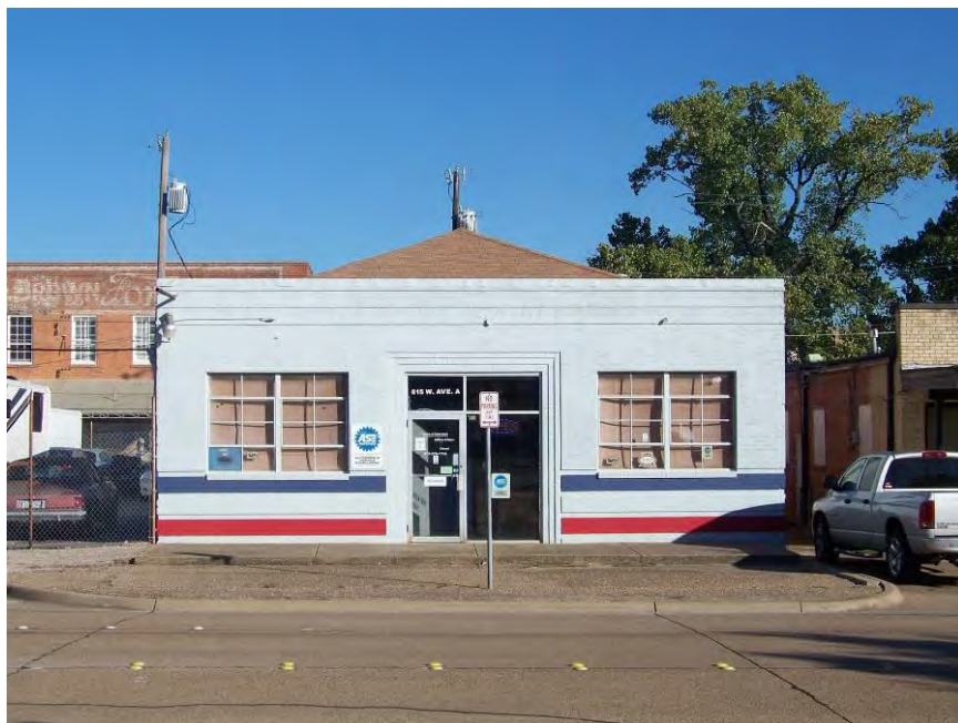
Photo – 26 View of 615 West Avenue A. Contributing building.
