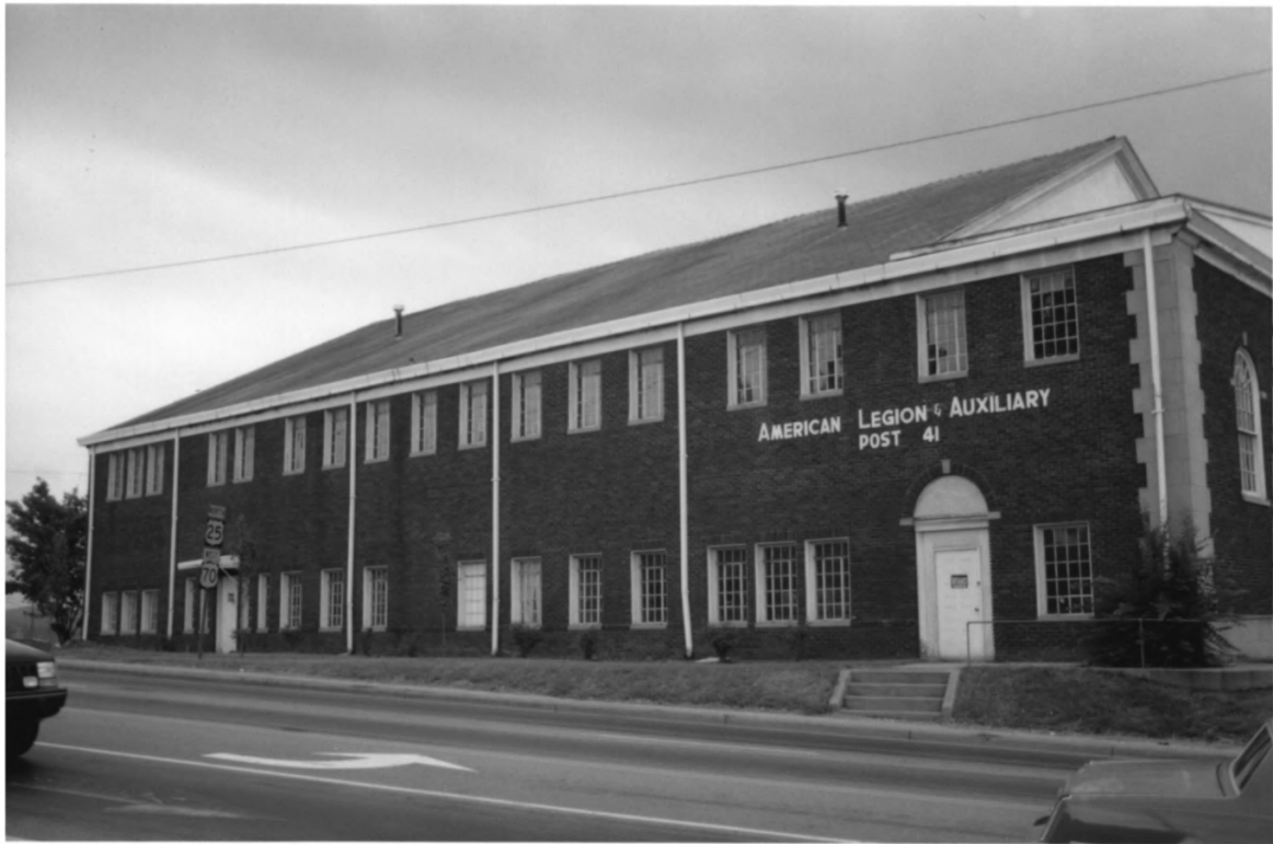
Cocke County Memorial Building Cocke Co., TN 3 of 22
