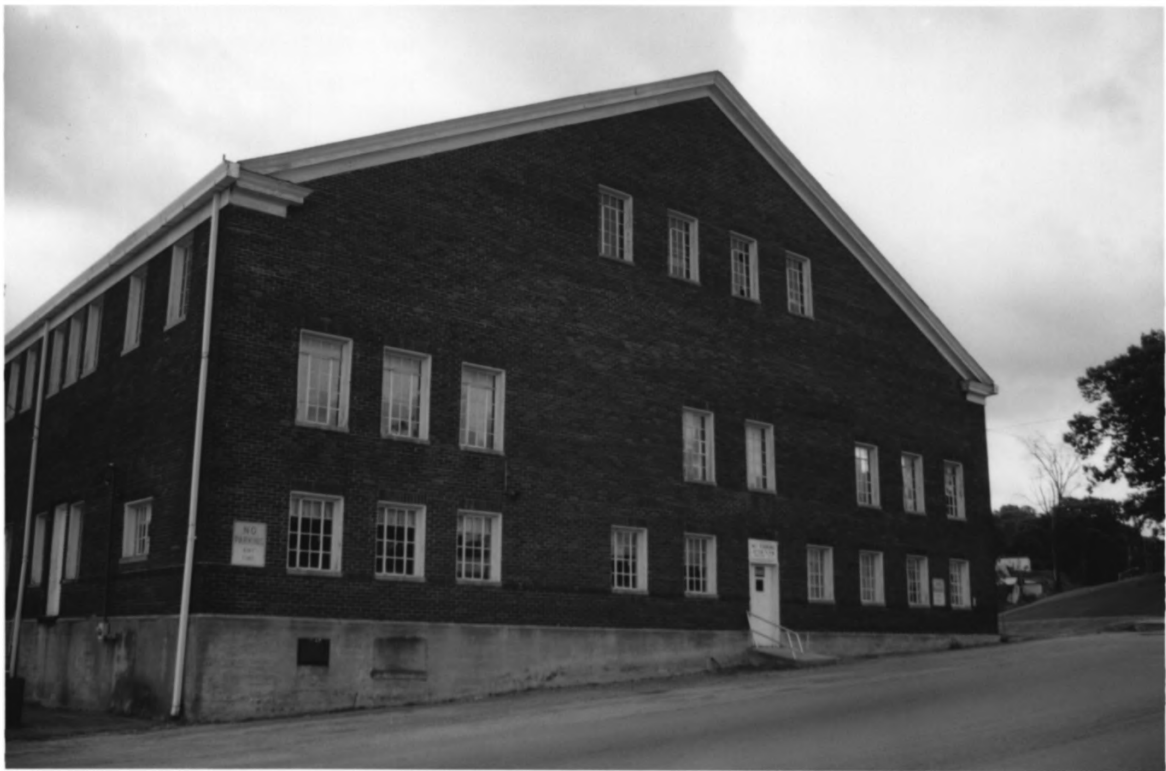
Cocke County Memorial Building Cocke Co., TN 4 of 22
