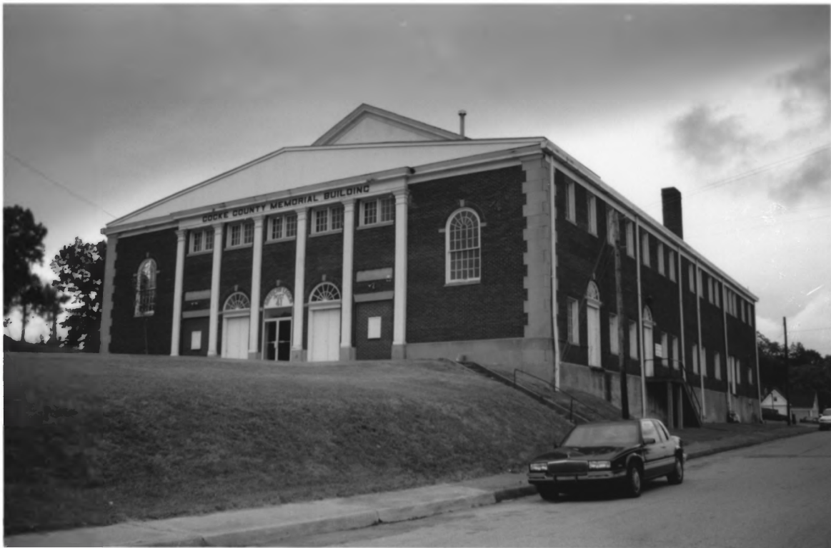
Cocke County Memorial Building Cocke Co., TN 1 of 22
