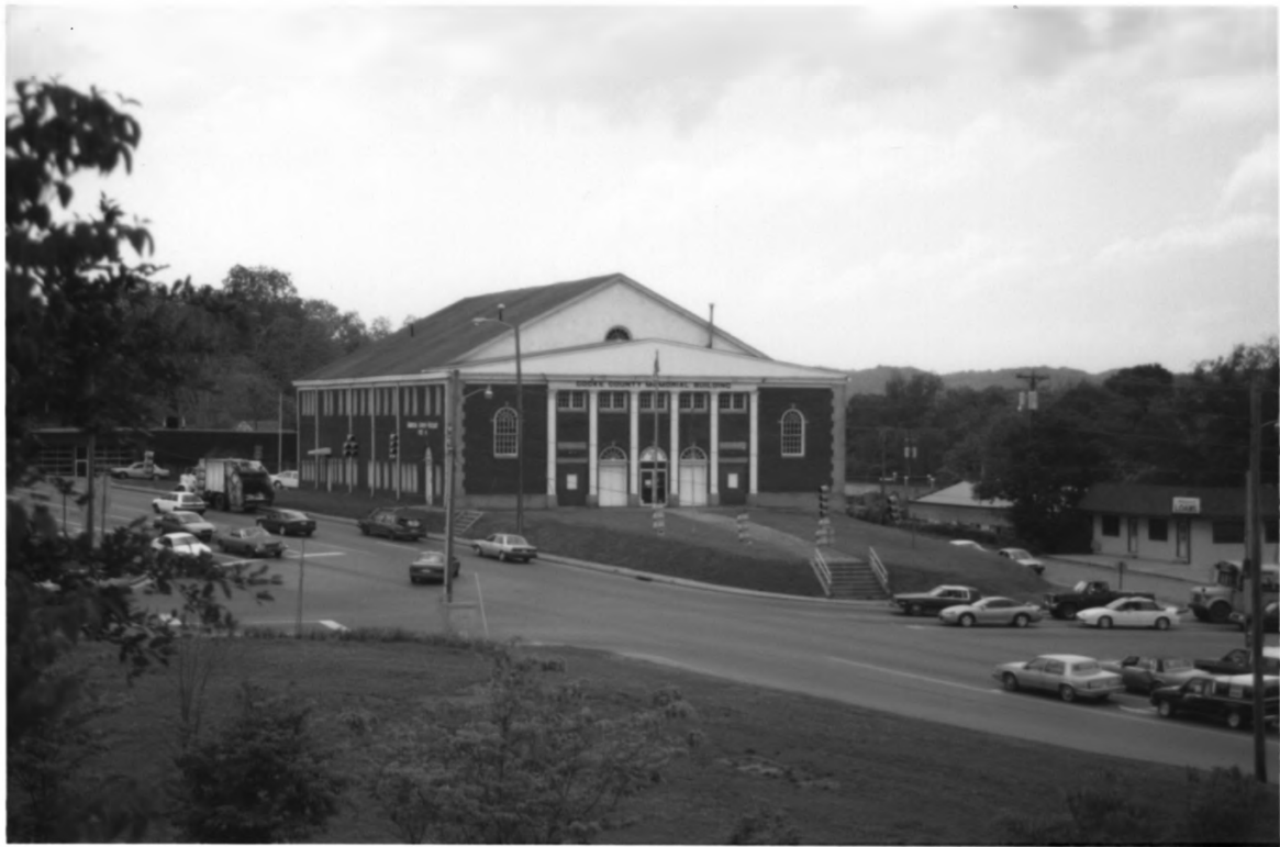
Cocke County Memorial Building Cocke Co., TN 2 of 22
