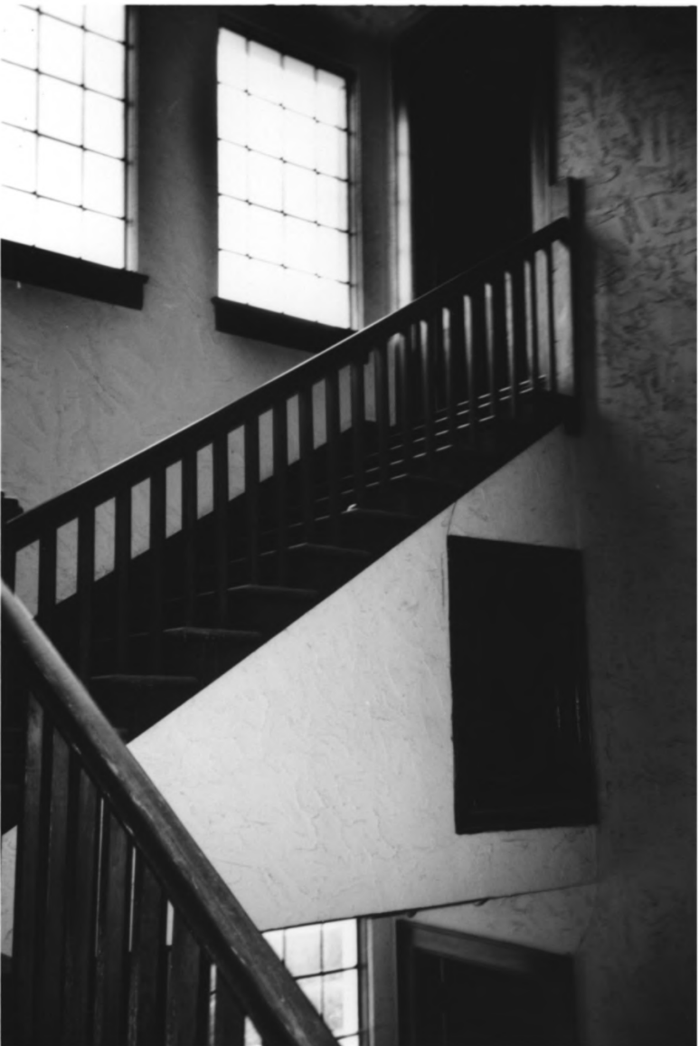
Cocke County Memorial Building Cocke Co., TN 19 of 22
