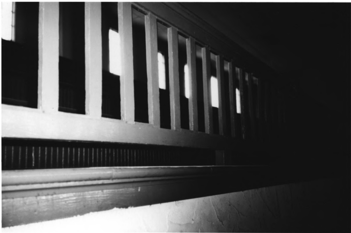
Cocke County Memorial Building Cocke Co., TN 13 of 22
