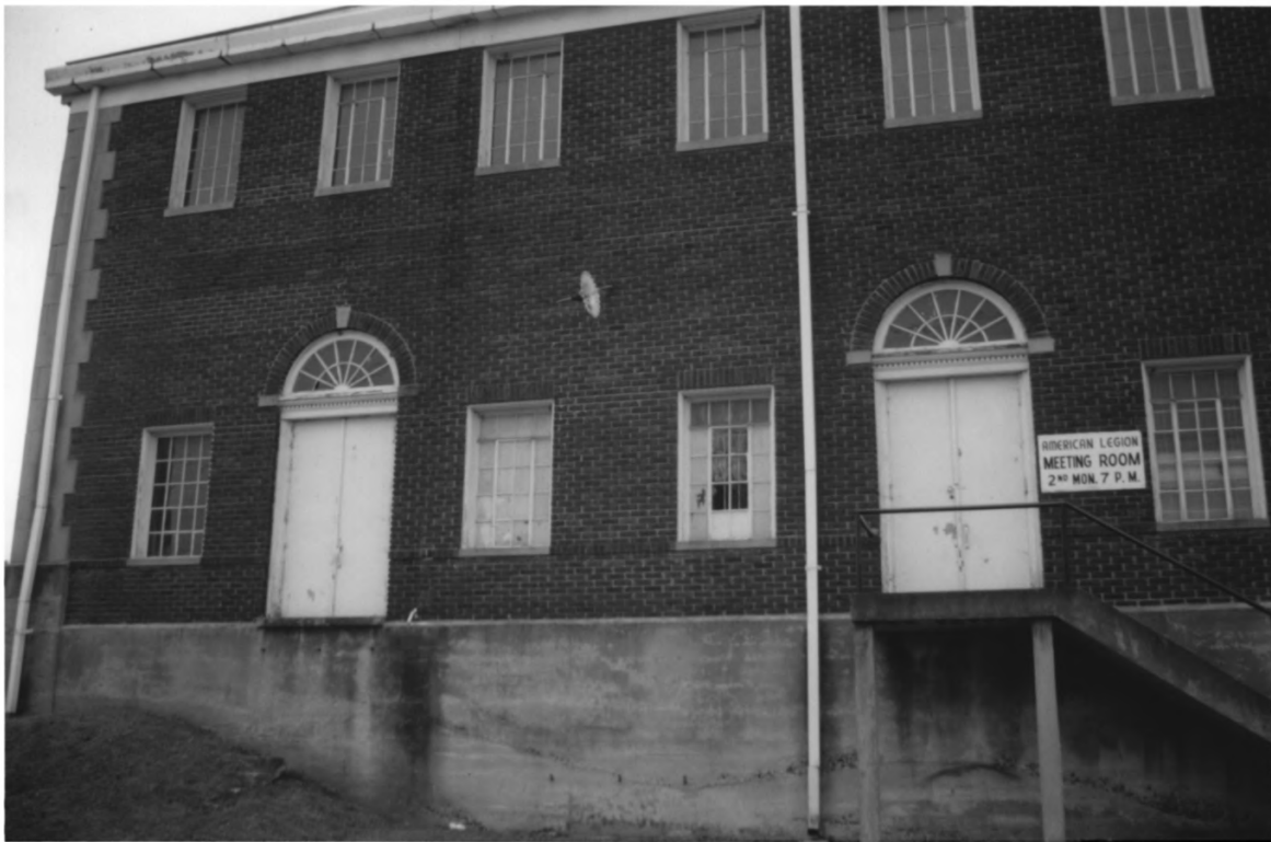
Cocke County Memorial Building Cocke Co., TN 8of22
