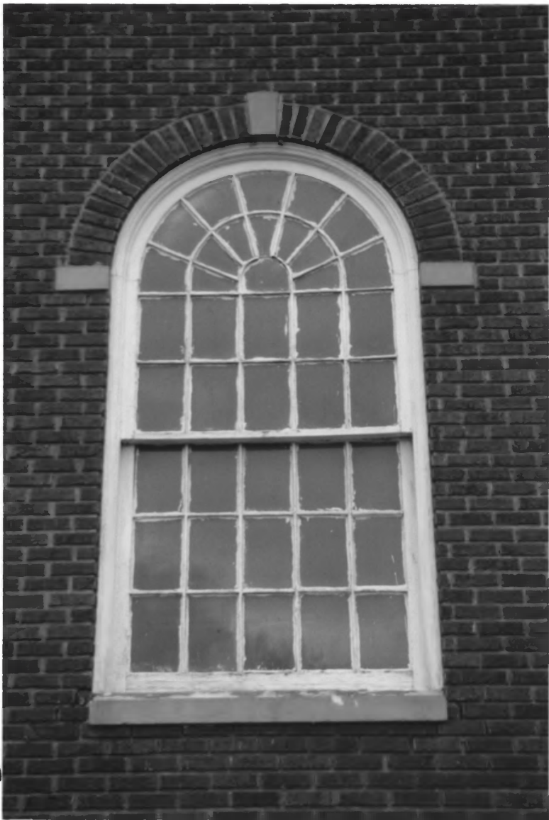
Cocke County Memorial Building Cocke Co., TN 7 of 22
