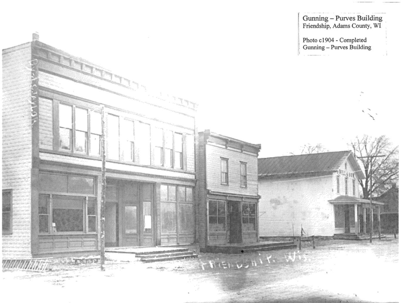
Figure 5: Historic Photograph, c1904
