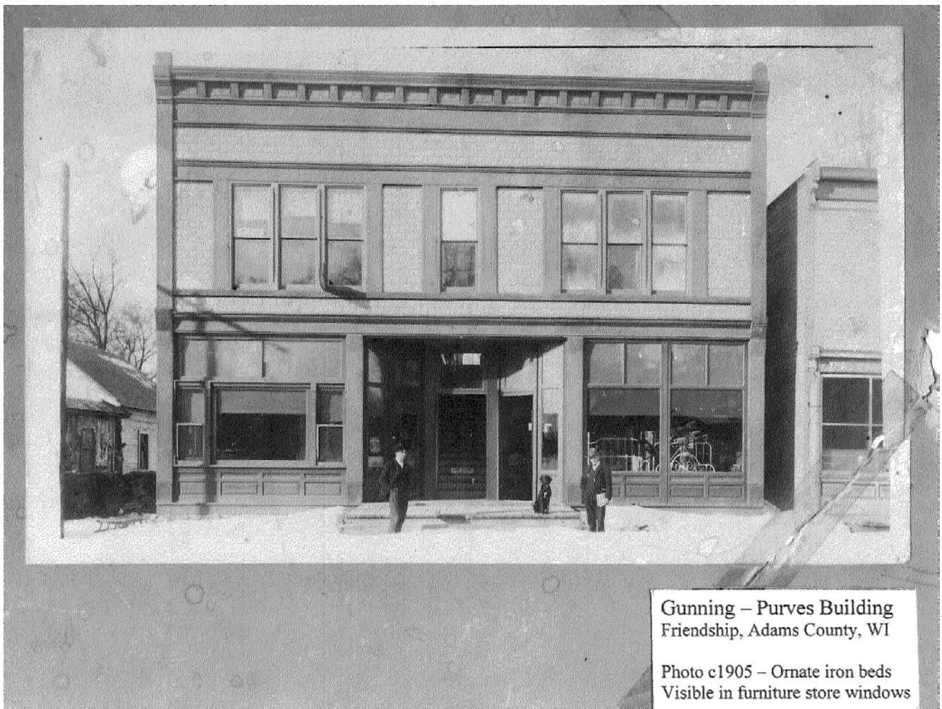
Figure 6: Historic Photograph c1905
