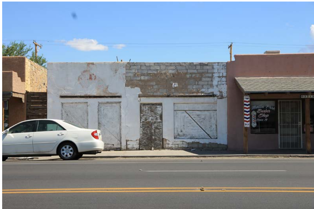
2 of 48. Commercial building at 3211 Main Street, photographer facing northeast.
