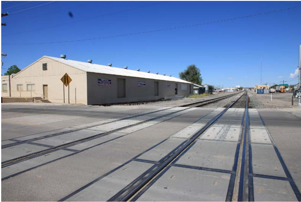
13 of 48. Warehouse, 3301 Harrelson Street, photographer facing northwest.
