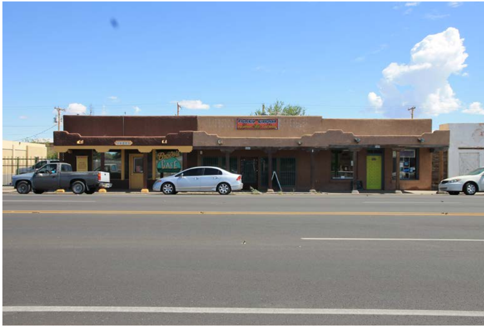
3 of 48. Commercial buildings at 3205 to 3209 Main Street, photographer facing northeast.
