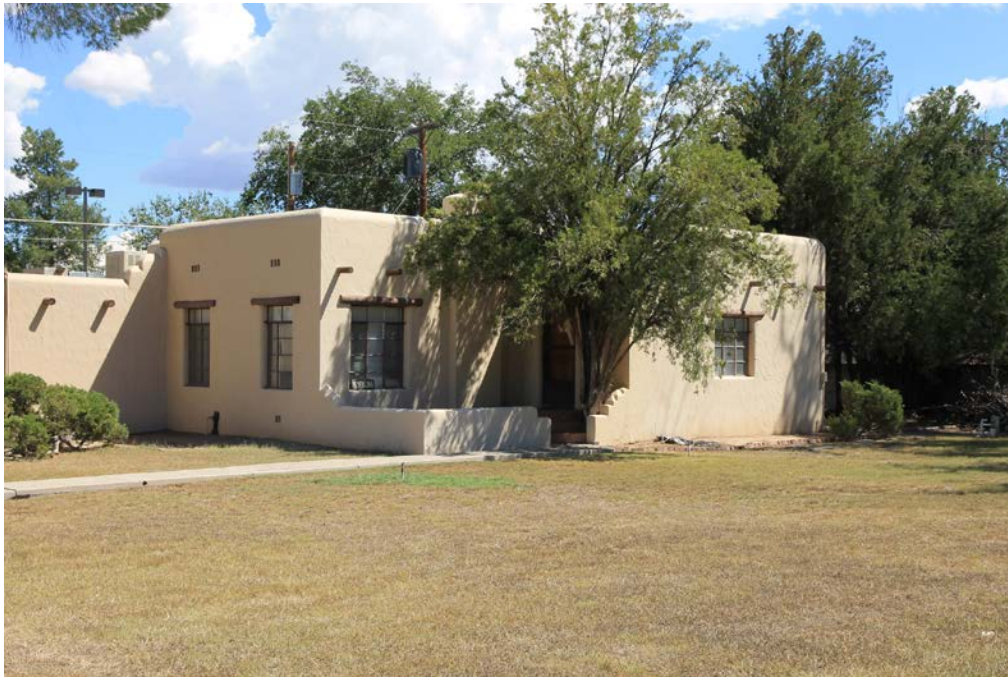
41 of 48. 3301 Bowman Street, photographer facing east.
