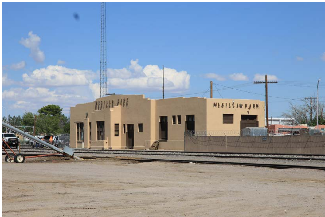
12 of 48. Mesilla Park railroad depot, photographer facing north.
