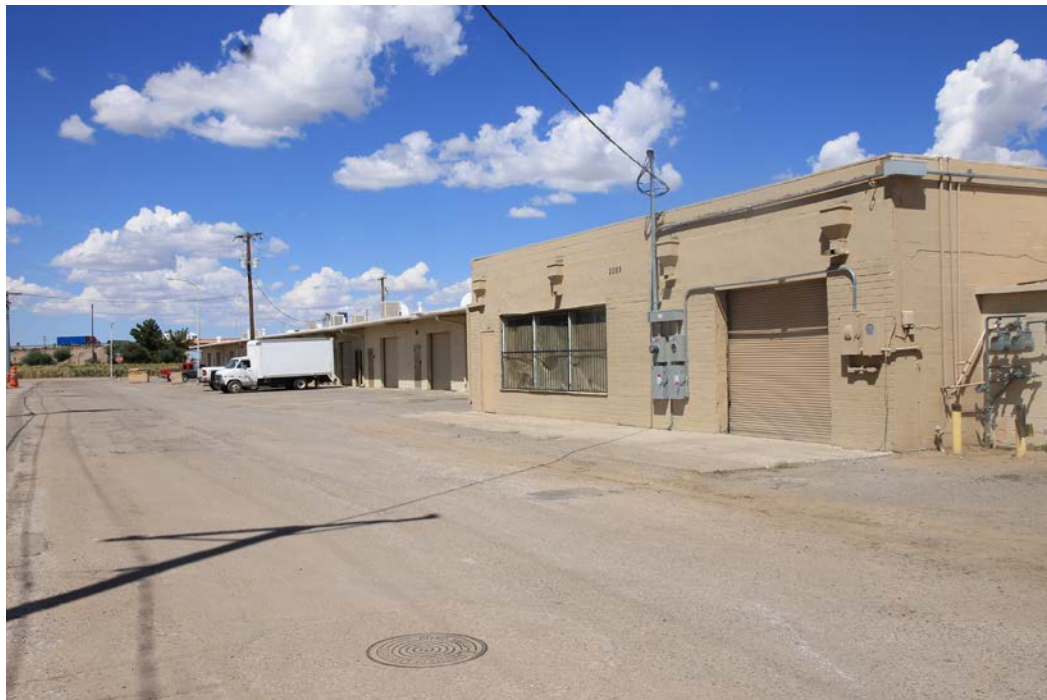
18 of 48. Warehouse at 3055 to 3001 Harrelson Street, photographer facing north.
