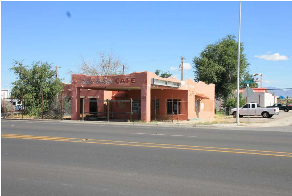
5 of 48. Commercial building at 3111 Main Street, photographer facing northeast.
