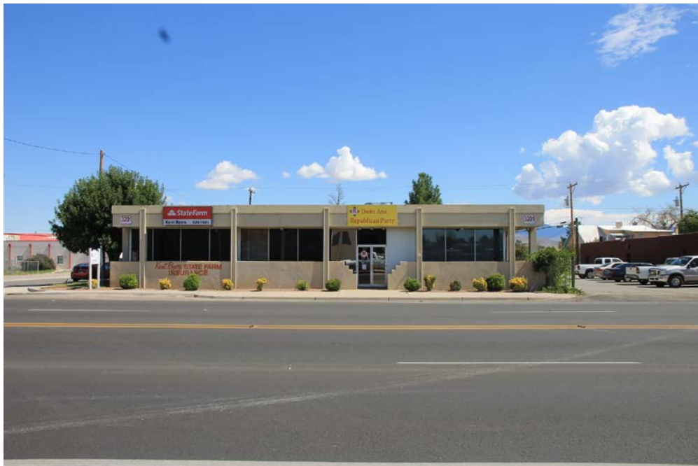
4 of 48. Commercial building at 3201 Main Street, photographer facing northeast.
