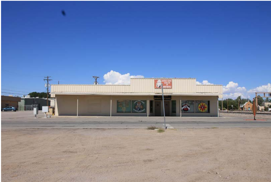
17 of 48. Commercial Building at 102 Conway Avenue, photographer facing northwest.
