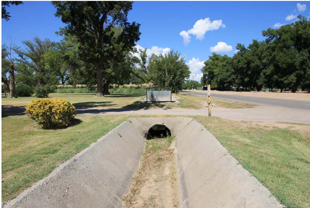
21 of 48. Paved ditch, Bowman Street, photographer facing northwest.
