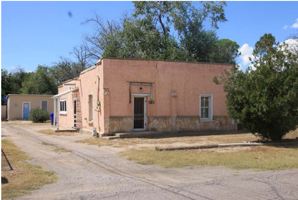
33 of 48. 3104 Linden Avenue, photographer facing southwest.
