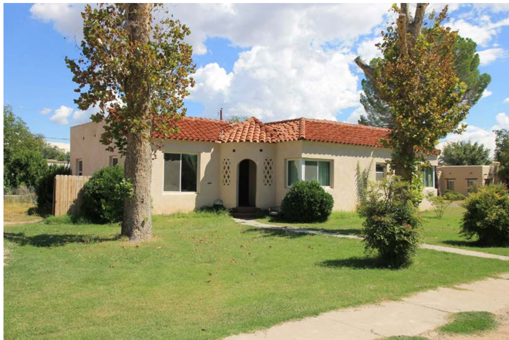
40 of 48. 3207 Bowman Street, photographer facing east.
