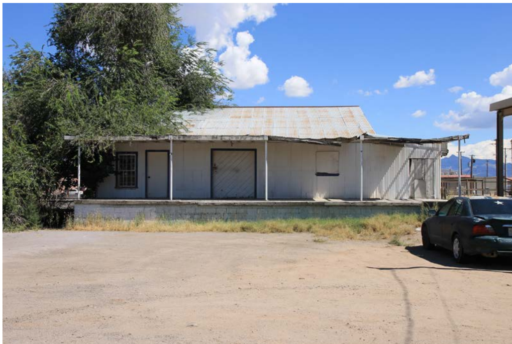
14 of 48. Warehouse, 3301 Harrelson Street, photographer facing east.
