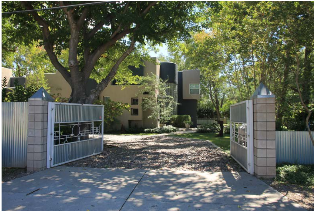
23 of 48. 3101 Bowman Street, photographer facing east.
