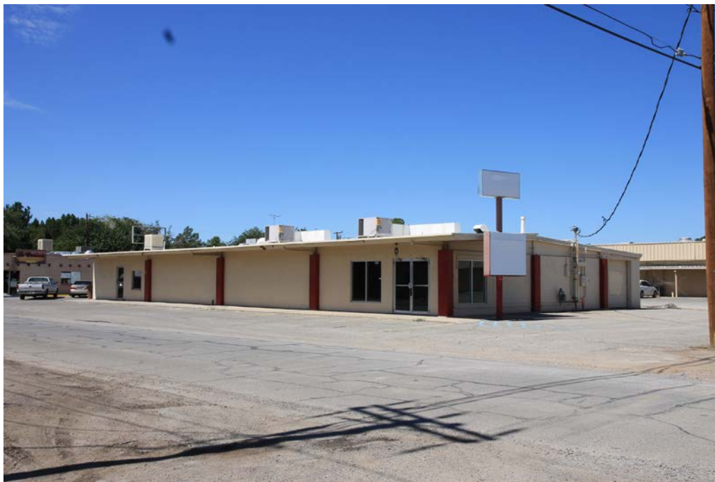
16 of 48. Commercial Building at 200 Conway Avenue, photographer facing west.
