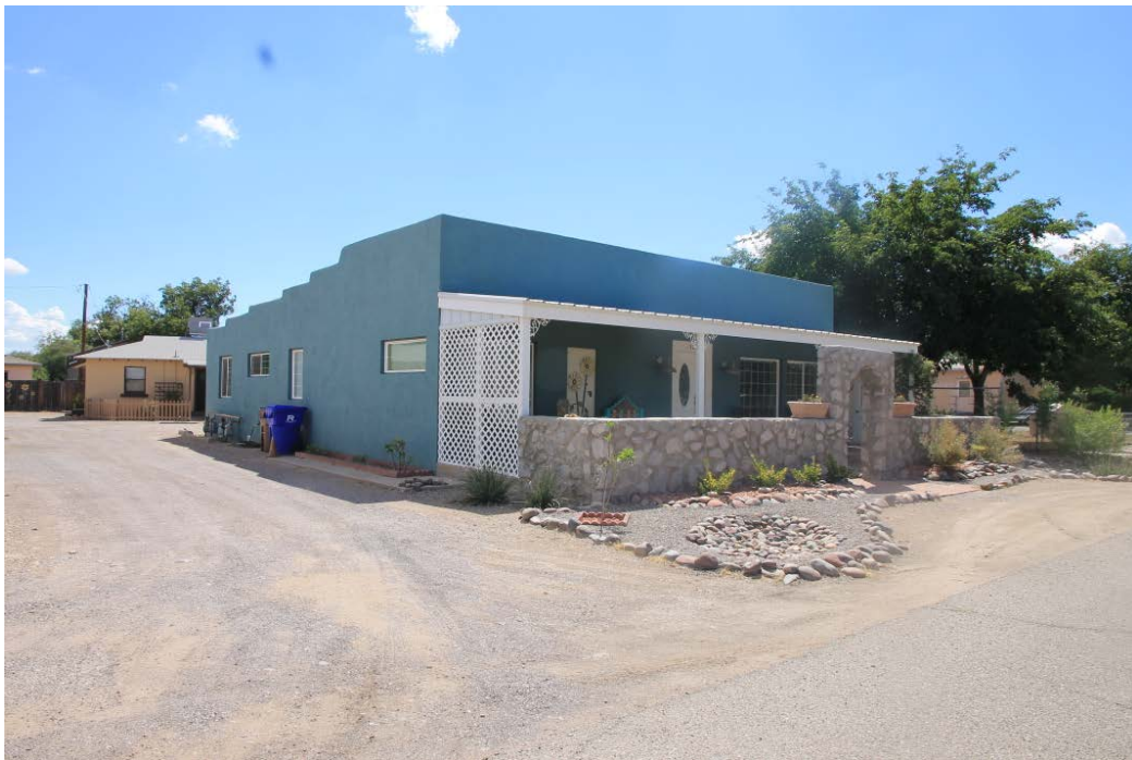
44 of 48. 321 Bell Avenue, photographer facing south.
