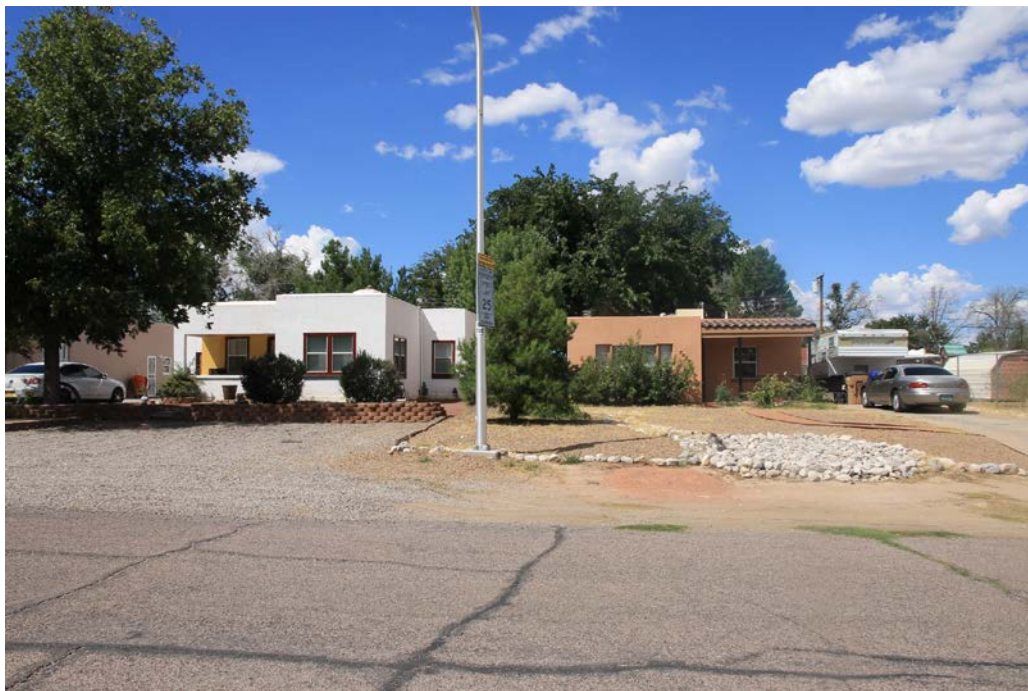
36 of 48. 400 and 390 Manso Avenue, photographer facing northwest.
